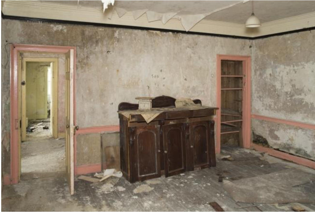
South Block, ground floor, dining room (0.18), view from east (RCAHMS: DP 194644)
