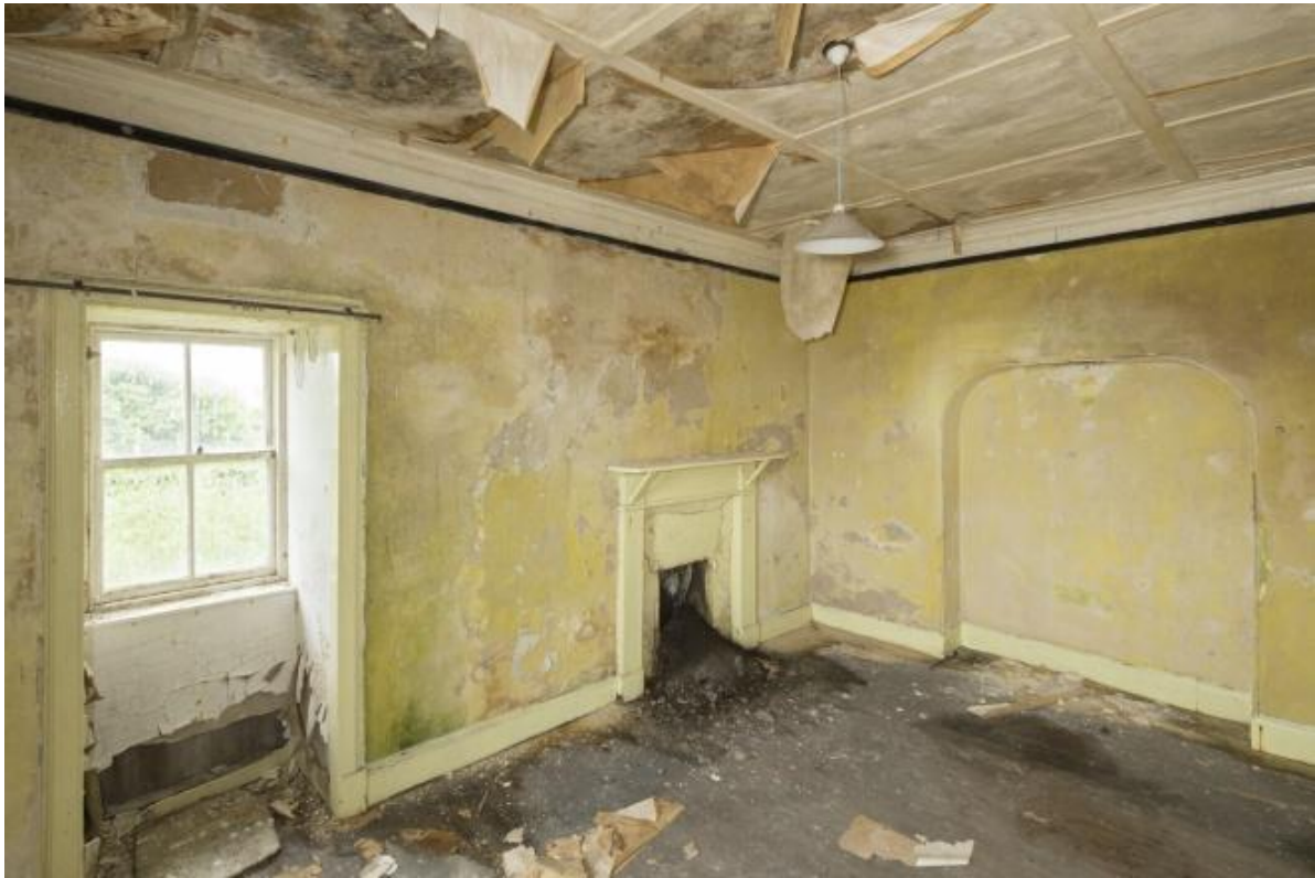
South Block, ground floor, parlour (0.12), view from east (RCAHMS: DP 194639)
