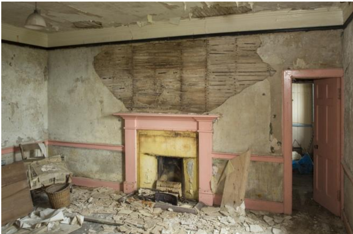
South Block, ground floor, dining room (0.18), view from south (RCAHMS: DP 194642)
