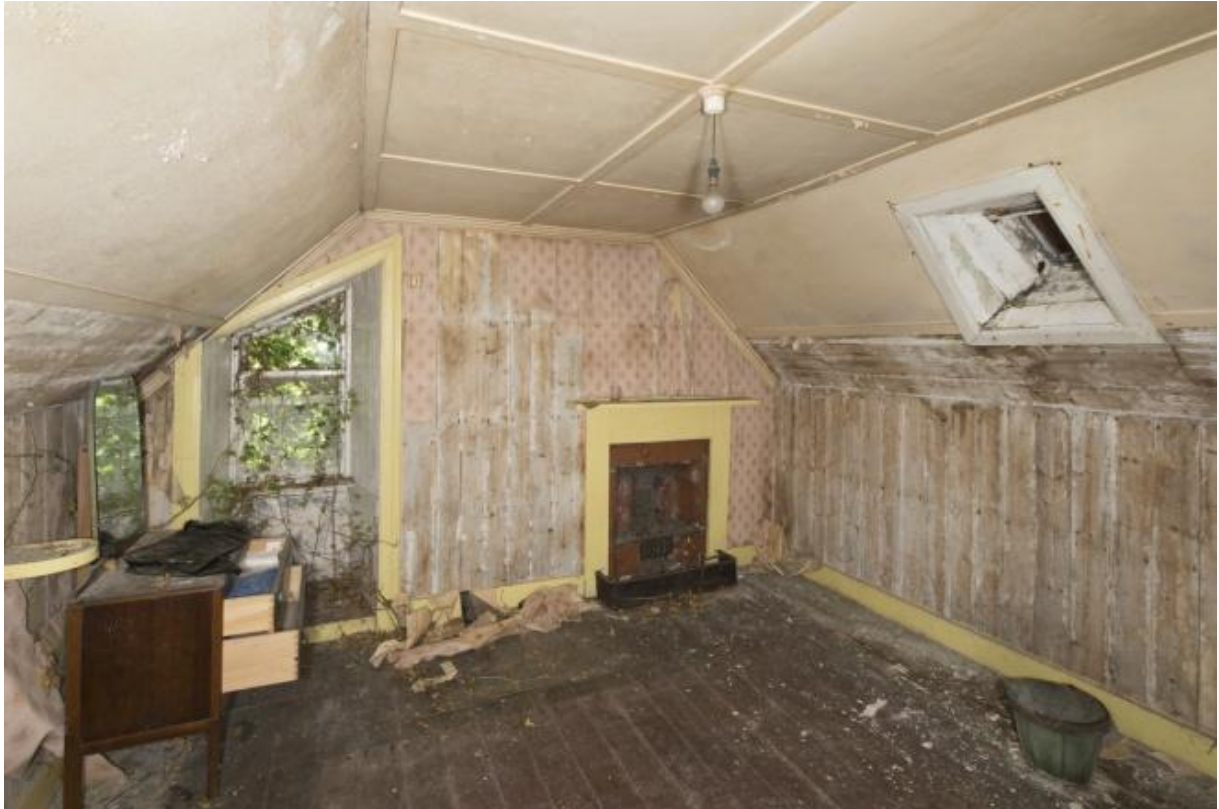
North Block, first floor, south bedroom (1.1), view from east (RCAHMS: DP194668)
