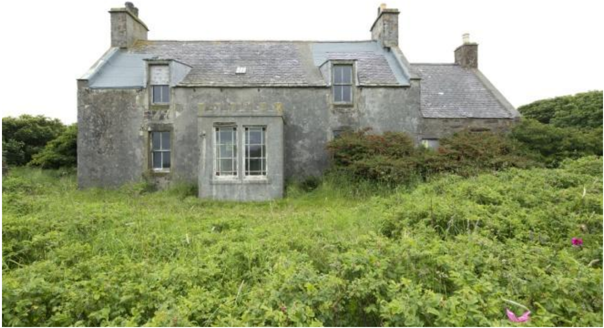
South range, main block, view from south east (RCAHMS: DP 194614)
