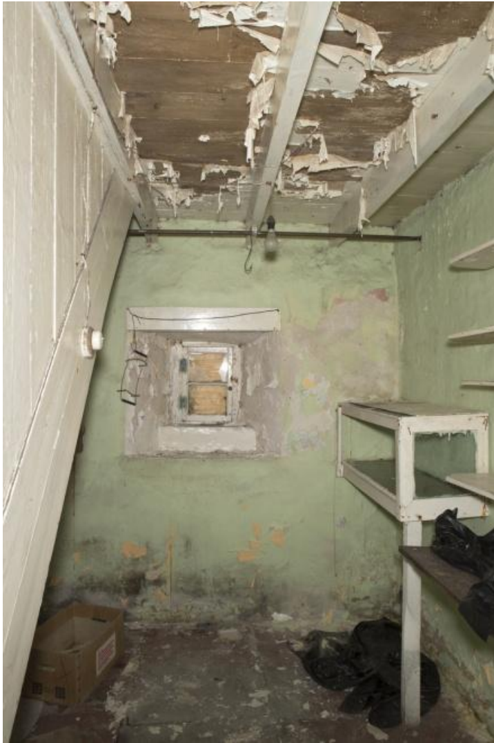
North Block, ground floor, pantry (0.4), view from south east (RCAHMS: DP 194662)
