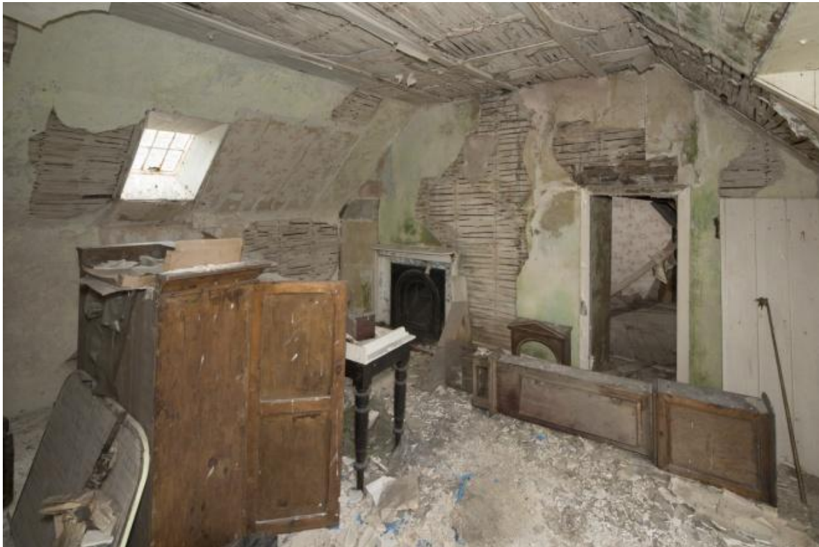
South Block, first floor, north bedroom (1.8), view from south (RCAHMS: DP 194656)
