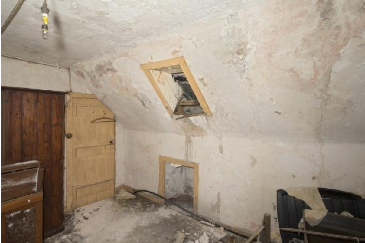
North Block, first floor, north bedroom (1.4), view from east showing blocked window at floor level (RCAHMS: DP194670)
