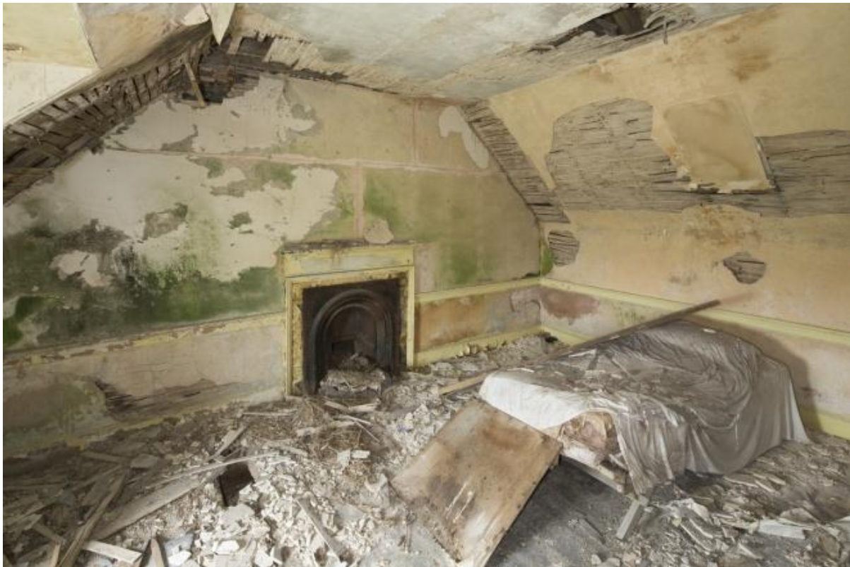
South Block, first floor, south bedroom (1.5), view from east (RCAHMS: DP 194653)
