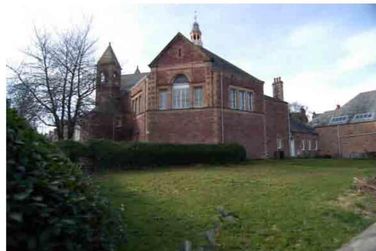
Fig. 7 North-east facing elevation of Braid Church
