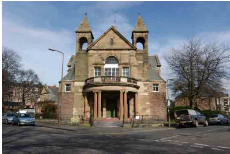
Fig. 3 South-west-facing elevation of Braid Church
