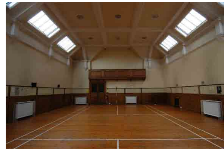
Fig. 15 Small hall showing the beams and ceiling configuration
