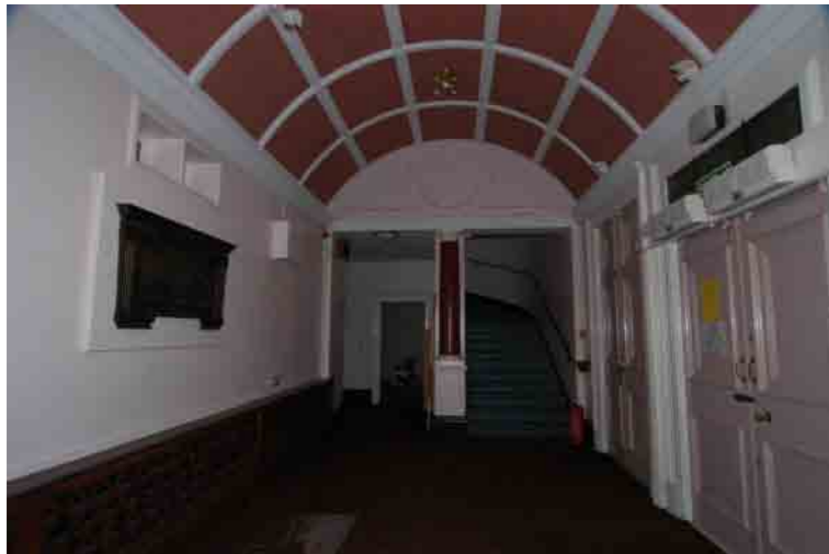
Fig. 9 Church vestibule with painted vaulted ceiling
