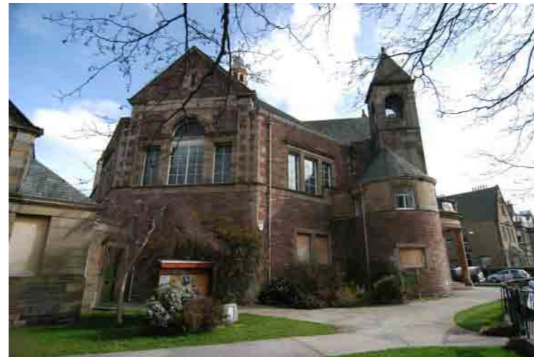
Fig. 4 Snecked-built sandstone stair turret, south-east elevation
