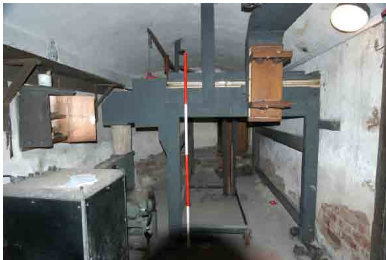
Fig. 17 Interior view of the basement organ pump room with vaulted ceiling
