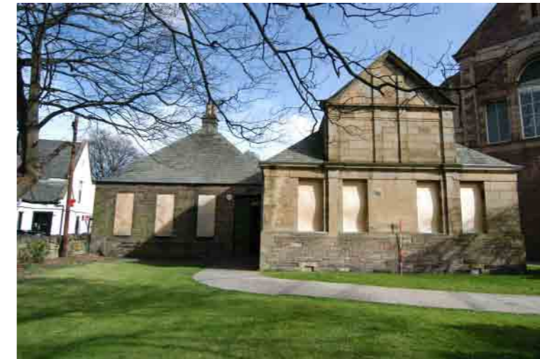
Fig. 5 South-west facing elevation of the Small Hall
