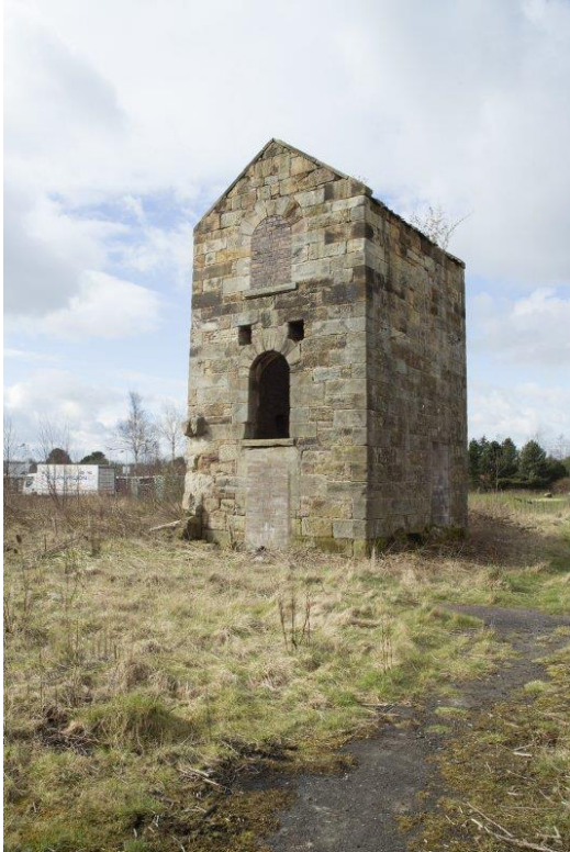
View of east gable showing the windows (frames and glazing gone) and the east doorway (blocked) at ground level. This doorway may have originally been a window feature. [DP231993, HES]
