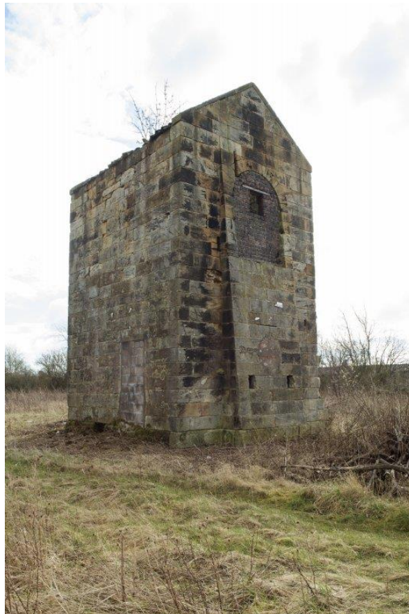
View from north west [DP 231994, HES]
