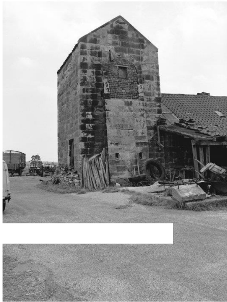
Left: View of Pump Engine House from west, showing the now demolished south range (right). Some of the now demolished buildings may have been part of the colliery. The low footings visible in front of the west wall is the backfilled shaft down which the pump rods of the engine ran. Men may also have used the shaft to get out of the mine workings at the end of their shift. [SC 454959, 1974, John R Hume Collection, National Record of the Historic Environment]
