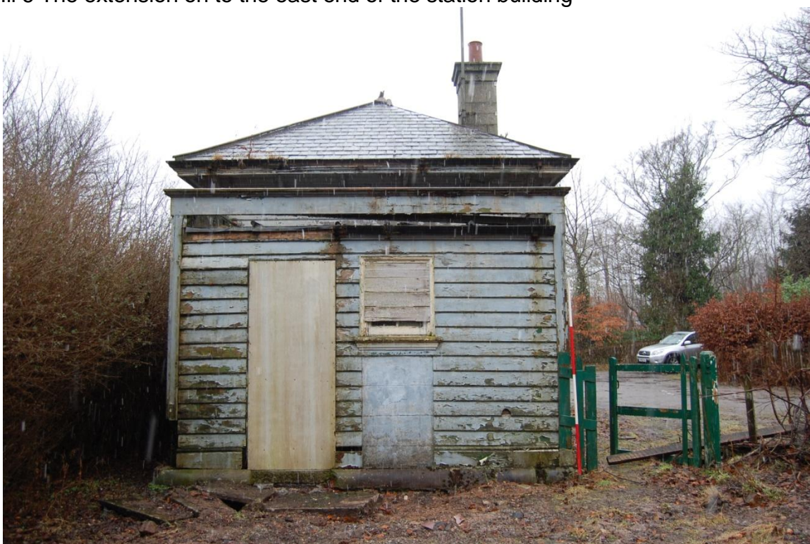
III 7 The extension on to the east end of the station building
