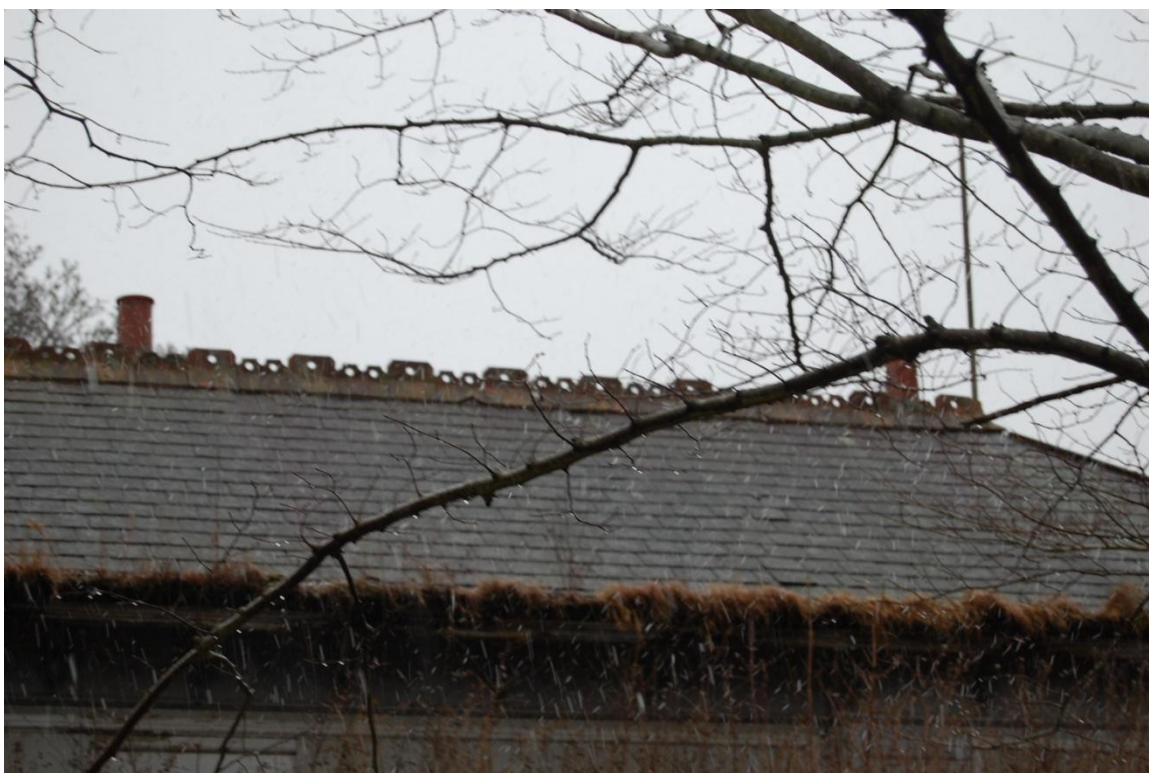
Ill 8 The terracotta ridge tiles
