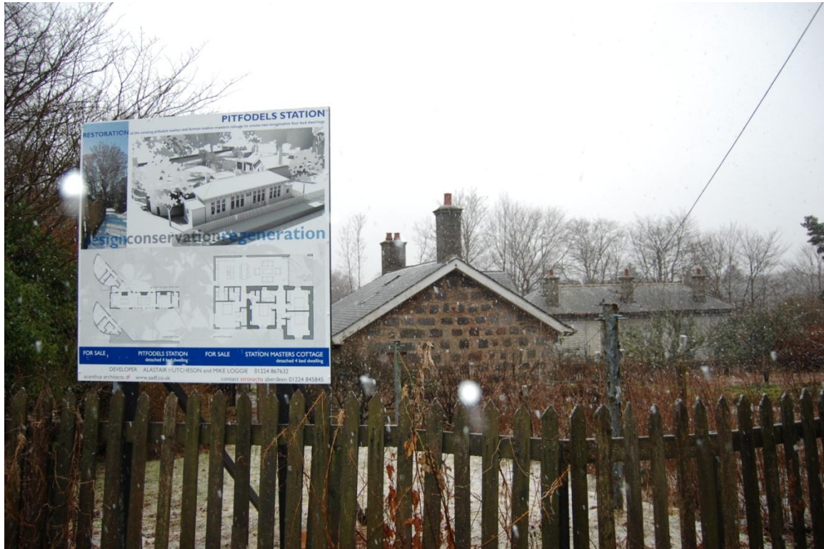
Ill 2 Station Building (right) and cottage (left) from the north
