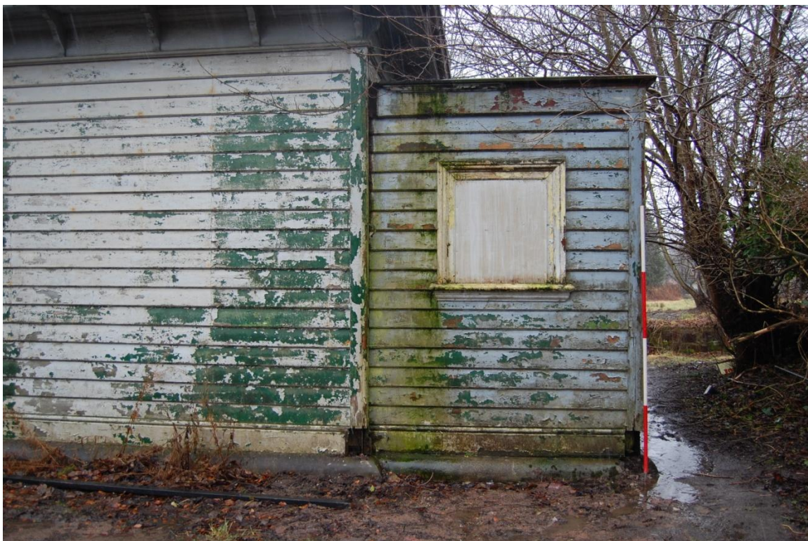
III 5 The extension to the west end of the station building
