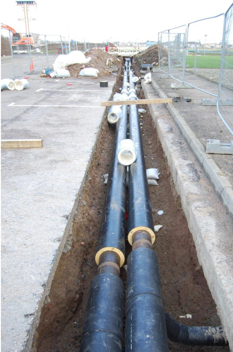
III 3 Trench excavated through Seaton Pottery site
