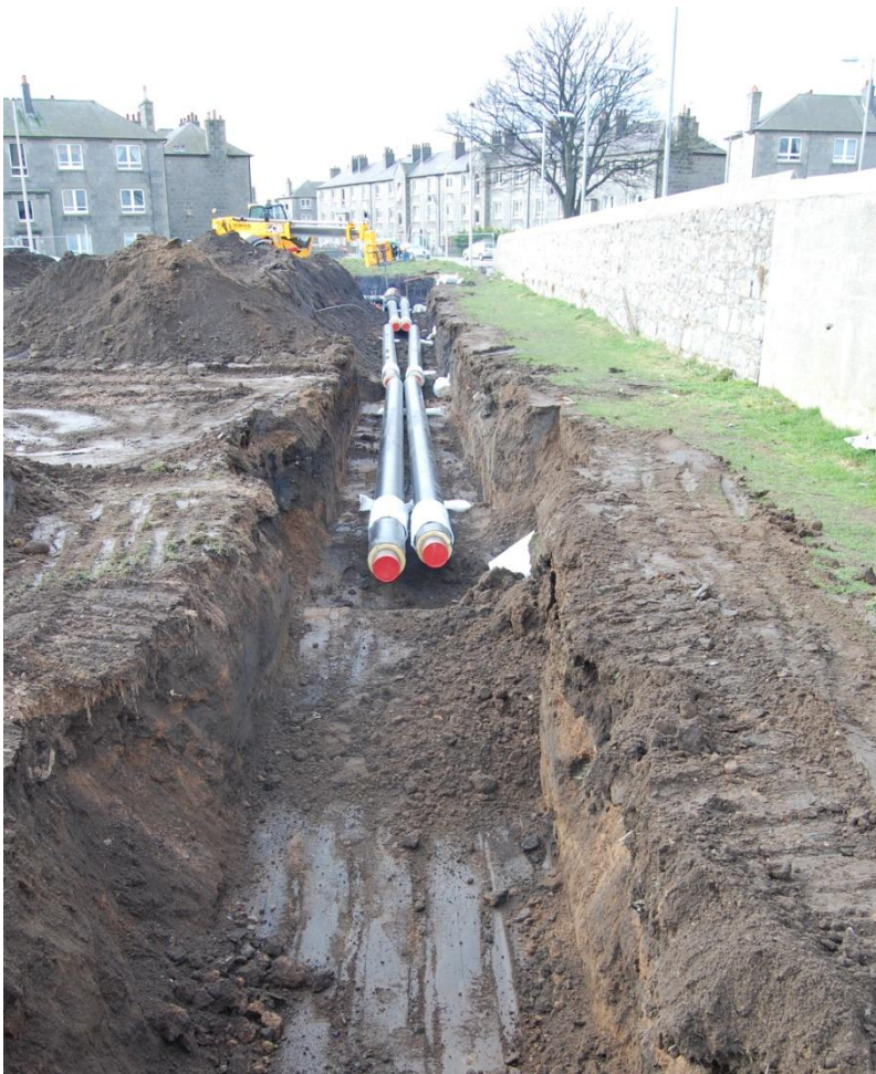
Ill 5 Trench 2 with Seaton School wall (right)
