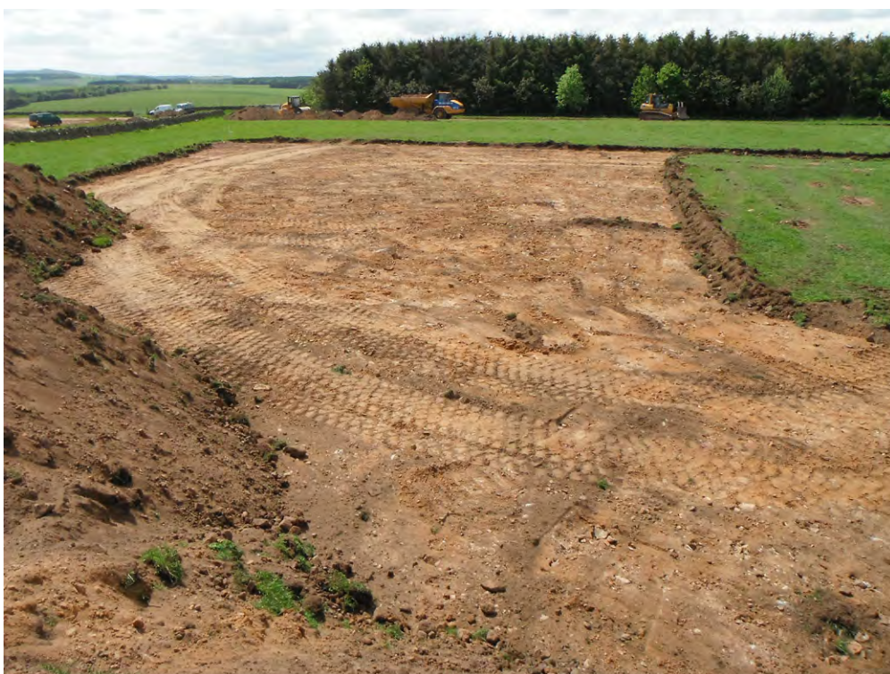
Fig. 9 Soil stripping within Site 16
