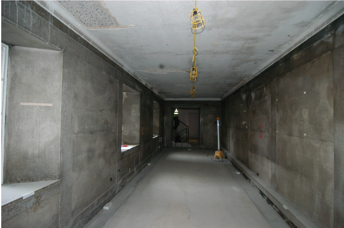
Fig. 10 Interior of the Link Bridge facing north
