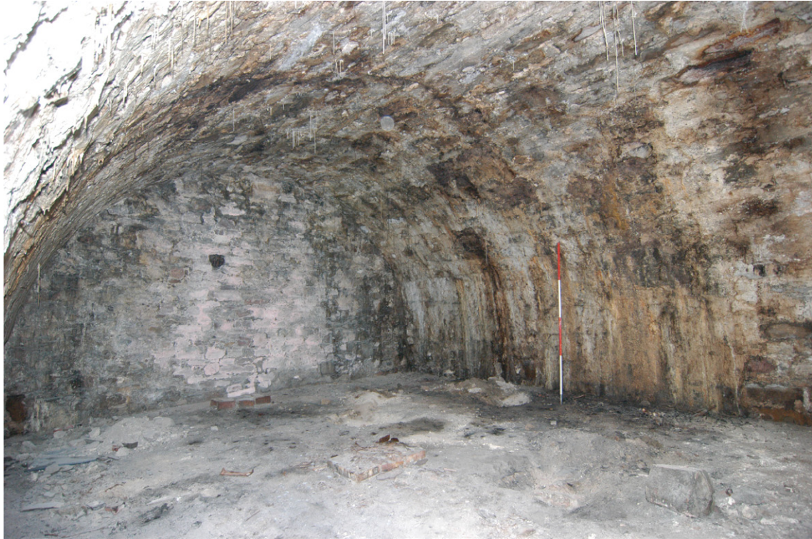
Fig. 6 Interior of the Vault 2
