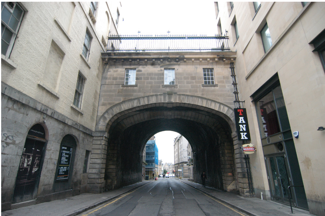
Fig. 9 Exterior west-facing elevation of the Link Bridge
