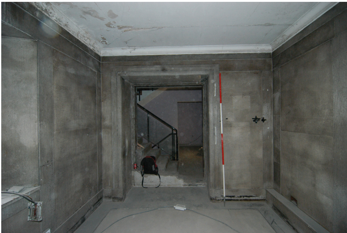
Fig. 13 Moulded door surround on the north entrance
