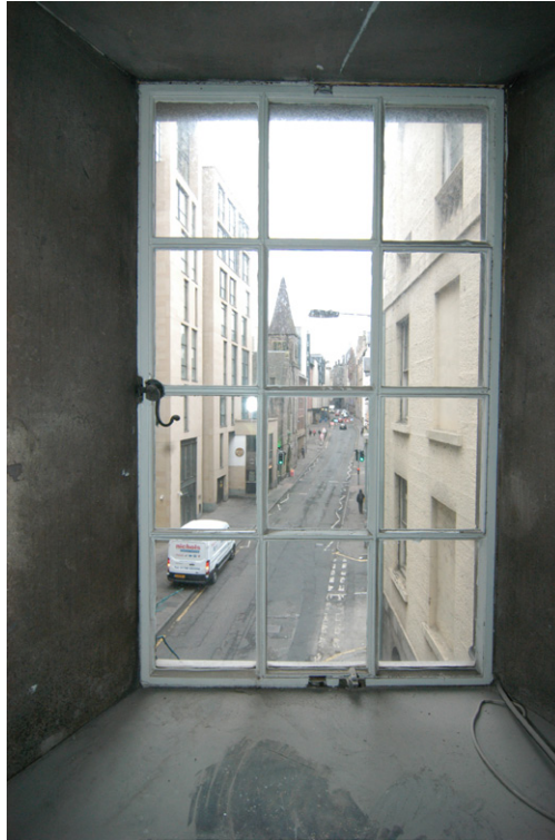
Fig. 12 Northernmost window with original window latch
