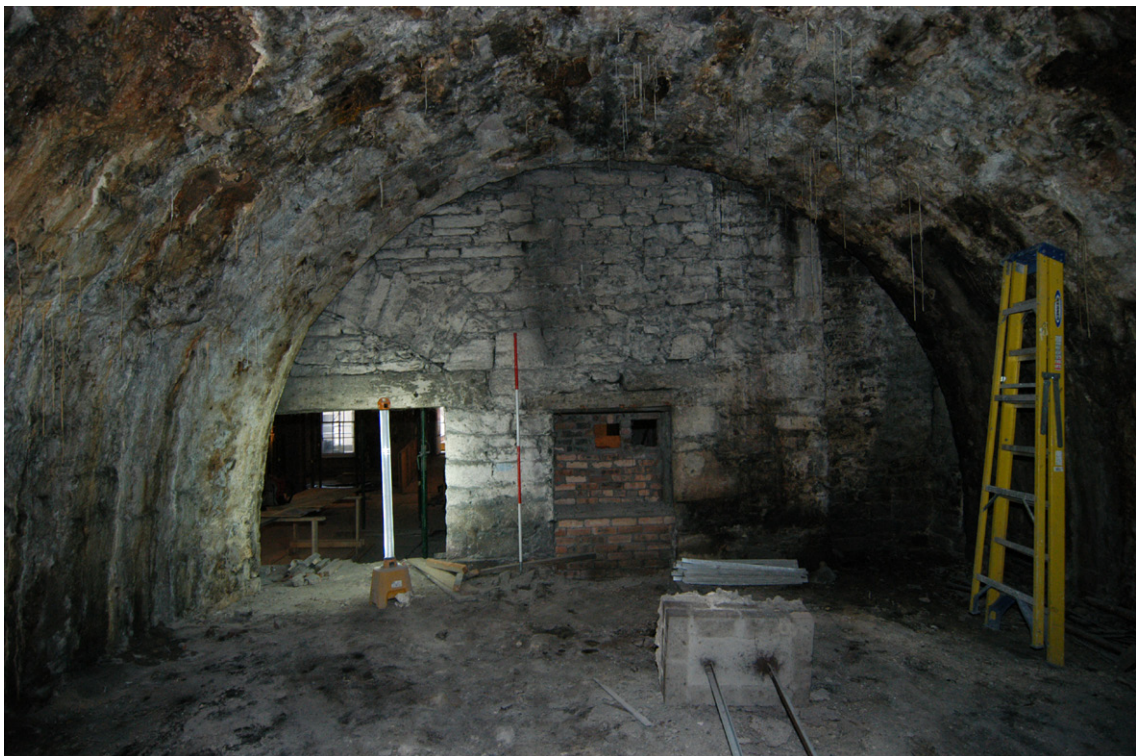
Fig. 5 Vault 1 interior east-facing wall with a central blocked doorway and part of a larger opening with a segmented relieving arch
