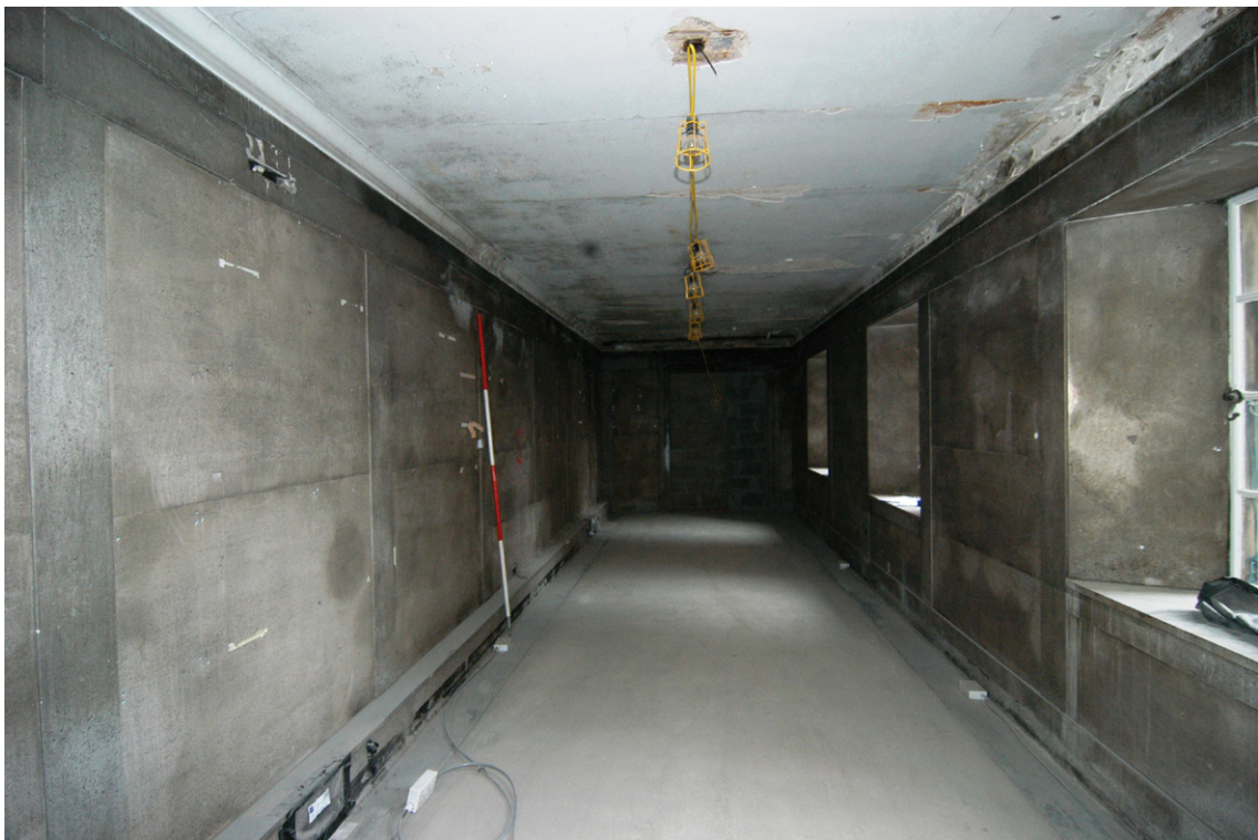
Fig. 11 Interior of the Link Bridge facing south
