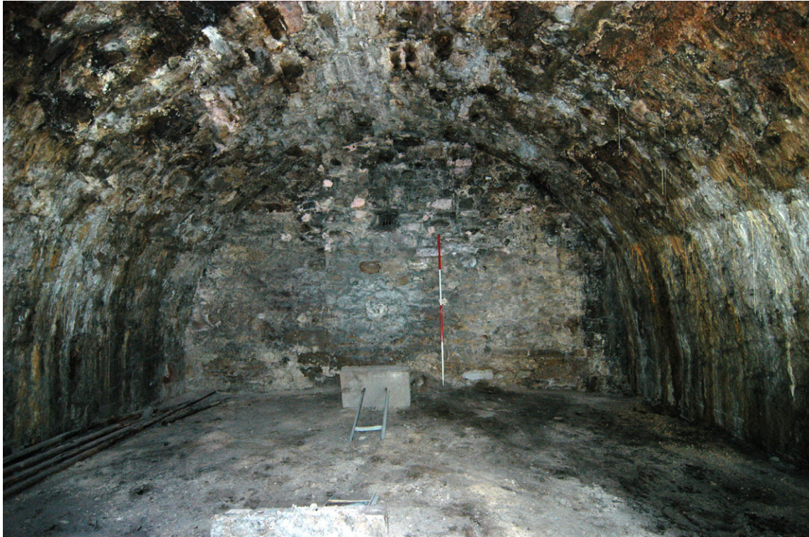
Fig. 4 Interior of the Vault 1
