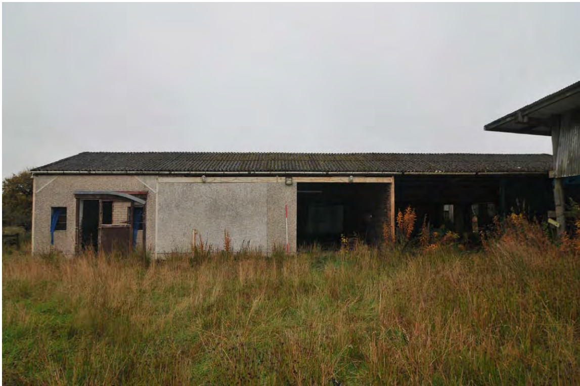
Fig. 17 Unit 12, steel-framed animal shed, west-facing elevation
