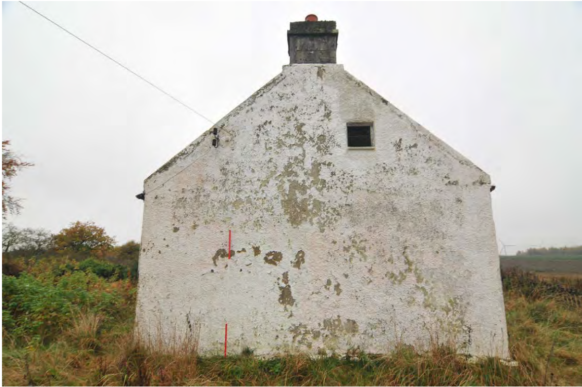
Fig. 4 West-facing elevation of the cottage
