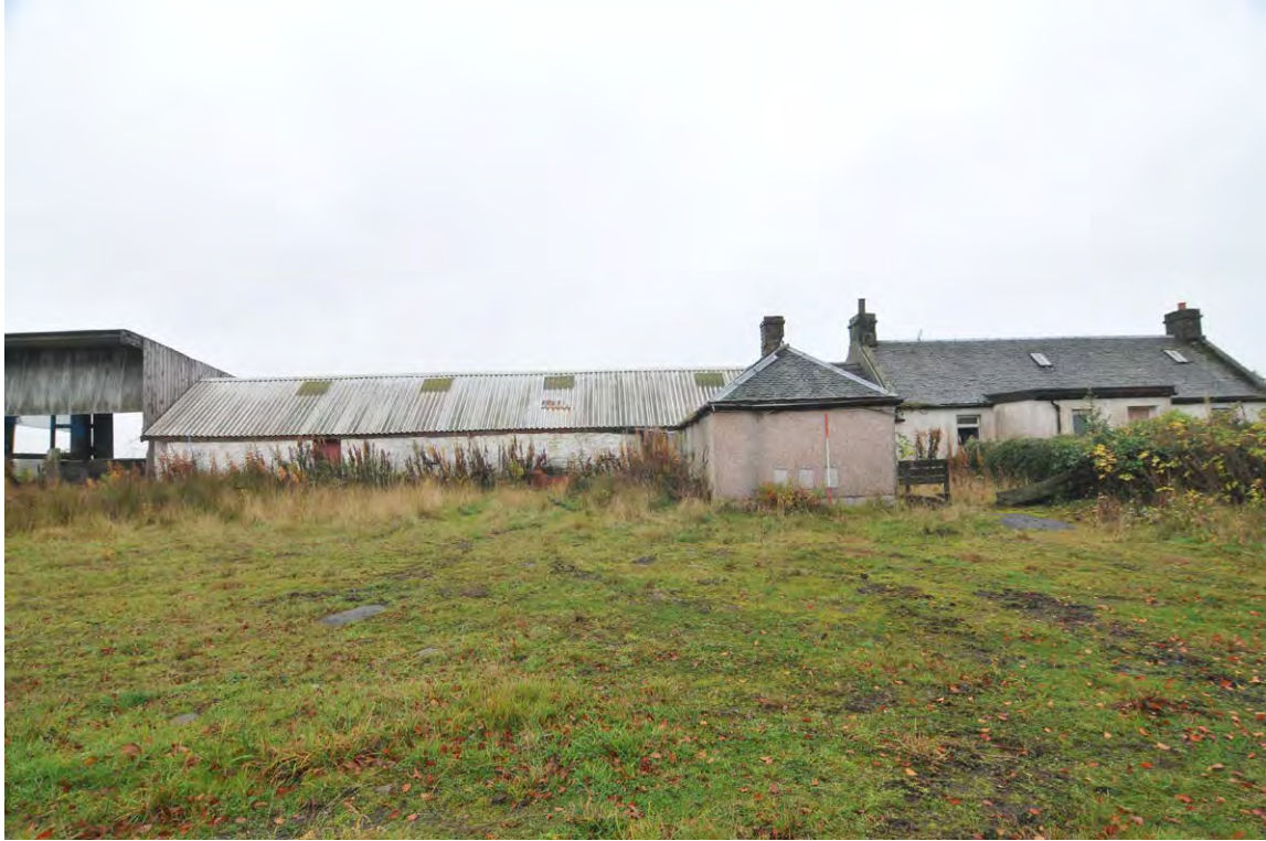
Fig. 14 Unit 8 and 9 Outhouse and byre, north-facing elevation
