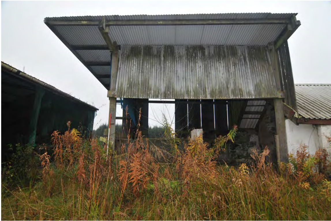
Fig. 16 Unit 11, timber-framed barn, north-facing elevation
