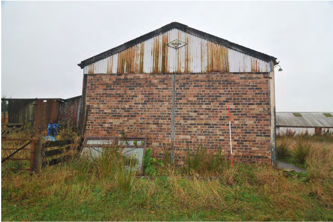
Fig. 18 Unit 12, steel-framed shed, north-facing gable
