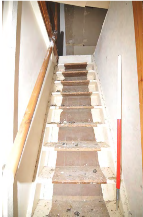
Fig. 10 Wooden staircase between Units 3 and 5
