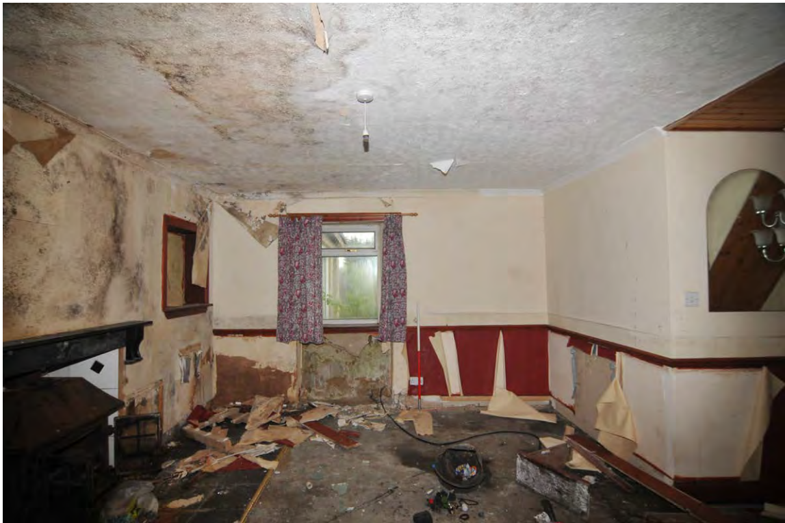
Fig. 9 Unit 4, Living room, north-facing window
