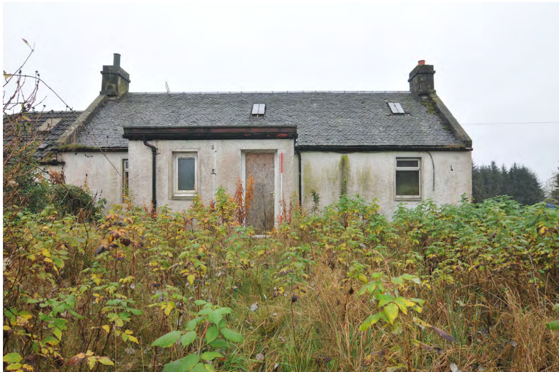
Fig. 3 North-facing elevation of the cottage
