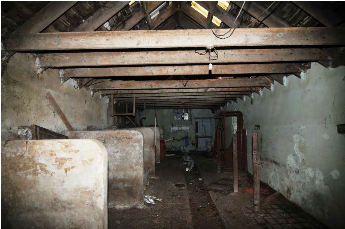
Fig. 15 Unit 9, byre stalls on the north-facing elevation
