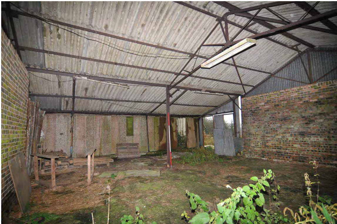
Fig. 19 Unit 12, interior of the steel-framed shed facing, south-east corner
