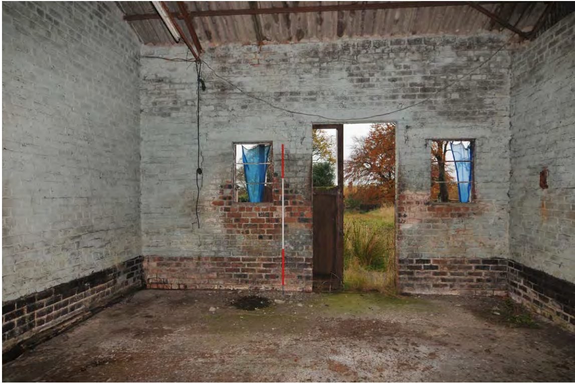
Fig. 20 Unit16, interior of the steel-framed shed, east end
