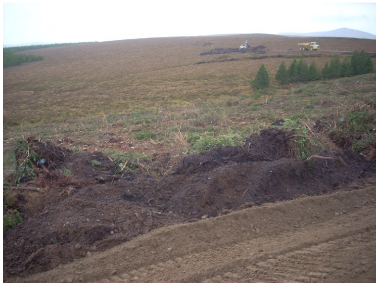
Fig. 13 - General view of the work at T4 from the N
