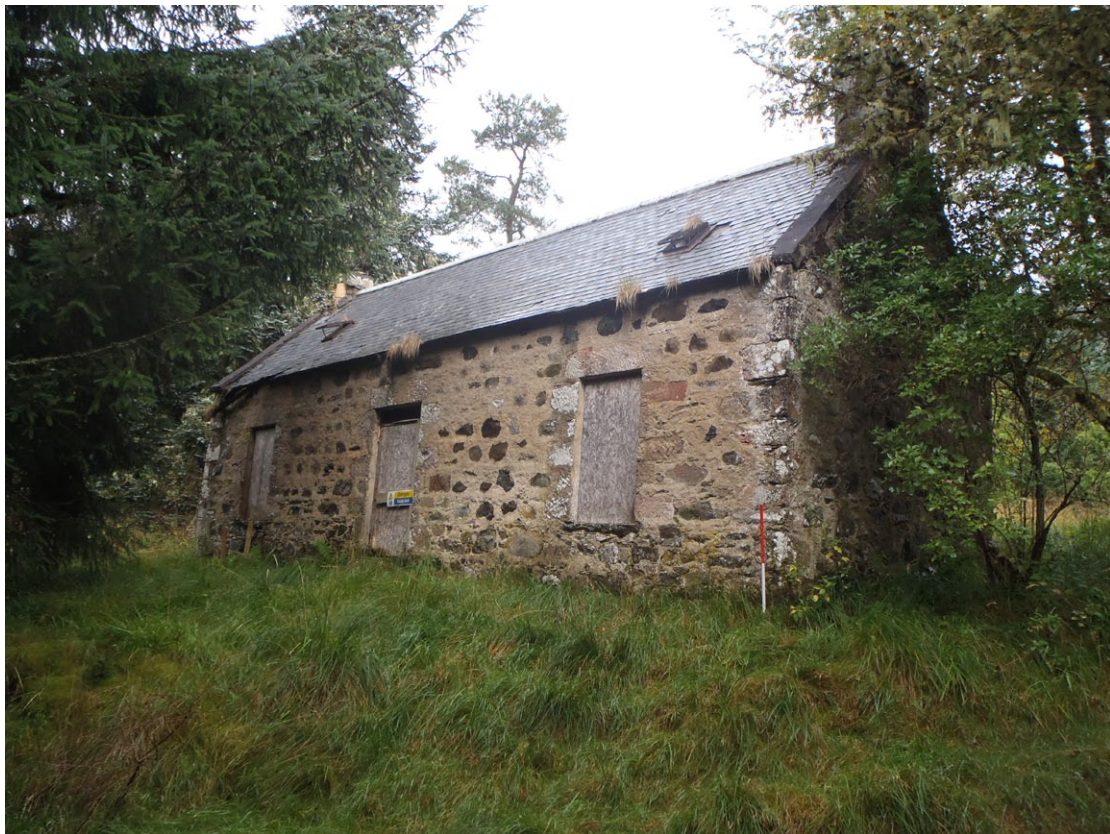
Fig. 7 - View of the farmhouse at Oxter Burn (Site 2)
