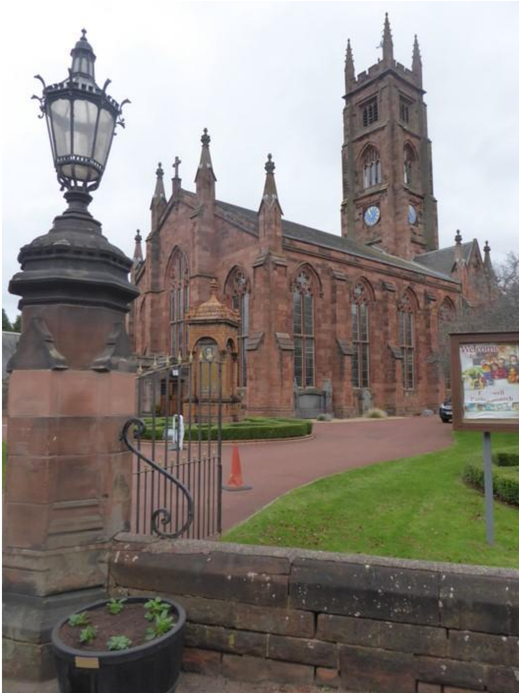
Illus.29 (6.4a) Bothwell Parish Church with view of nave which was built in 1833 and refurbished in 1898. The quire (the roof of which can be seen to the rear) was 4.5 feet lower than the nave, but the two were united by the tower when a massive reconstruction programme took place in 1933 and the floor of the nave was lowered.
