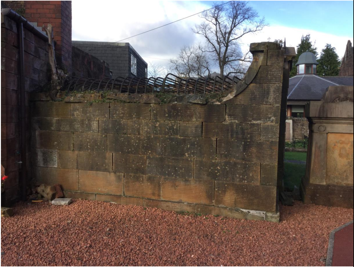
Illus.35 (6.4f) Side view of Hamilton Mausoleum showing structure of iron bars beneath roof designed to foil grave robbers
