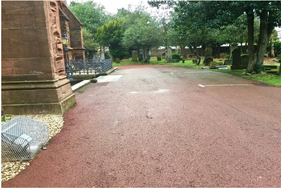
Illus .18 (6.2c) Red tarmac driveway from main gate with parking to the right, changing to red gravel as it winds around behind the church.
