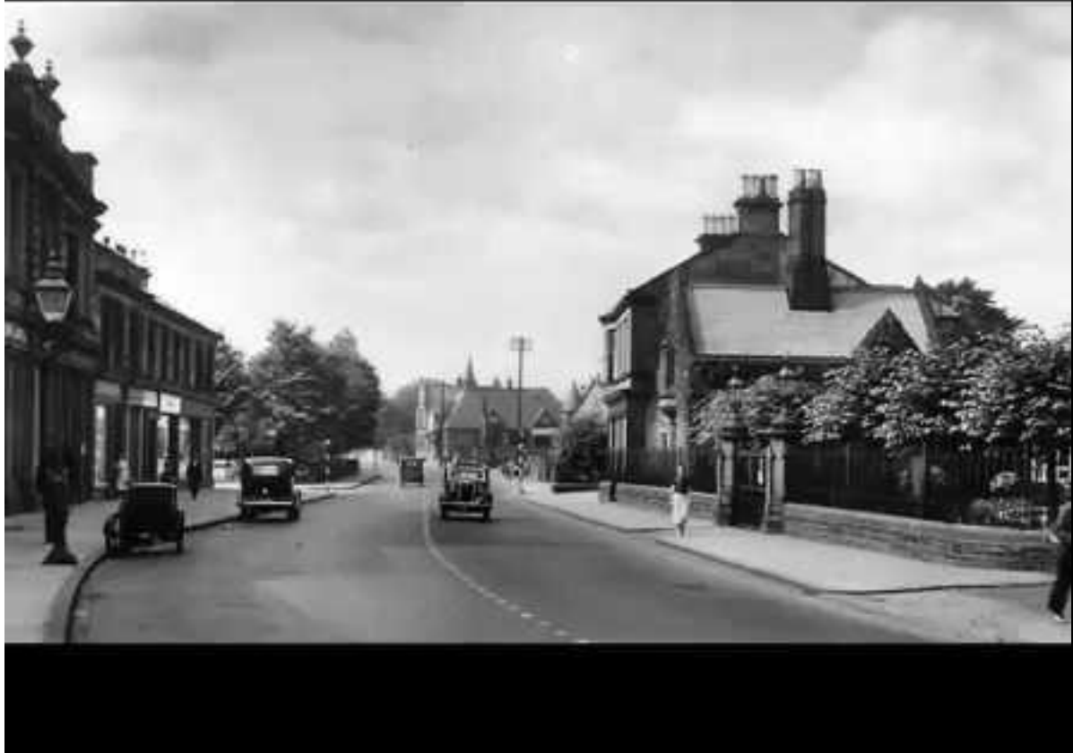
Illus.11 (6.1a) View of Bothwell Main Street with Church Lodge and main gateway to Bothwell Parish Church on right.
