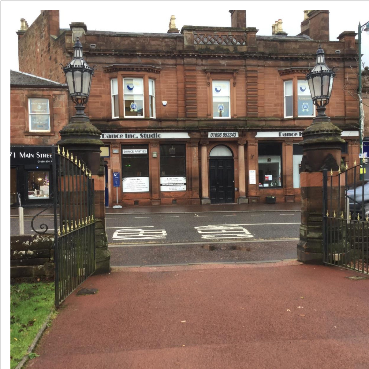
Illus.25 (6.3c) Red sandstone gate piers at main entrance with arrow design and dentilled caps topped by original octagonal gas lanterns, now converted to electricity.
