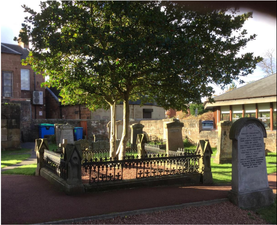
Illus.28 (6.3f) Wrought iron, ornamental railings, in reasonable condition, at Area A.
