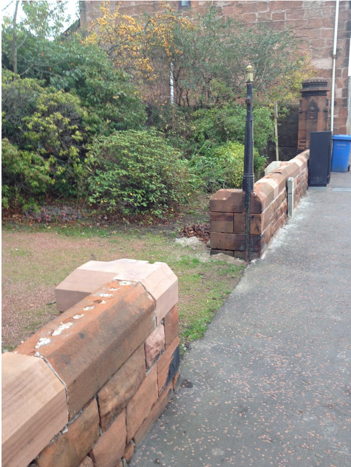
Illus.22 (6.3a) Gateway at Dixon Gate, before restoration of new gate and railings, showing remains of old railings with arrow design matching same on gate piers. Finial on metal post matches dentilled design on pier cap further along.
