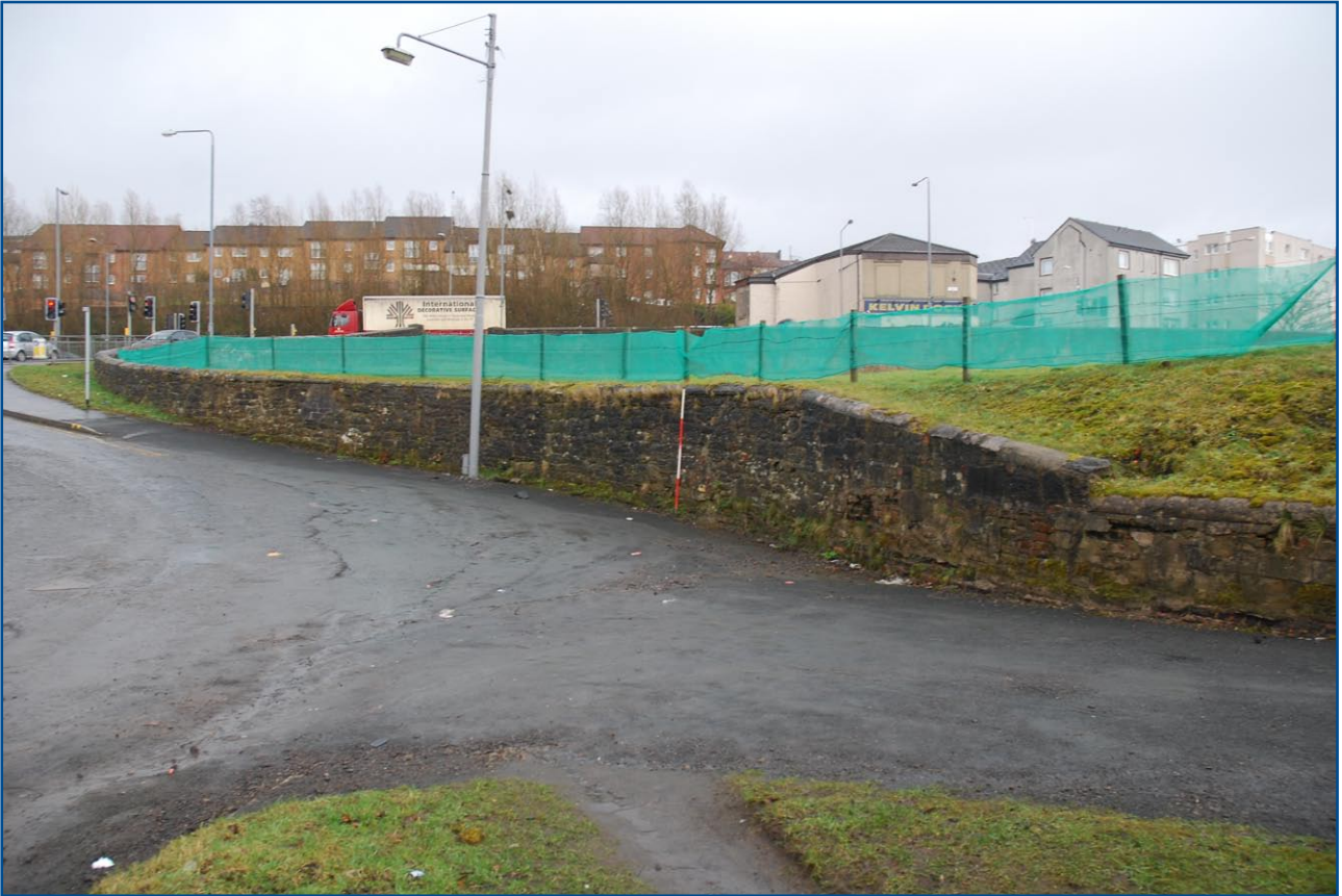
Plate 23: General view of the north wall to Skaethorn Road from NW
