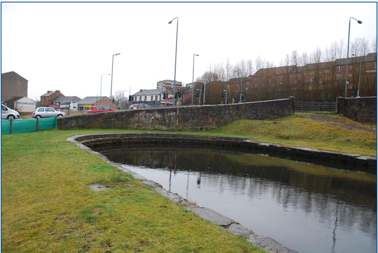
Plate 22: General view of north wall to Skaethorn Road from south
