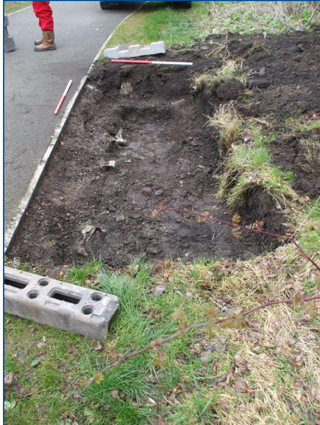
Plate 10: Trench 5 from west
