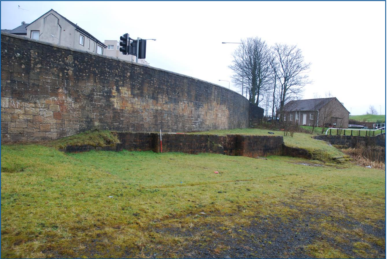
Plate 31: General view of the brick enclosure associated with the slipway from NW
