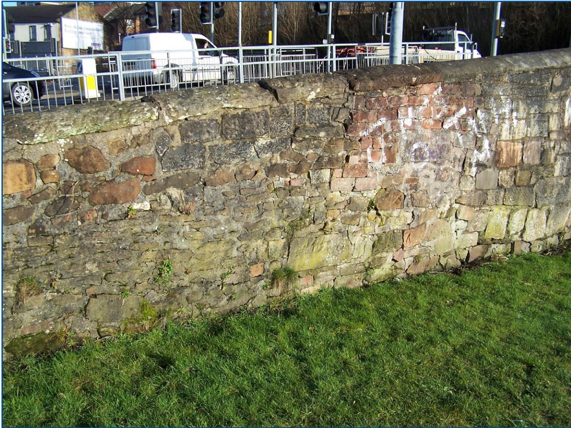
Plate 5: The wall N of the Kelvin Dock from SSW
