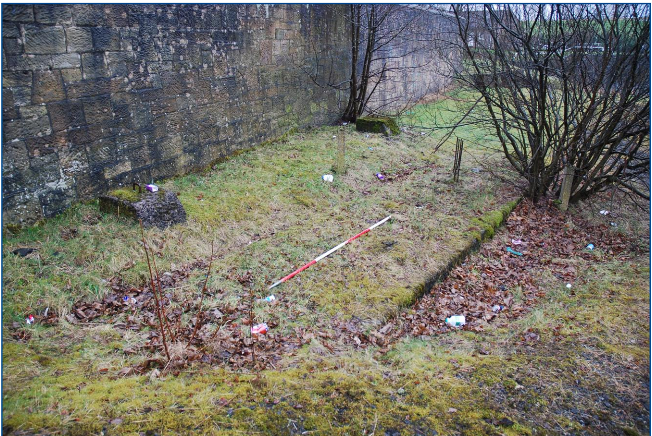
Plate 30: General view of the northern side of the slipway, showing concrete footings and associated fittings from NW
