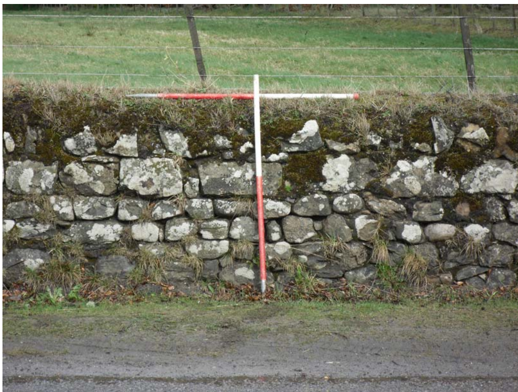
Plate 2: West facing elevation of eastern Knockbreck House Wall
