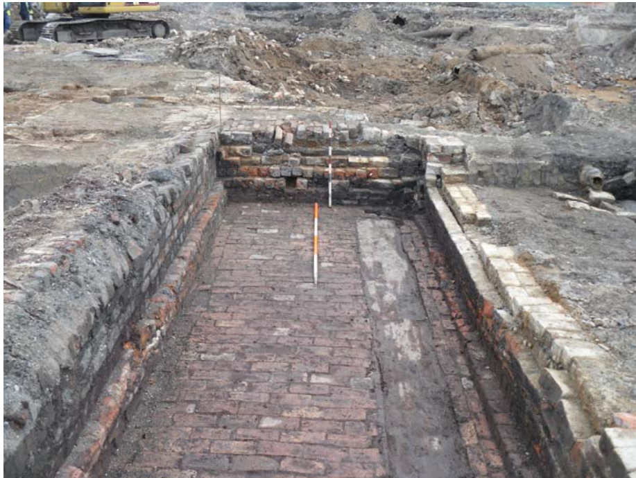
Plate 32: Detail of red brick tank [872], Area 29
