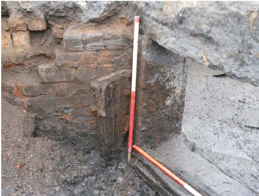
Plate 21: Detail of Glasgow Waterworks Filtering Tower gateway [1671] and wall [1653]
