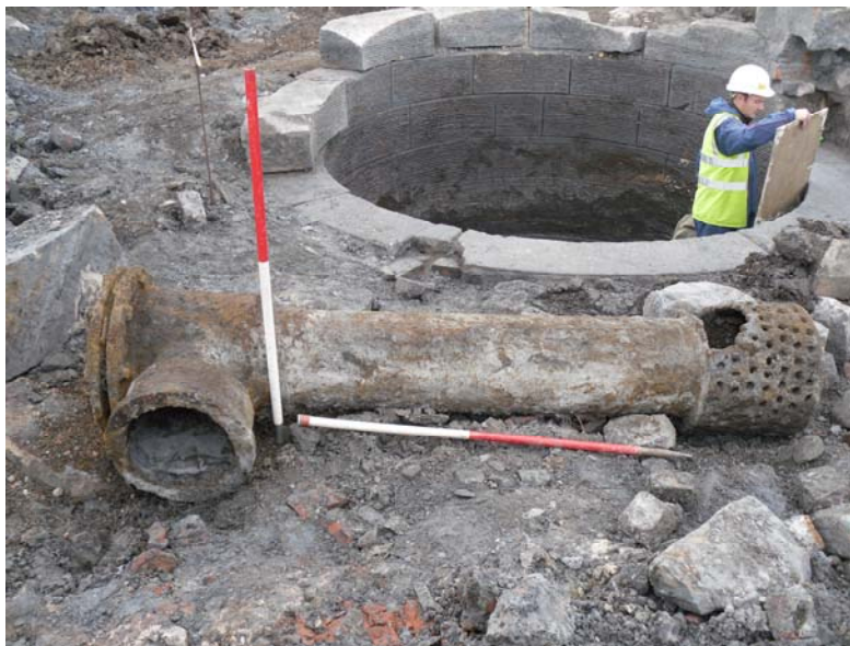
Plate 20: Detail of Glasgow Waterworks Filtering Tower filtering pipe [1661]
