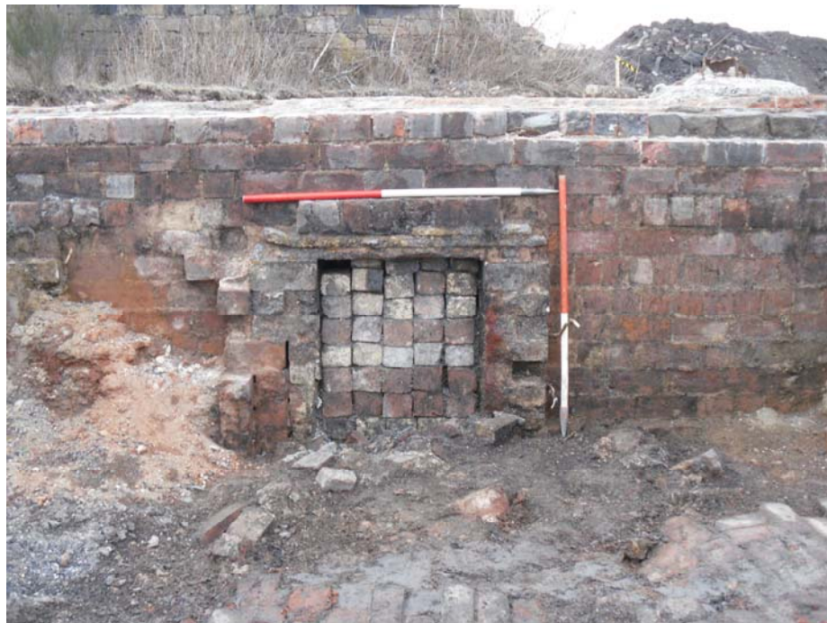
Plate 47: Detail of wall [231] of Building O, with flue entrance [232]
