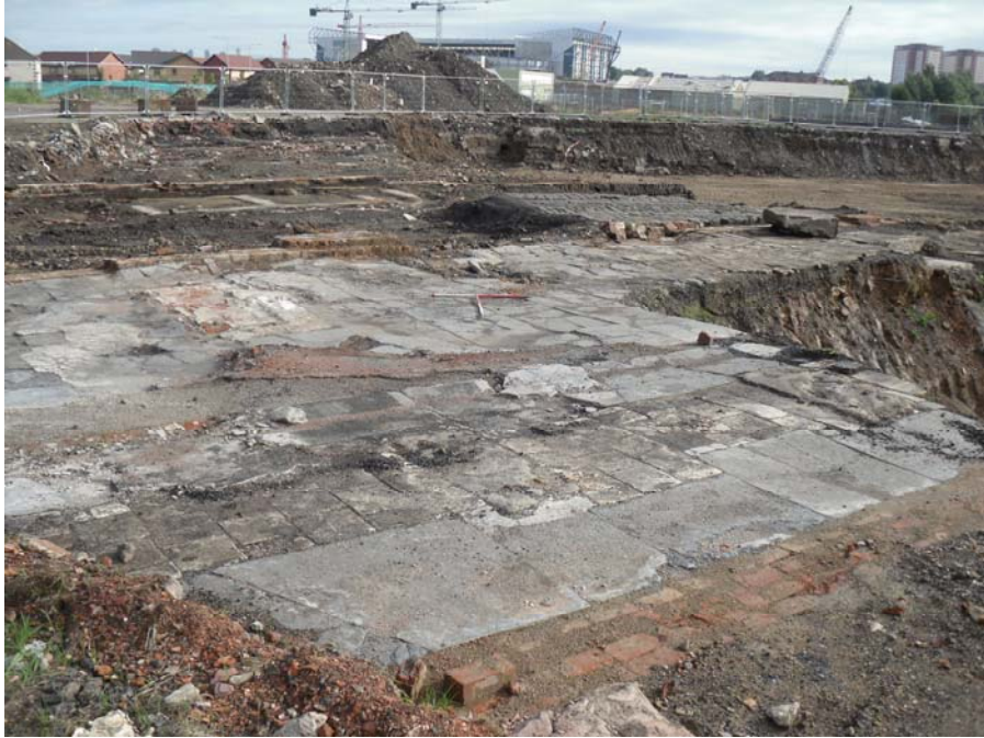
Plate 33: Detail of load bearing wall [1592] and later concrete floor [1590], Area 29
