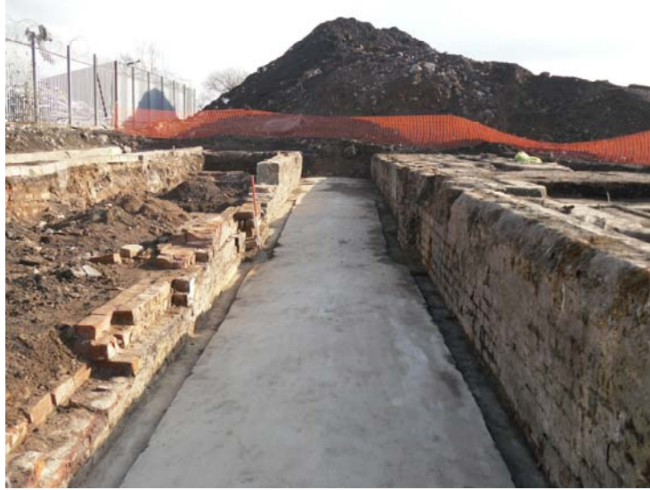
Plate 13: Detail of later machine base overlying earlier Glasgow Waterworks Boilerhouse
