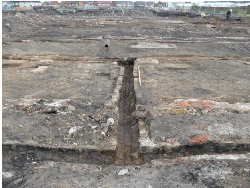
Plate 36: General shot of Building E, with Drain [1032], Area 29
