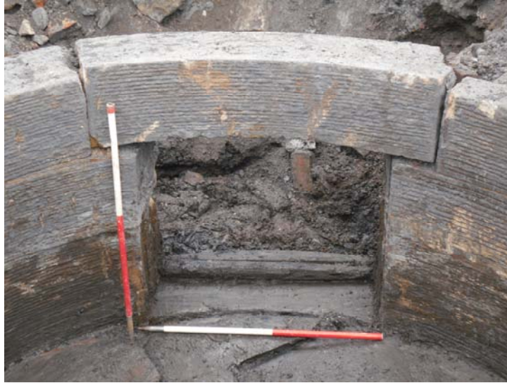
Plate 18: Detail of Glasgow Waterworks Filtering Tower gateway [1671]
