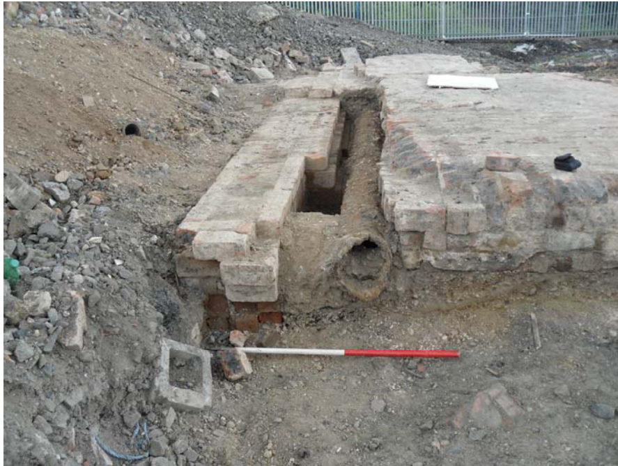
Plate 23: Detail of internal floor [1283] and water pipe [1274], Area 27
