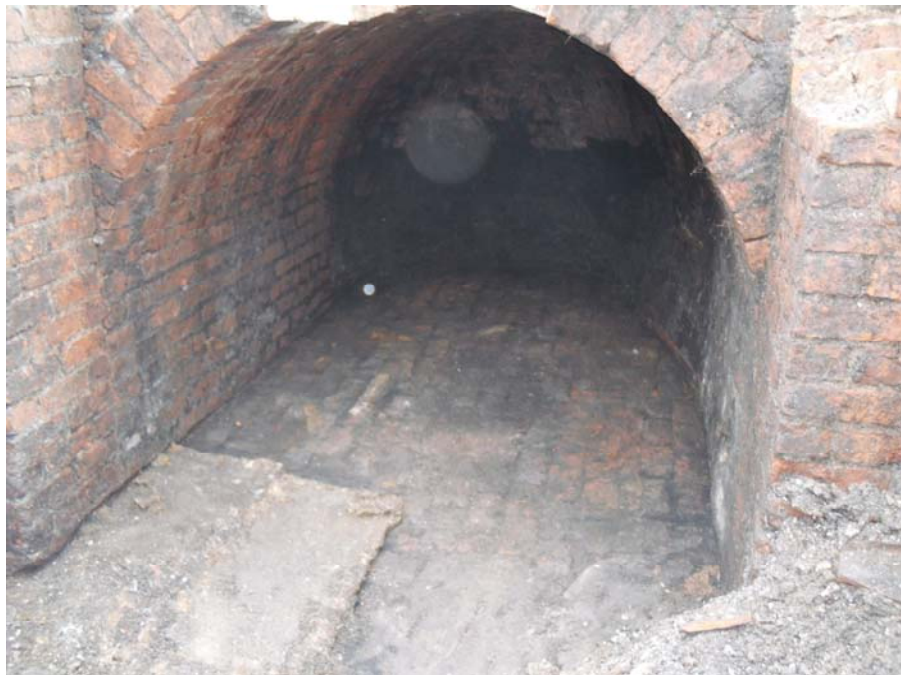
Plate 44: Detail of Coal Bunker [254]
