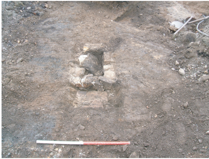
Plate 11: Sandstone culvert 805 with manhole 806 in Trench 8
