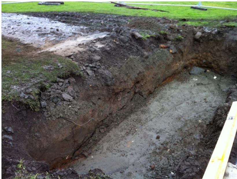
Plate1: Northern foundation trench of Peel Bridge
