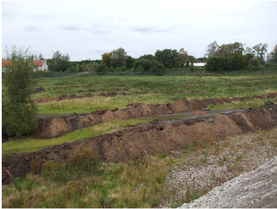
Plate 1: General post-excitation view of Trenches within the rough grassy area
