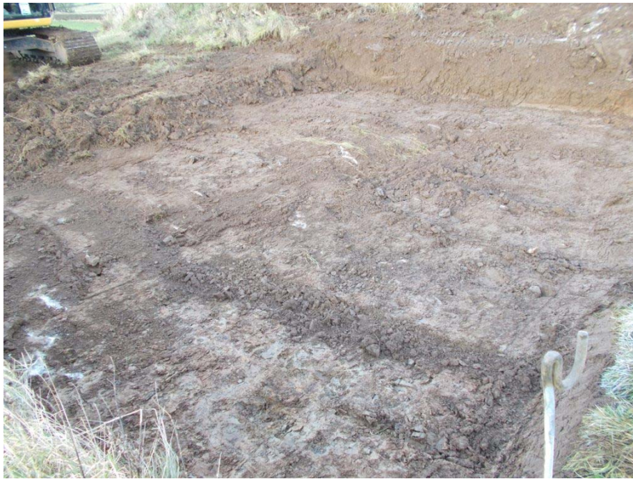
Plate 1 - Post ex view of turbine base
