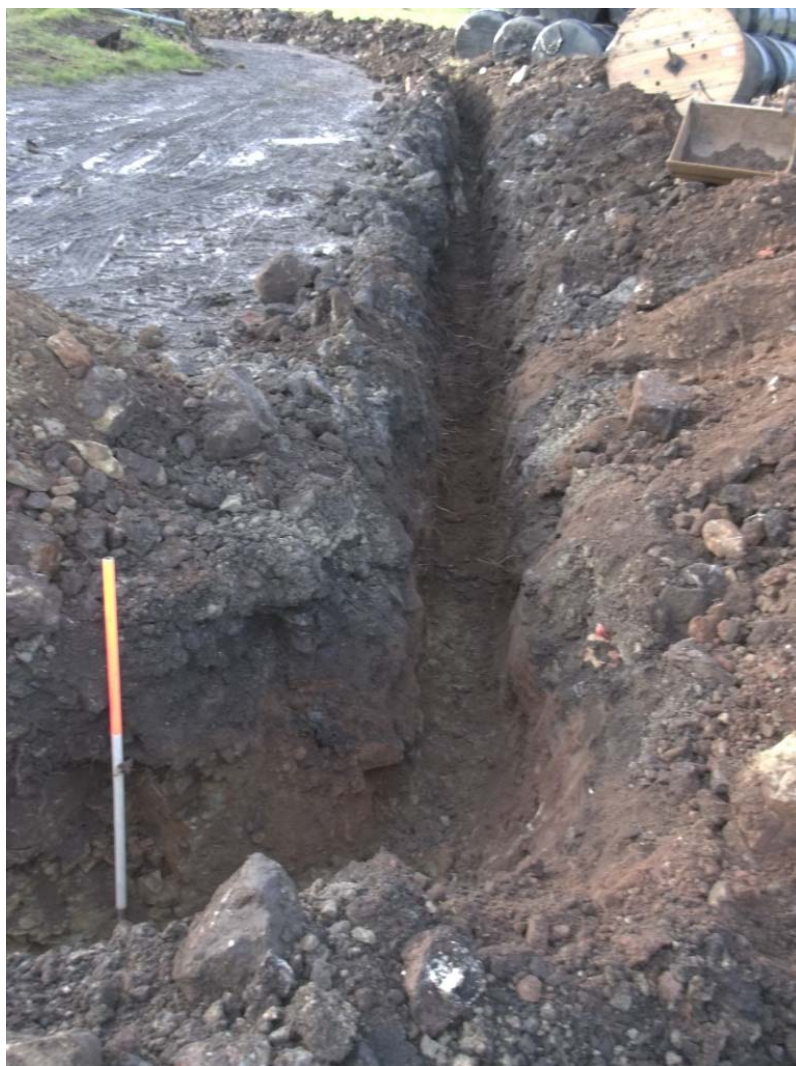
Plate 2 - General view along cable track
