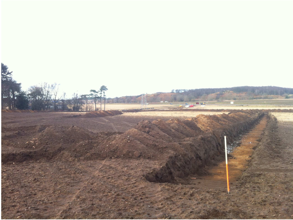
Plate 1: General view of open trenches
