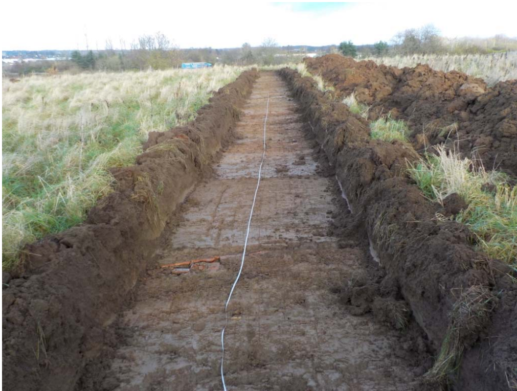
Plate 1 - View of Trench 8
