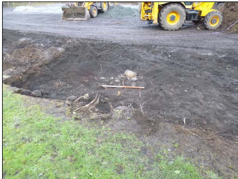
Plate 1- Demolished wall fragment [007] within made ground [013]
