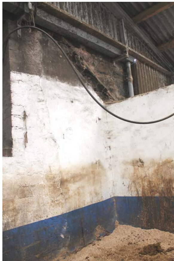
Plate 6: Barn A, north-east elevation, detail of gable scar within the later modern stables from the east
