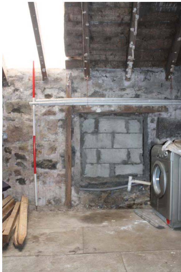
Plate 38: Barn B, detail of blocked hay loft window on the south-west wall from the north-east
