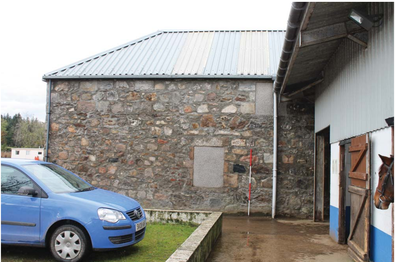
Plate 24: Barn B, south-west elevation, detail of blocked openings to the south-east side from the south-west
