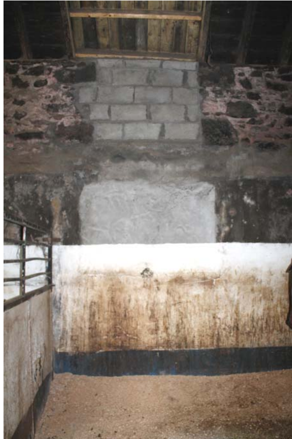
Plate 15: Barn A, detail of blocked openings on the south-west wall from the north-east
