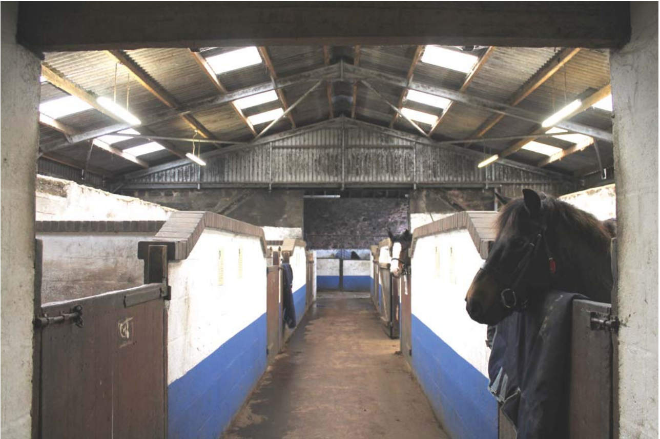
Plate 5: Barn A, north-east elevation, general view of gable scar within the later modern stables from the north-east
