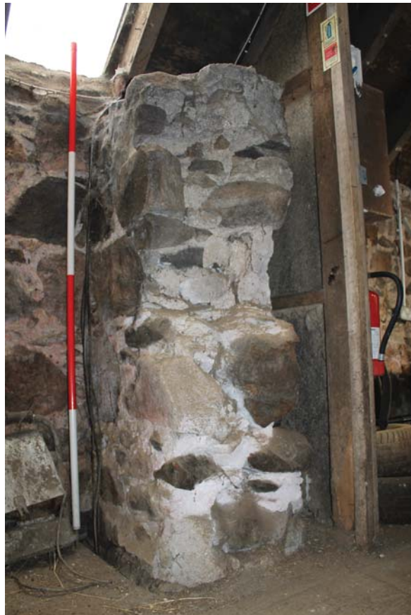
Plate 34: Barn B, detail of broken former gable wall in the upper level of the stables from the west
