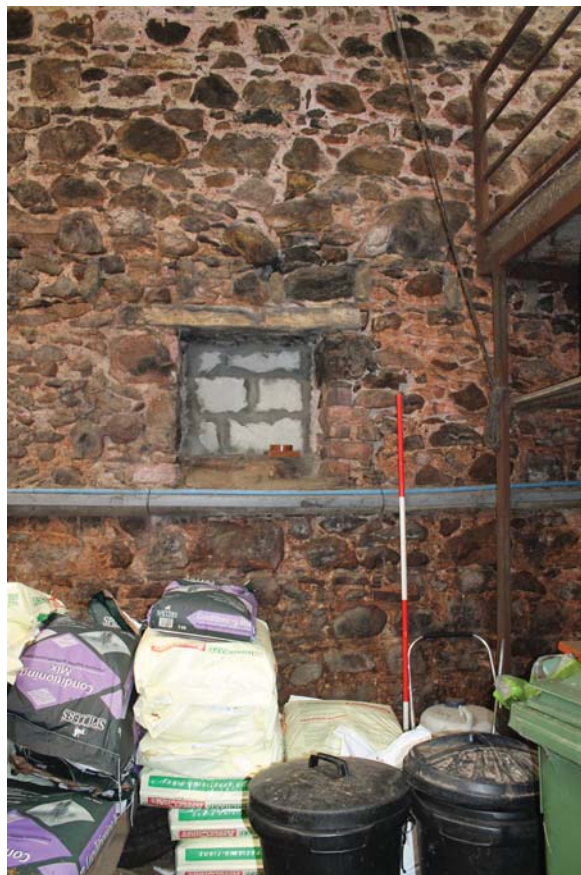
Plate 32: Barn B, detail of blocked window on the north-east wall from the south-west
