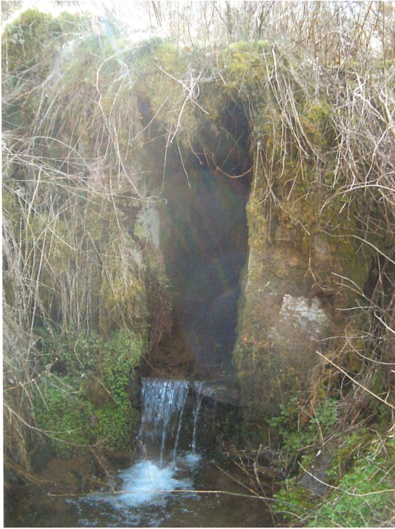
Plate 13: Site 27/30, eastern opening of culvert
