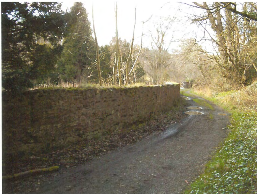
Plate 22: site 35, northern extent of boundary wall
