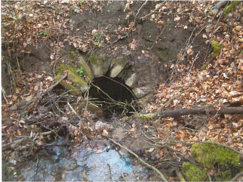
Plate 15: Site 28, upstream opening of culvert
