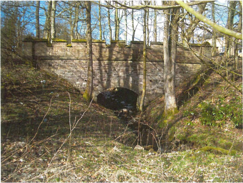
Plate 3: Lesmahagow, South Driveway, Bridge
