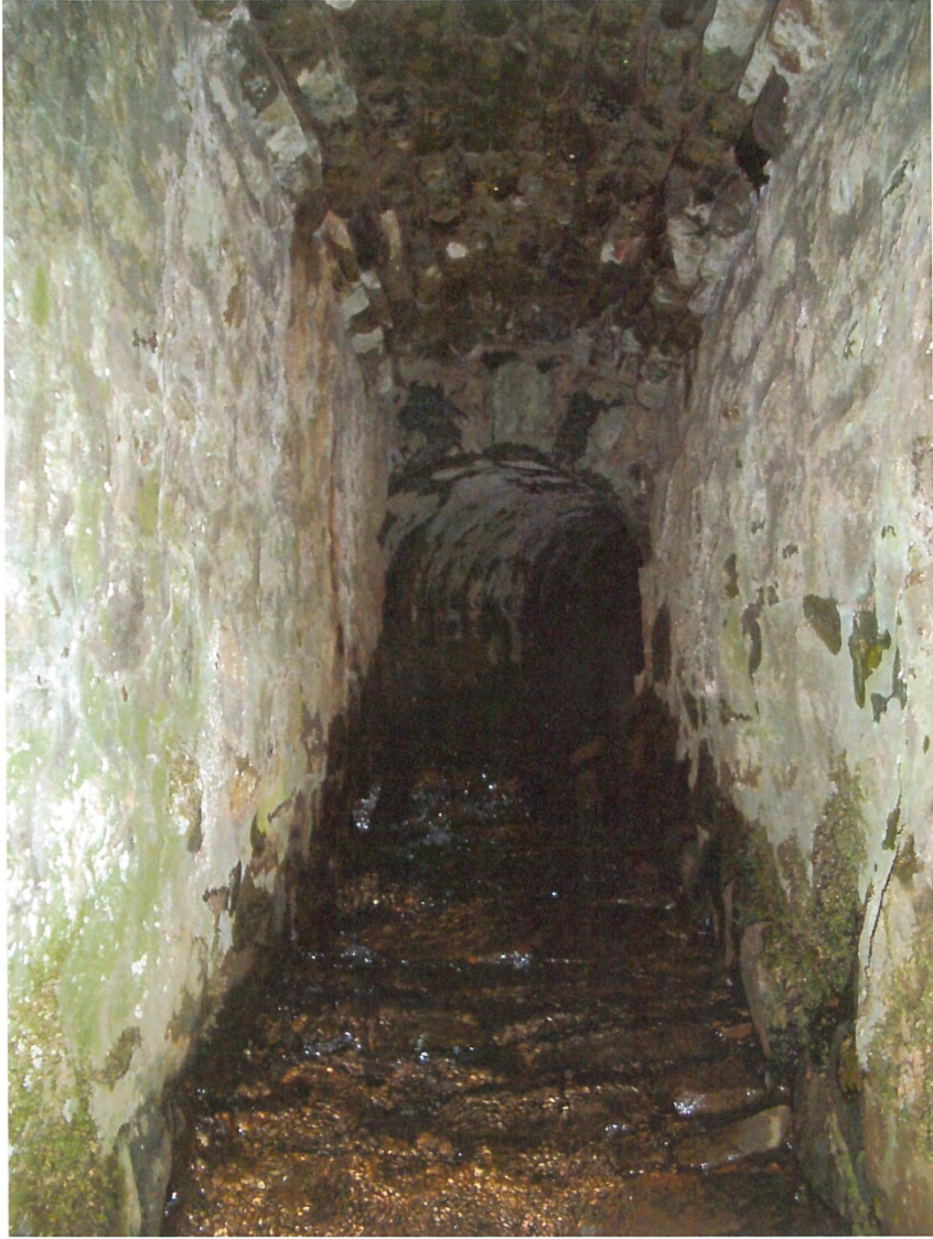
Plate 14: Site 27/30 Internal detail of culvert
