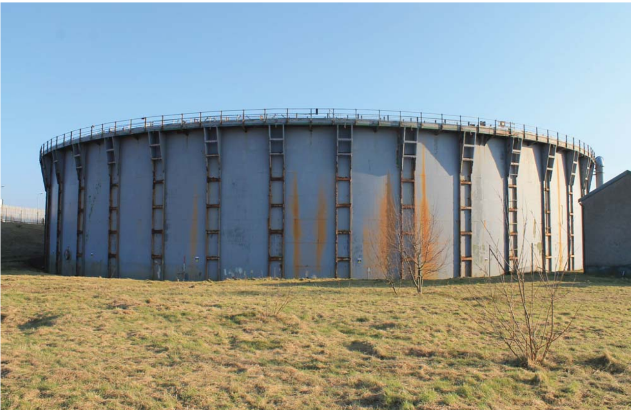
Plate 2: Weir Road, Newtown-on-Ayr, general view of the gasholder from the west
