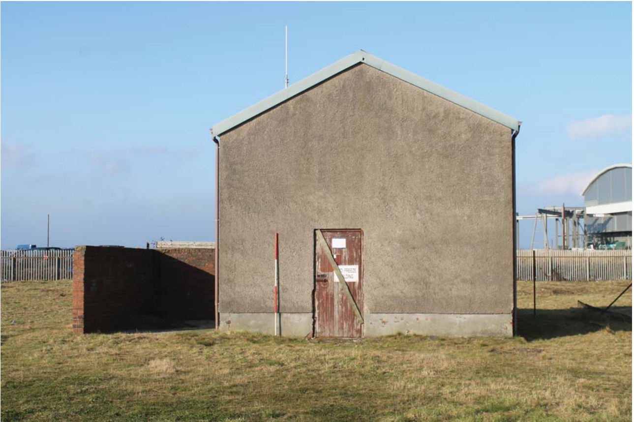
Plate 21: Weir Road, Newtown-on-Ayr, general view of the gasworks buildings from the east
