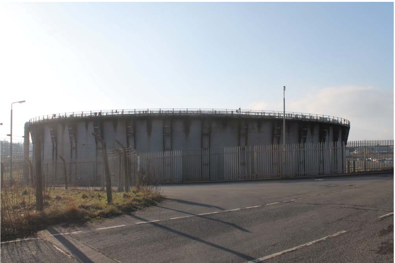
Plate 4: Weir Road, Newtown-on-Ayr, general view of the gasholder from Saltpans Road from the north
