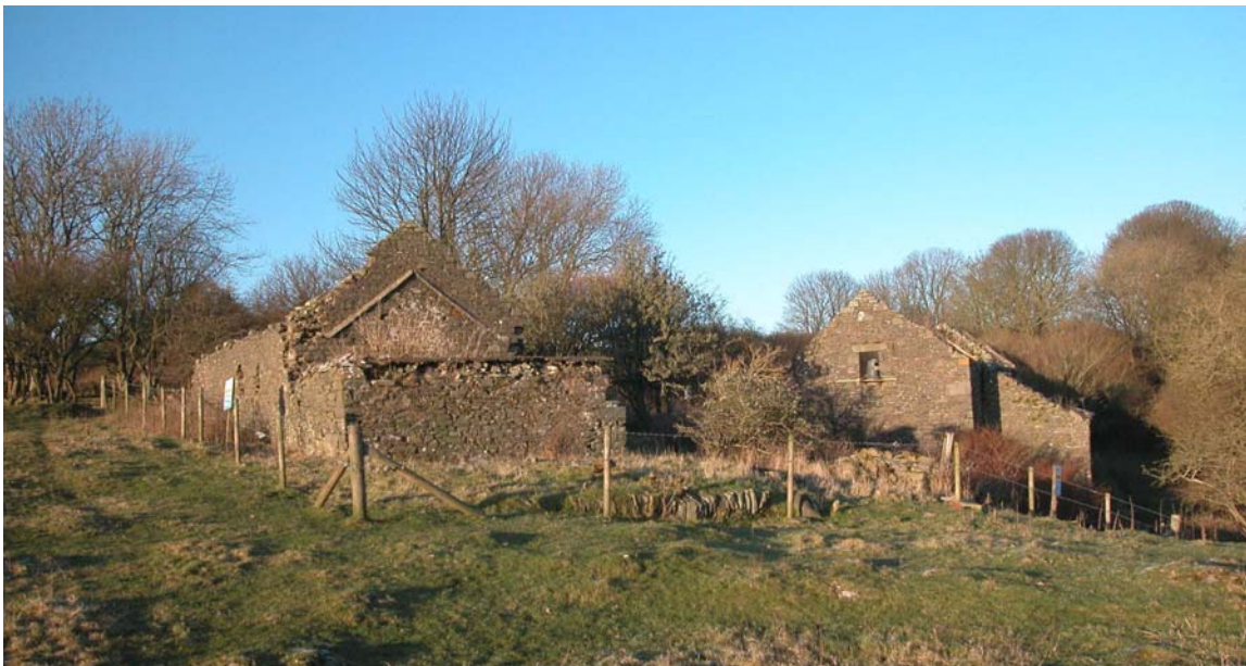
View of Dunrod Mill (right) and adjacent building from the south.
