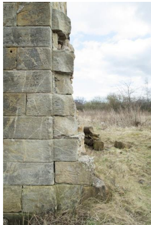
Above left and right: south west corner of engine house showing raggle wall. The masonry is clearly keyed into the engine south wall of the engine house, suggesting that the south range was built at the same time. [DP232016 and DP232015, HES]
