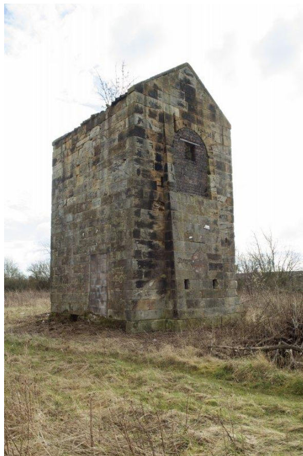
View from north west [DP 231994, HES]
