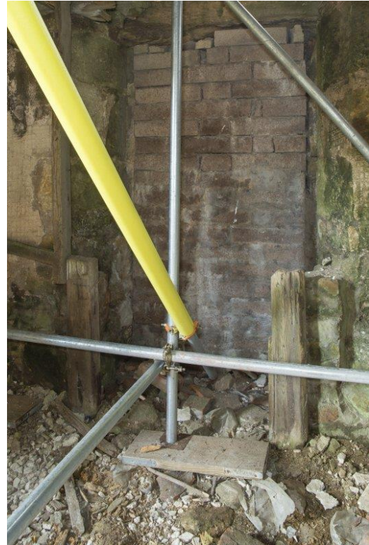
Above: Interior view of blocked east gable doorway with later brick built wing walls and wood facing. The east doorway may have originally been a window. [DP254023, HES]
