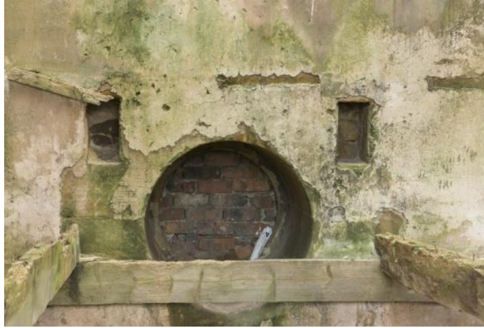
Above: View of interior, west elevation: Ground/First Level. Detail of socket holes and delivery pipe from the pump riser. [DP231999, HES]
