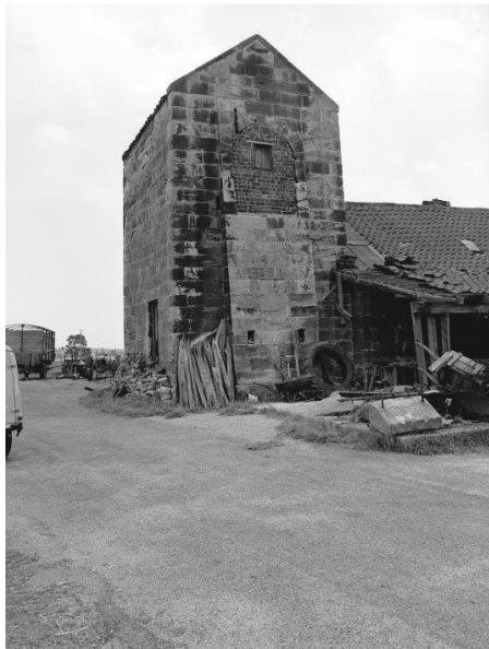
Left: View of Pump Engine House from west, showing the now demolished south range (right). Some of the now demolished buildings may have been part of the colliery. The low footings visible in front of the west wall is the backfilled shaft down which the pump rods of the engine ran. Men may also have used the shaft to get out of the mine workings at the end of their shift. [SC 454959, 1974, John R Hume Collection, National Record of the Historic Environment]
