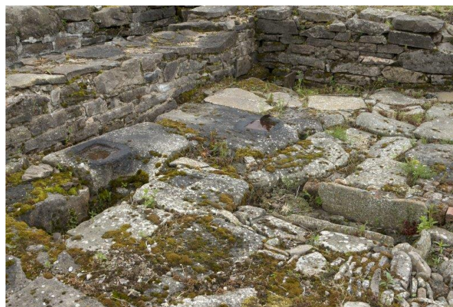
View of floor of 18th century lint mill with later features at the west end of the North Mill. The metal plates visible are the possible remains of the bone crushing machine with the waterwheel pit (extreme left) [DP 237893, HES]
