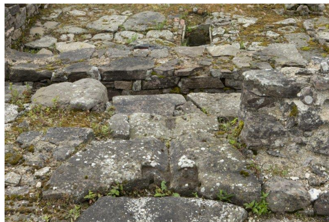
View of remnants of waterwheel shaft and bearing mount - the stones has been cut to take the metal bearing components, west end of North Mill [DP 237890, HES]
