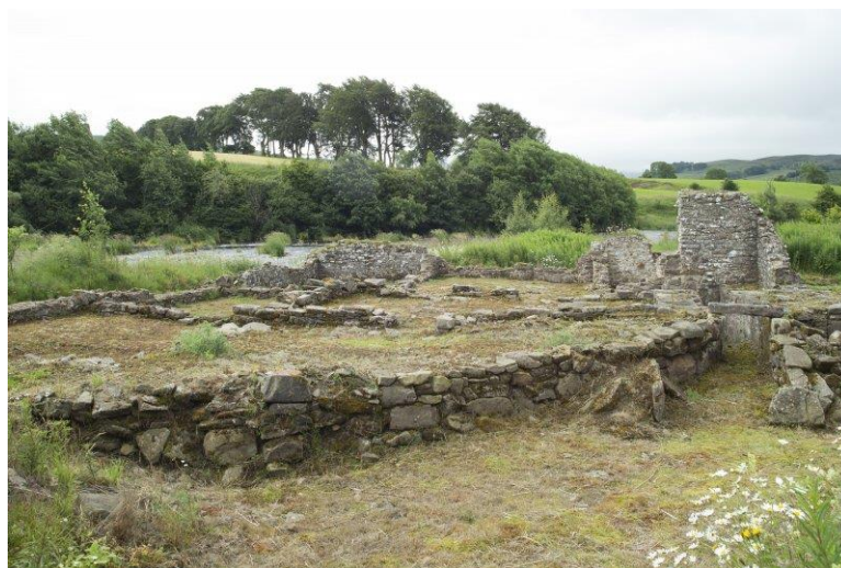
View from north east across North Mill foundations with the lade on the right [DP 237887, HES].
