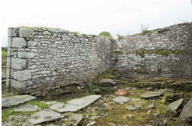
View of interior of remains of South Mill from north. The lade is beyond the wall on the right and the remnants of the double door entrance can be seen (left) [DP 237910, HES]
