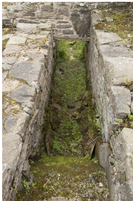
View from north of North Mill waterwheel pit. Here we see the remains of the metal 'shrouds' of the waterwheel. These 'shrouds' held the 'buckets' in place. [DP 237928, HES].
