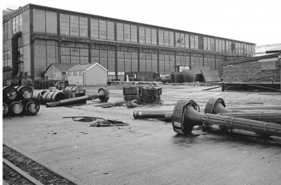
Above left: East wall of Bay A from south east showing original fenestration, beam which supported the 15 Ton Gantry crane which operated in the open yard (SC557091, JR Hume Collection, RCAHMS, 1978). Above right: Bay A from south showing original fenestration, steel stanchions and beam supporting the two 15 Ton electric overhead travelling cranes (SC518165, JR Hume Collection, RCAHMS, 1978)
