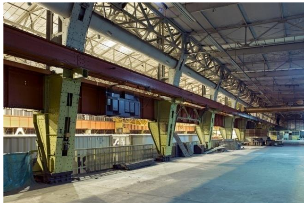
Above left: General view of Bays A-C (centre) showing extent of original glazing and Bays D-G (right). (SC581133, JR Hume Collection, RCAHMS, 1978) Above right: General view of Bay A and B upper level (originally light engineering 'gallery' from south). On the left, the columns show the 'hinged' bearing which site on the gallery's concrete floor. The beam that can be seen running the length of the Bay is the east rail for the three Electric Overhead Travelling cranes. (DP172002, RCAHMS, 2013)
