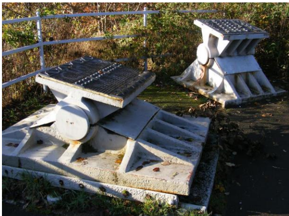
Above left: Hinged bearing, Bilston Glen Viaduct, Midlothian. This is the same type as used at Barclay Curle and is a German/European practice. (Image: Mark Watson, 1999). Above right: Former fabrication shop showing the original glazed roof. The west wall can be glimpsed on the right. (SC518201, JR Hume Collection, RCAHMS, 1978)
