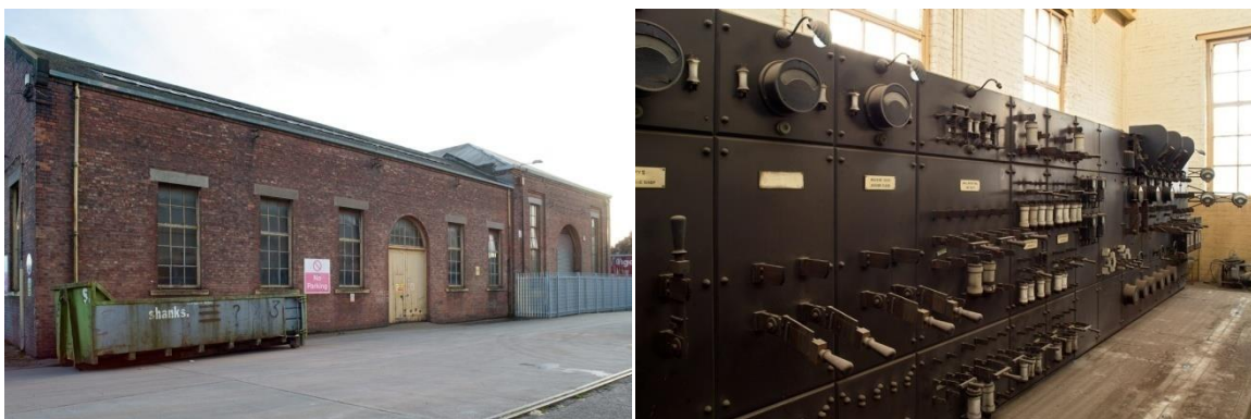
Above left: Power House with Boiler House on right. (DP171755, RCAHMS, 2013). Above right: Interior of Power House. Control panel for the works from south east. (DP171755, RCAHMS, 2013)
