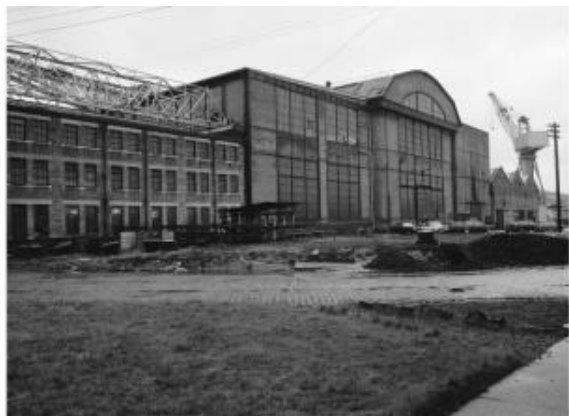
Above left: General view of Bays A-C (centre) showing extent of original glazing and Bays D-G (right). (SC581133, JR Hume Collection, RCAHMS, 1978) Above right: General view of Bay A and B upper level (originally light engineering 'gallery' from south). On the left, the columns show the 'hinged' bearing which site on the gallery's concrete floor. The beam that can be seen running the length of the Bay is the east rail for the three Electric Overhead Travelling cranes. (DP172002, RCAHMS, 2013)
