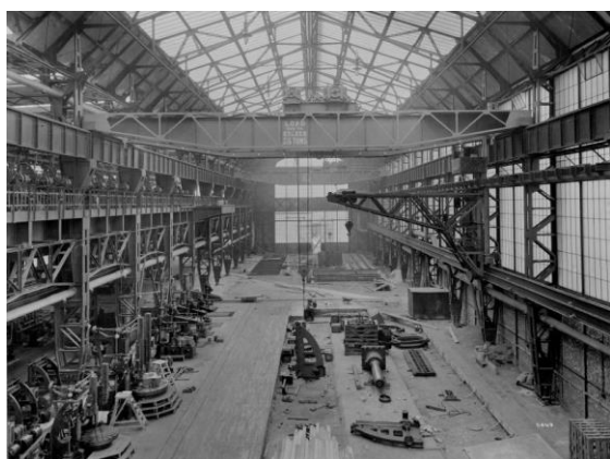
Above left: Bay C, main workshop from north showing the original fenestration, west wall, jib cranes and both 75 Ton electric overheat travelling cranes and the upper open gallery Bay B on the left. (SC1021309, RCAHMS, c.1914) Above right: Site from south. From left, Bay C, Bays A and B in middle, and 15 Ton gantry crane and yard on right (SC603744, JR Hume Collection, RCAHMS, 1978)
