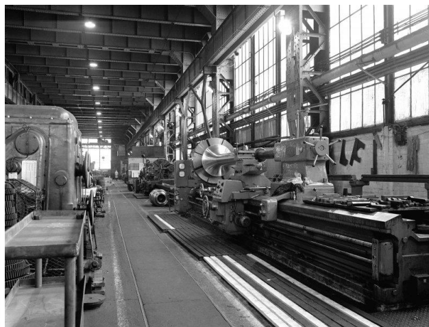
Above left: East wall of Bay A from south east showing original fenestration, beam which supported the 15 Ton Gantry crane which operated in the open yard (SC557091, JR Hume Collection, RCAHMS, 1978). Above right: Bay A from south showing original fenestration, steel stanchions and beam supporting the two 15 Ton electric overhead travelling cranes (SC518165, JR Hume Collection, RCAHMS, 1978)
