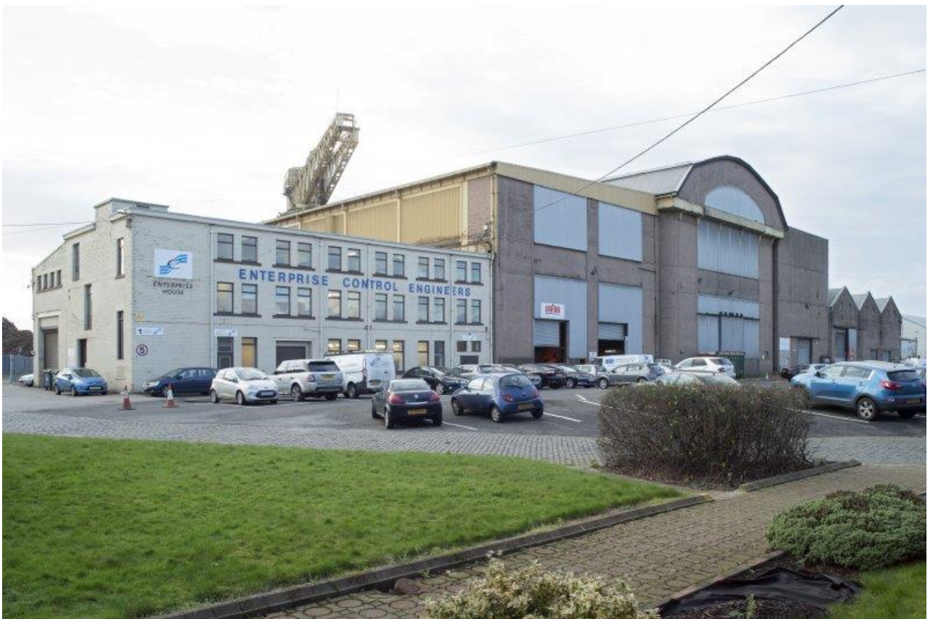
North elevation with giant cantilever crane in background (DP171994, RCAHMS, 2013)
