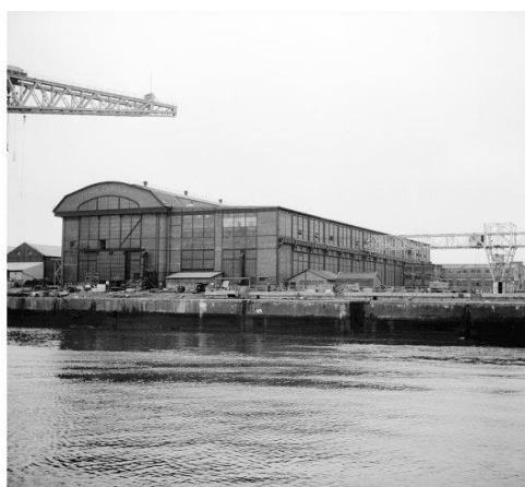
Above left: Bay C, main workshop from north showing the original fenestration, west wall, jib cranes and both 75 Ton electric overheat travelling cranes and the upper open gallery Bay B on the left. (SC1021309, RCAHMS, c.1914) Above right: Site from south. From left, Bay C, Bays A and B in middle, and 15 Ton gantry crane and yard on right (SC603744, JR Hume Collection, RCAHMS, 1978)
