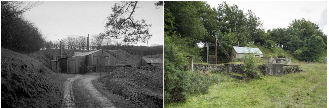
Left: Dalmore Mine photographed by J R Hume 1967 from the north. The timber buildings of board and batten build have been demolished (SC682116). The headgear and just glimpsed winding engine house survive. Right, the site today (DP162521) with the steel winding gear and electric winder which was originally a marine winding engine
