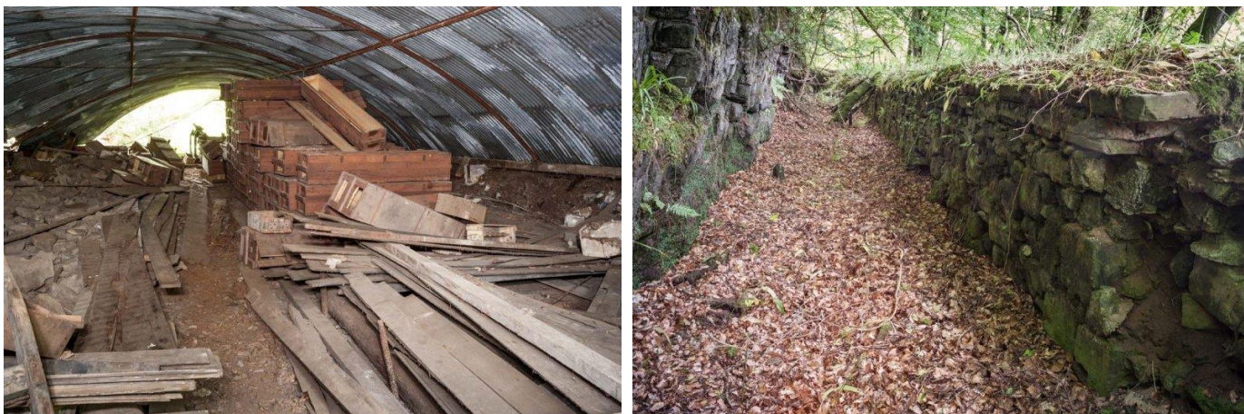
Left: Interior of storage shed 2 looking north (DP162032). Right: View along lade from east (DP161996)
