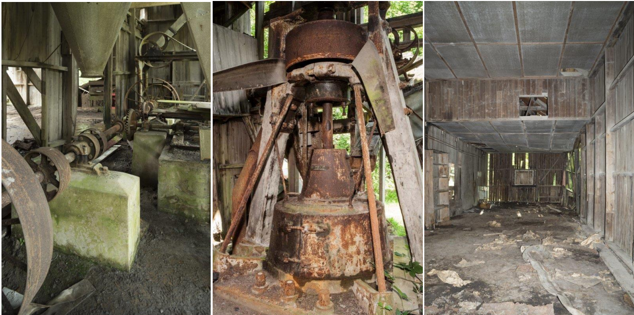
Above left to right: Drive shaft at Dalmore [DP170540, 2013, HES]; view of the Griffin Mill pulveriser (DP160205) - storage and former engine room from East showing the roof height difference between the two adjacent north sheds [DP170551, 2013, HES]
