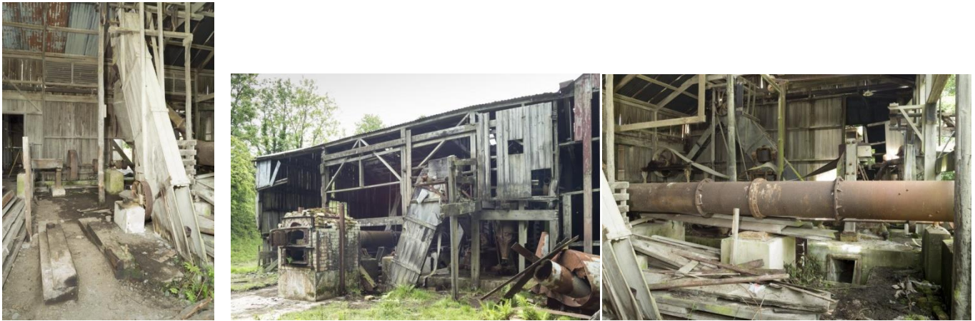
Stone crushing and grinding works. Left to right: wooden planks which originally supported a crusher with the bucket elevator to right carrying crushed material to the top of rotary dryer [DP170536, 2013, HES]; the furnace which heated the rotary dryer with the bucket elevator to its right carrying dried crushed material to the pulveriser [DP170532, 2013, HES]; the rotary dryer, the rivets which attach the vanes to the interior of the dryer drum can be seen [DP170535, 2013, HES]
