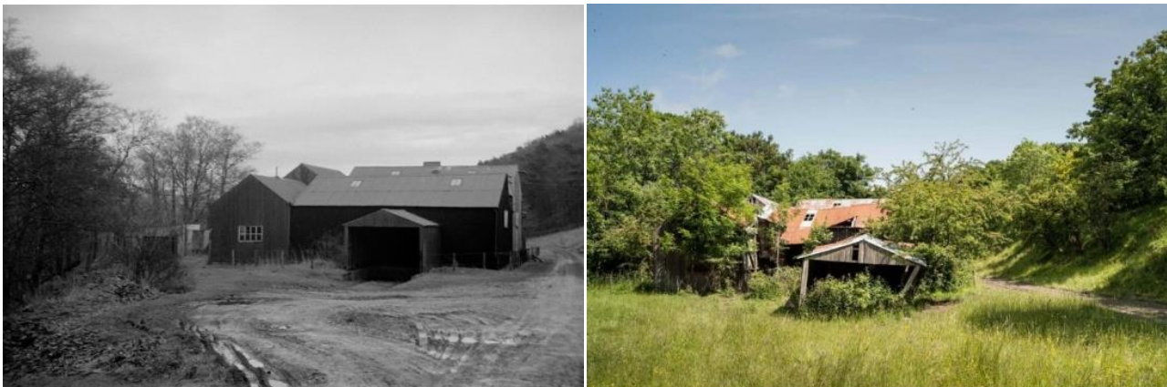
Left: works from west, 1967 [SC682115, 1967, John Hume Collection, HES] with lorry access area, and right, in 2013 [DP170553, 2013, HES]
