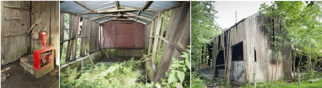
Above left to right: Weigh machine in bagging area from South West [DP170547, 2013, HES]; interior of lorry loading area from West (DP170544); building from North West [DP170545, 2013, HES]
