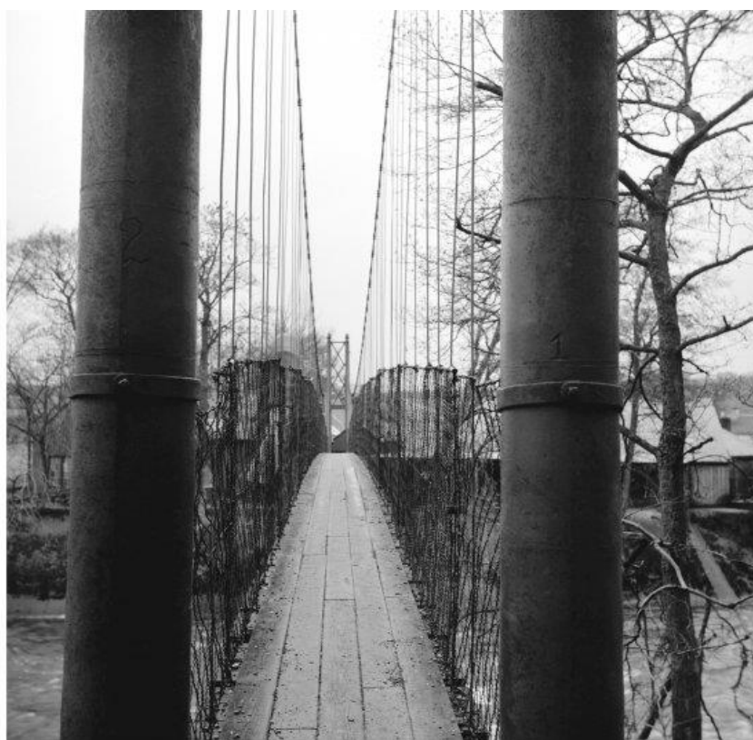
View from south looking towards Milton Hone Works, John R Hume, 1967 [SC589631, 2013, RCAHMS]
