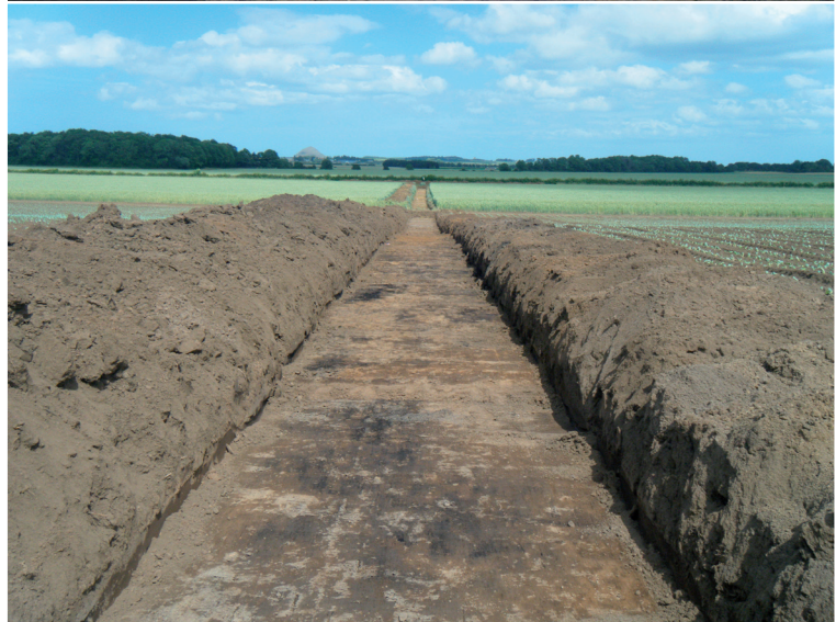
Illus 3 (top) Trench 5, Facing W
