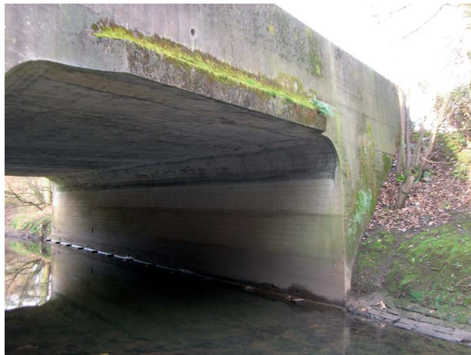
Illus 2 Northern elevation of Auldhouse Bridge: Structure 1
