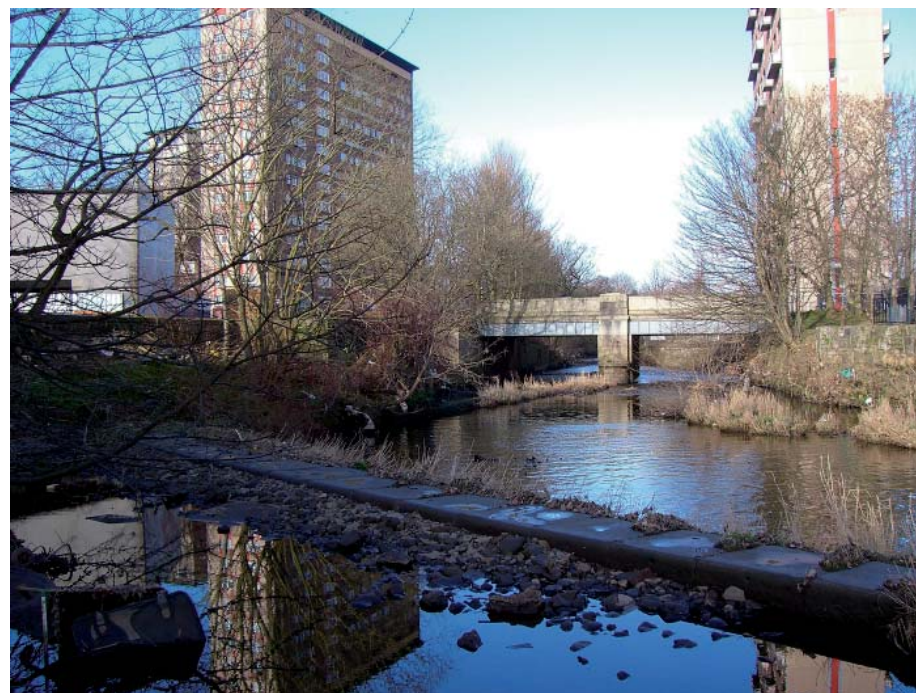
Illus 4 View of current Shawbridge St. Bridge, Str.2
