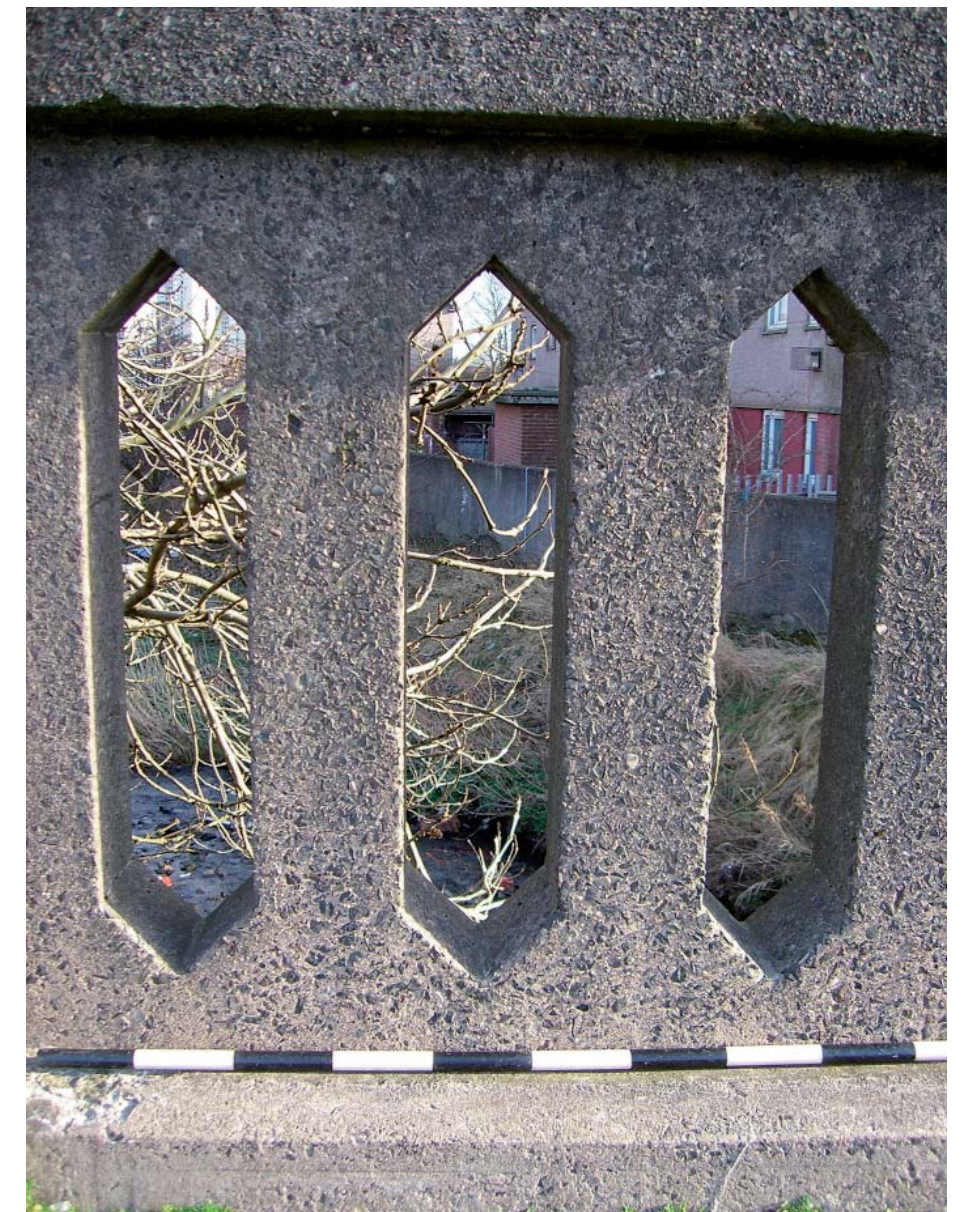
Illus 5 Balustrade detail of Carnwadric Road Bridge, Str. 3
