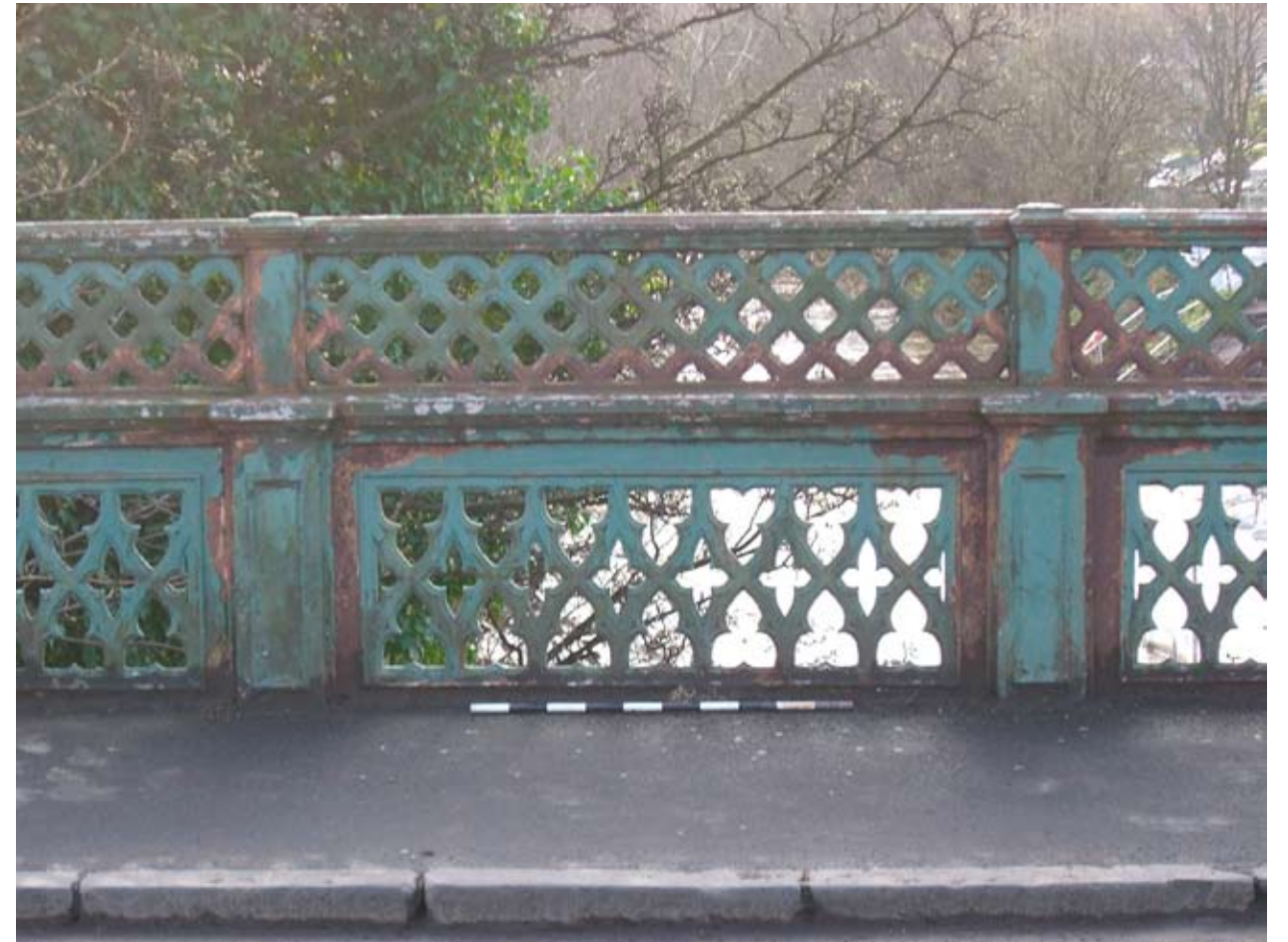
Illus 11 Detail of cast iron work on Devlin Bridge.
