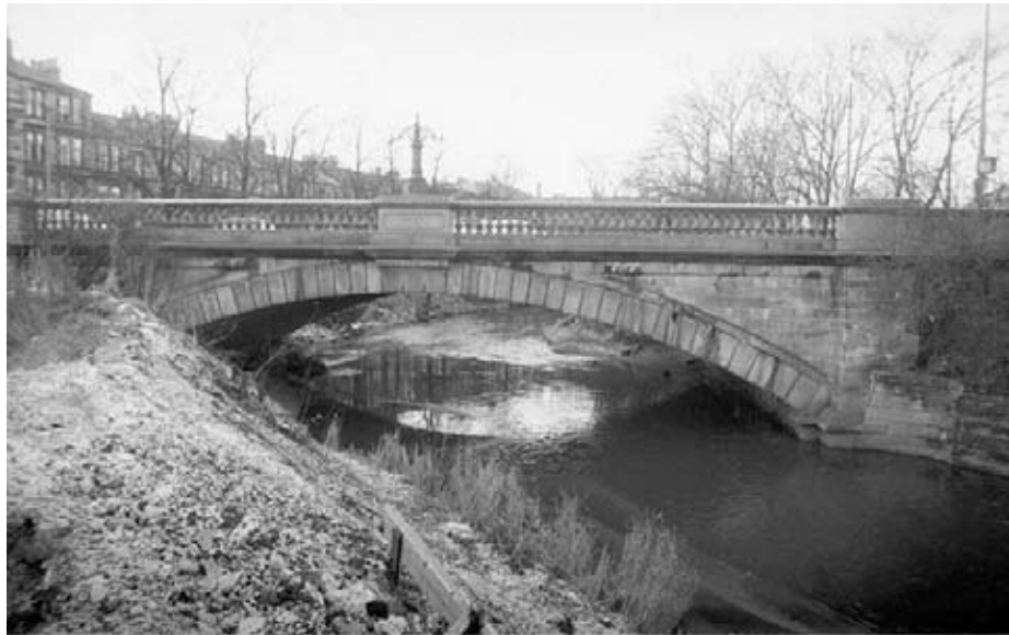
Illus. 4 Holmlea Bridge (© Reproduced by permission of Scran; 000-000-515-196-R)
