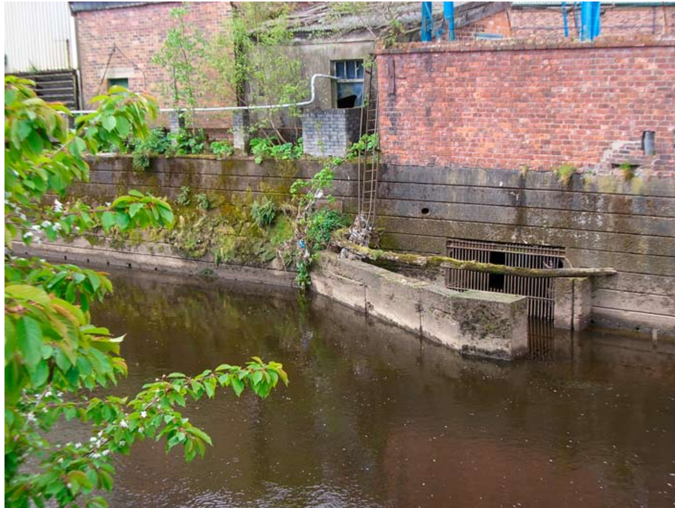
Illus 7 Photo showing detail of Structure 9
