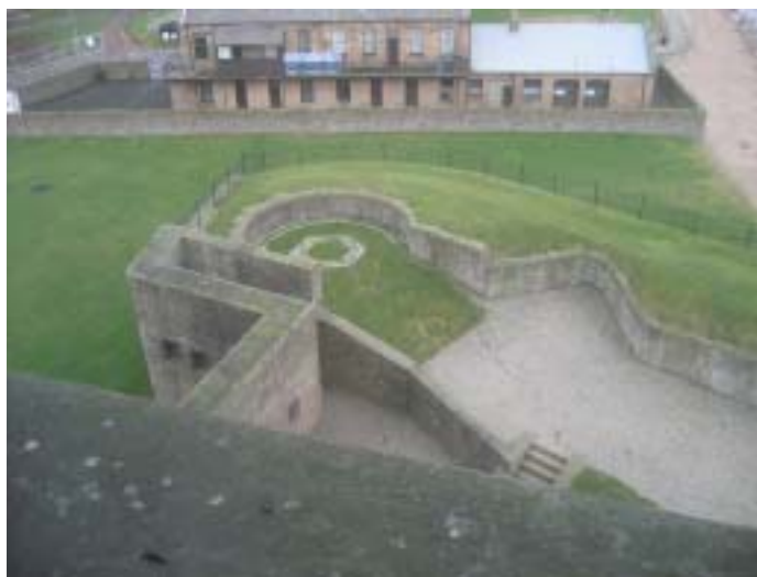
The northeast corner of the battery showing the 68 pounder 'Barbette' emplacement and the 10 inch gun emplacement
