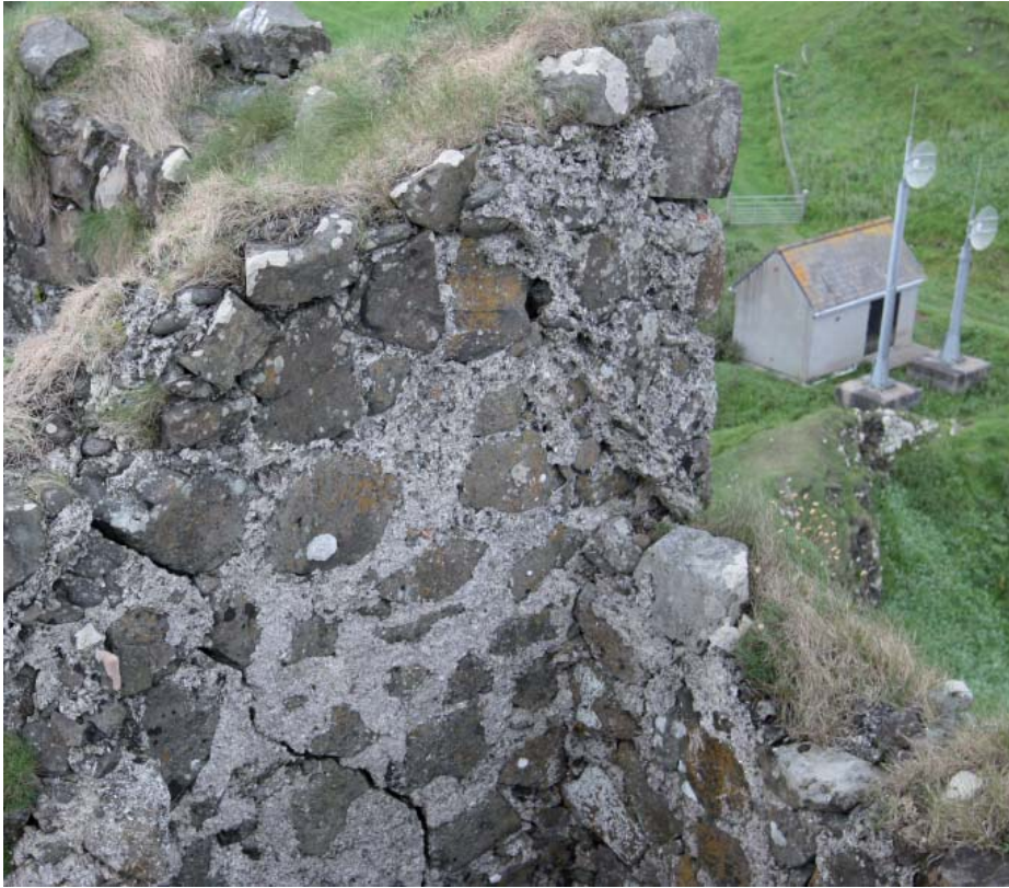
Illus 21 Traces of the pitched roof-line of Chamber D visible on the outer E wall of Chamber C
