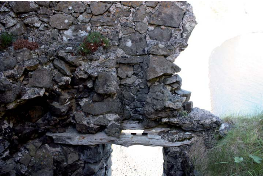
Illus 15 Vertical slot in wall with corresponding slot in wooden lintels above door opening.
