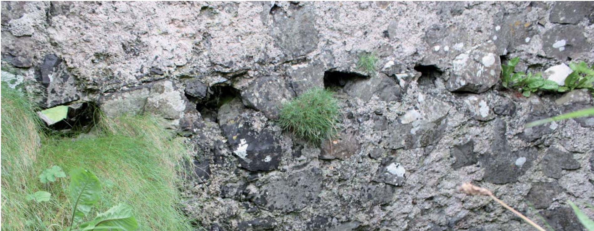
Illus 16 Five slots in the W wall for the floor joists of Chamber C
