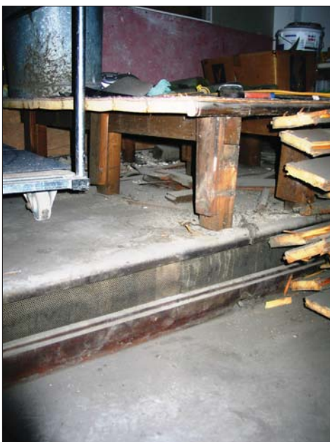
Plate 5: Detail of the construction of the later raked floor overlying earlier floor. Looking south-west.
