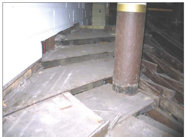
Plate 4: Detail of earlier raked floor leading to stairwell. Looking east.
