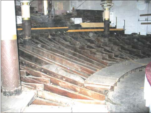
Plate 7 & 8: Timber floor beams after the removal of the early raked floor. Right - Looking south. Left - Looking west.
