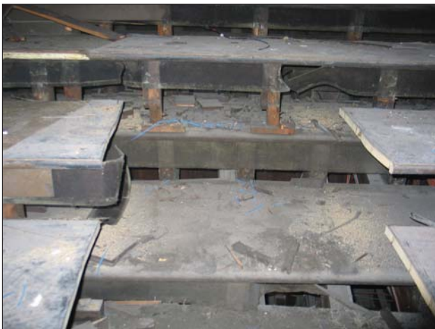
Plate 3: Detail of later raked floor with earlier floor seen below. Looking south-east.
