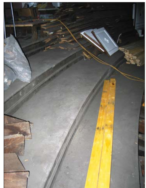
Plate 5: Detail of the construction of the later raked floor overlying earlier floor. Looking south-west.
