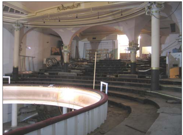
Plate 2: General view of later raked floor. Looking east.
