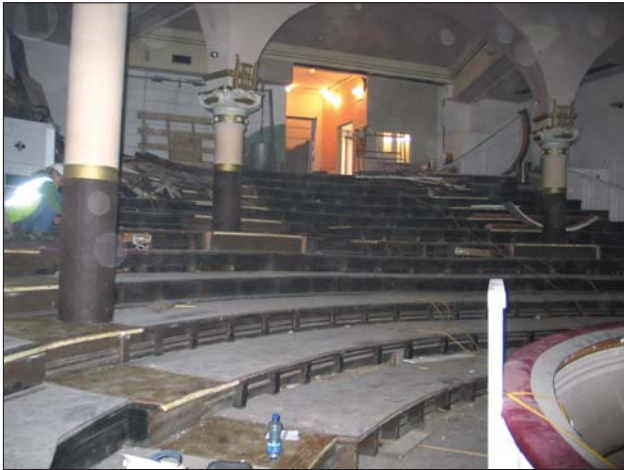
Plate 1: General view of later raked floor. Looking south.
