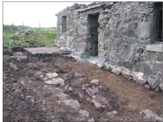
18. General view of area south of cottage
