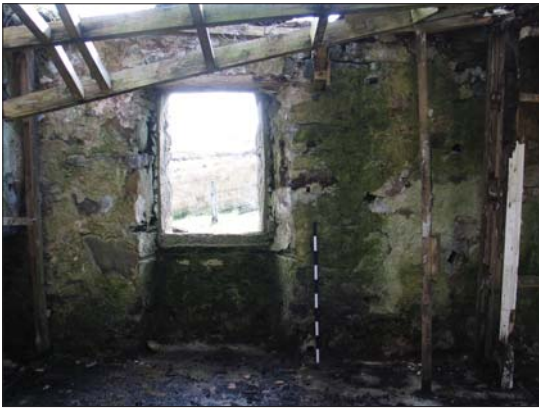
33. E window in S wall from N
