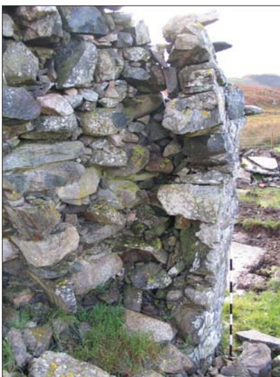
29. Detail of wall construction at SW corner from NW
