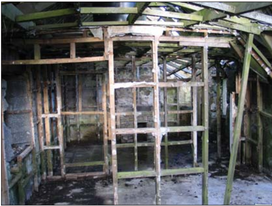
31. General interior shot from W
