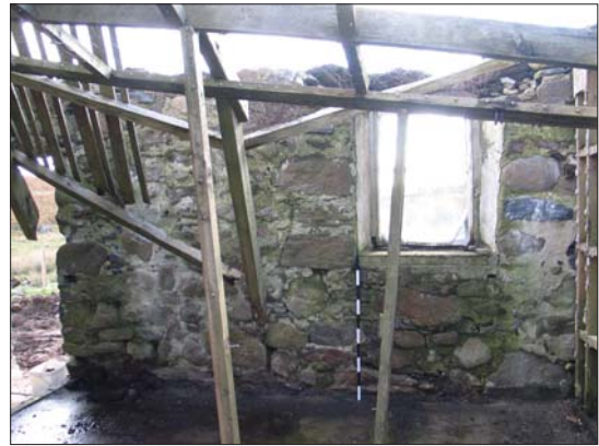
34. W window and doorway in south wall from N
