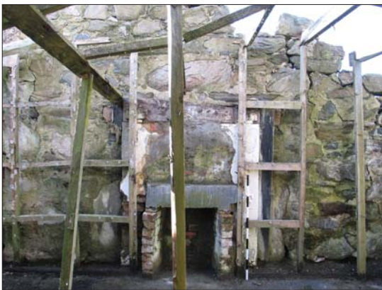
35. W internal wall from E
