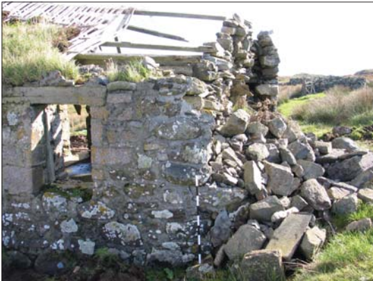
27. Detail of NW corner from NW
