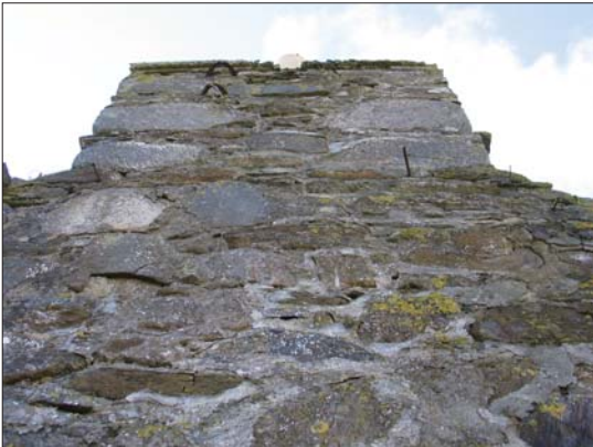
25. Detail of chimney cap and metal fittings
