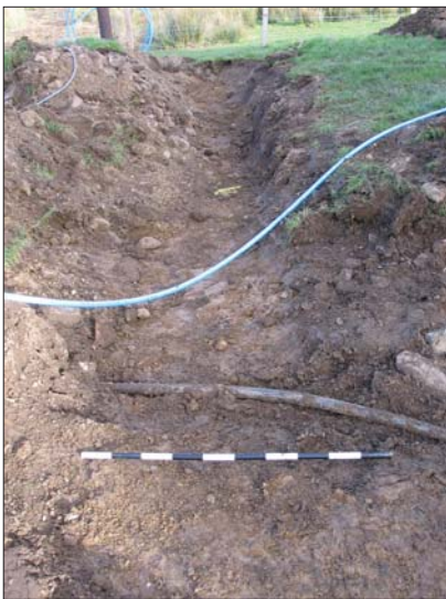
11. Service tracks at E of cottage from N
