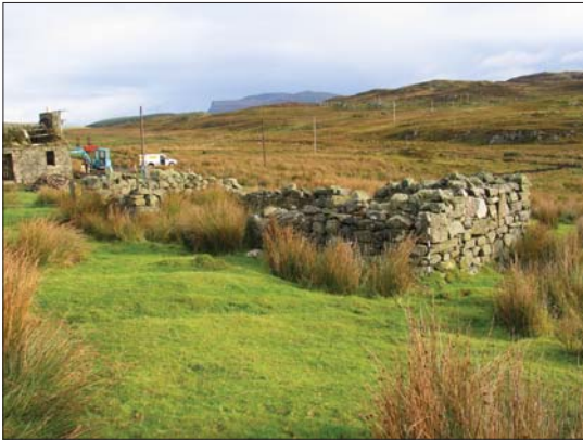
3 Township Building B from SW
