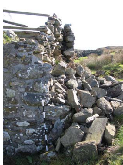
28. Detail of W gable from N
