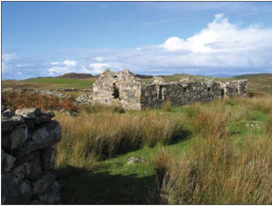
7. Township Building K from SE
