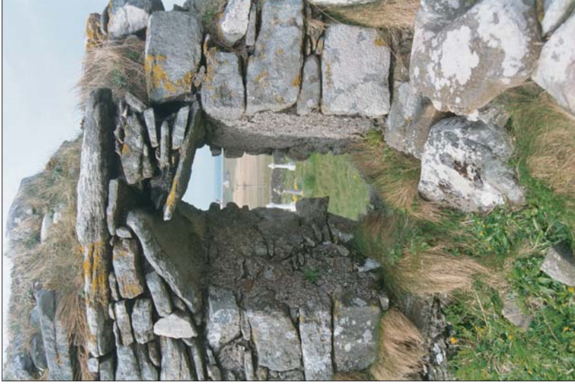
Plate 11: Building No.3, North Wall interior; detail of window, facing N.
