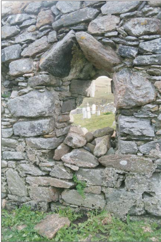
Plate 5: Building No.3, South Wall interior; detail of west window, facing S.
