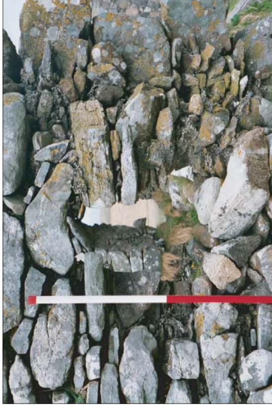
Plate 4: Building No.3, South Wall exterior; detail of east window, facing N.
