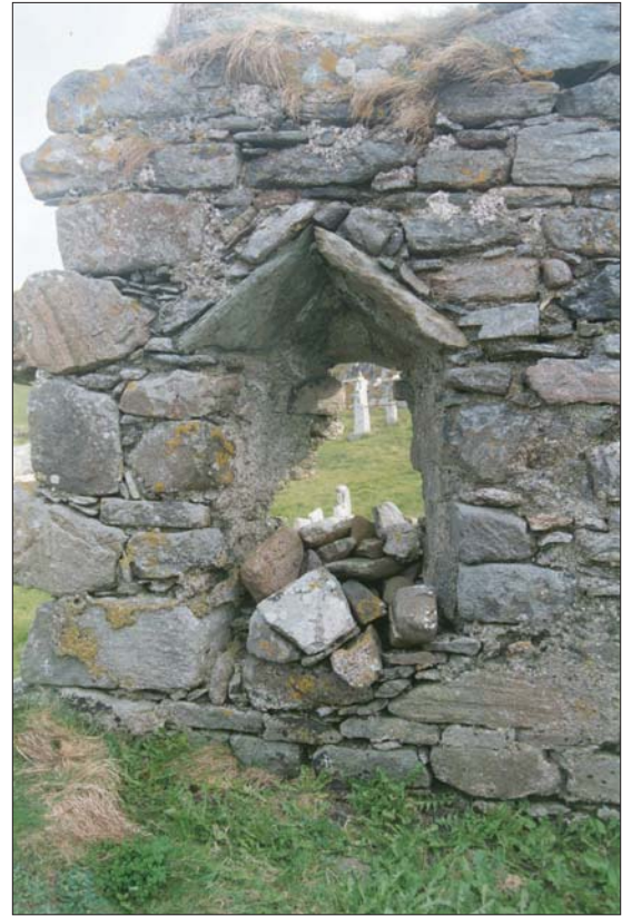
Plate 6: Building No.3, South Wall interior; detail of east window, facing S.
