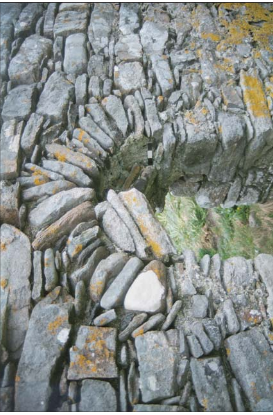
Plate 13: Building No.3, North Wall exterior; detail of entrance, facing SW.
