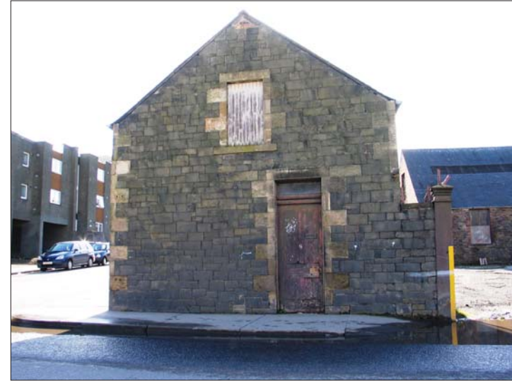
Plate 10 - Building 2, view from N
