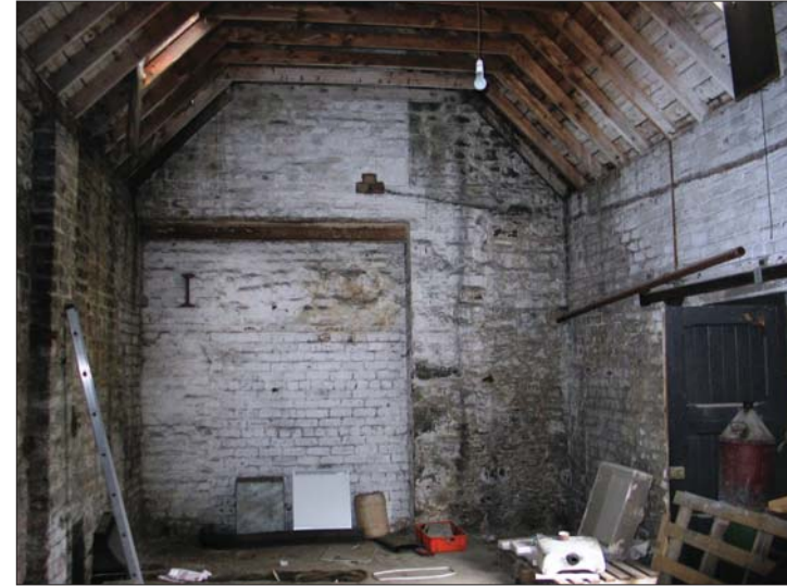
Plate 38 - Building 5, interior, detail of S wall (position of boiler)
