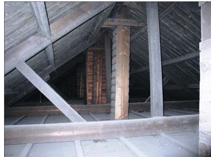
Plate 24 - Building 3, roof space (south), showing ridge vents
