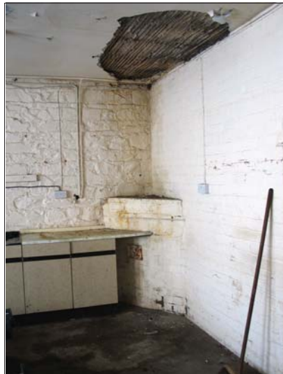
Plate 55 - Building 8, interior, ground floor
