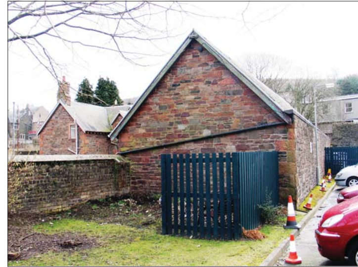
Plate 54 - Buildings 8-10, view from NW
