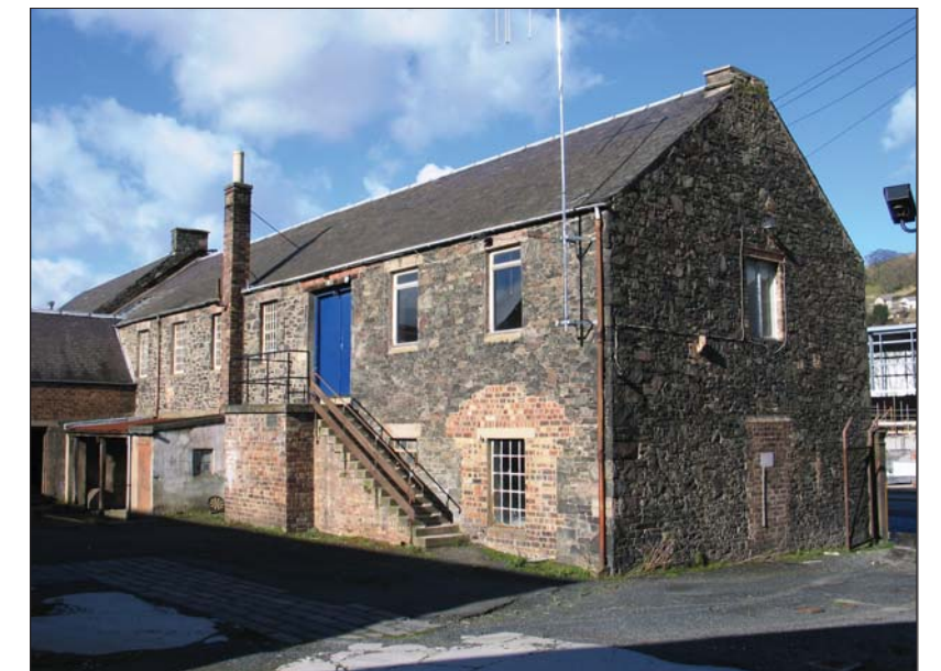
Building 4, view from SE
