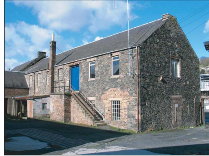
Plate 26 - Building 4, view from SE
