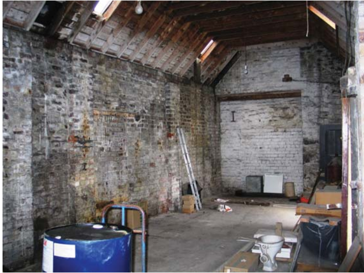
Plate 37 - Building 5, interior, view from S
