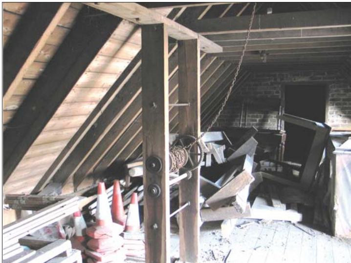
Plate 64 - Building 9, attic floor and hoist
