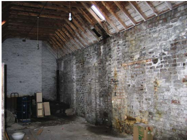
Plate 39 - Building 5, interior, E wall
