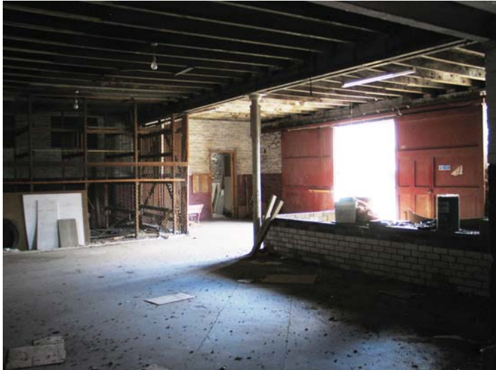
Plate 17 - Building 3, interior (north range)
