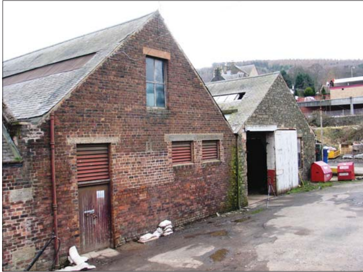
Plate 13 - Building 3, view from NW
