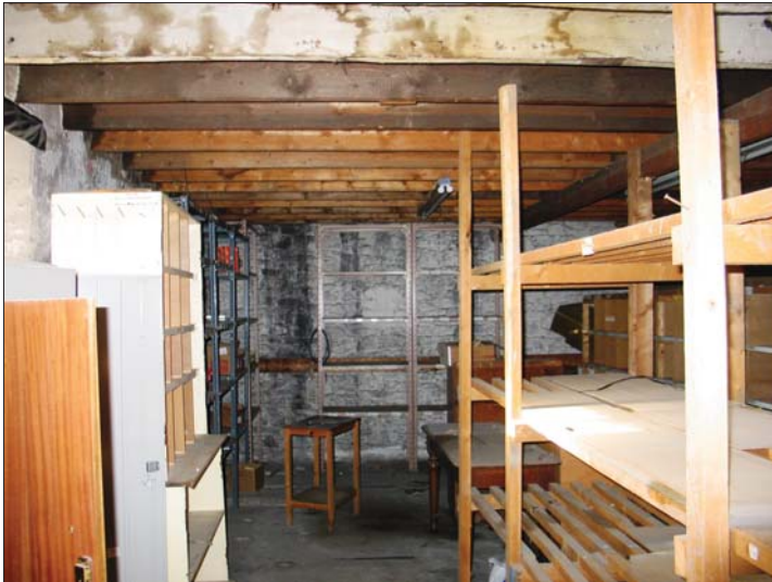
Plate 31 - Building 4, first floor interior (NW)
