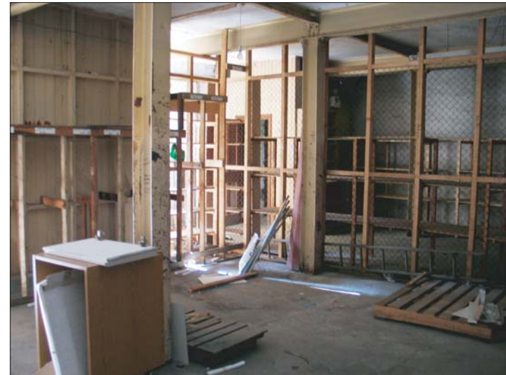
Plate 28 - Building 4, ground floor interior
