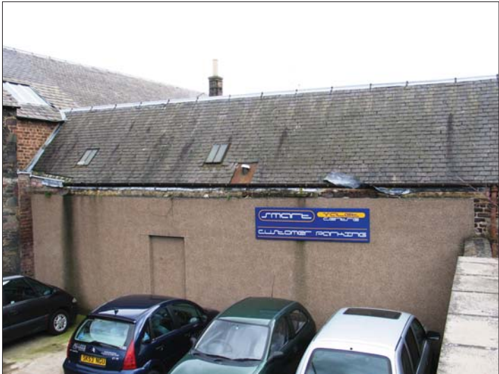
Plate 35 - Building 5, view from SW
