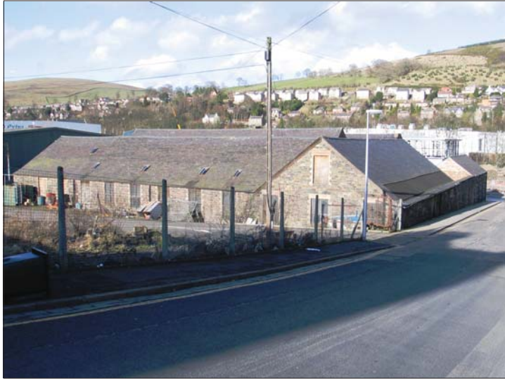
Plate 5 - Buildings 1 and 3, view from SE
