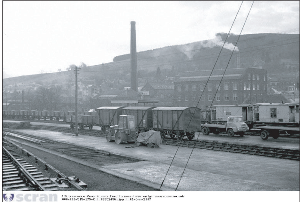
This photograph shows Waverley Mill looking across the river and railway. The tall chimney of the incinerator can be seen in the background behind the tall 1866 mill, still in use. Taken by John Hume c.1969
