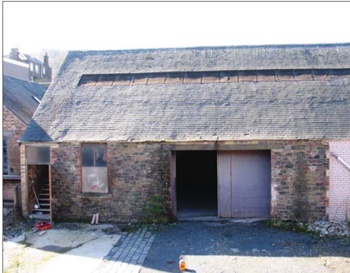
Plate 15 - Building 3, view from N
