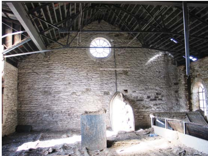
Plate 47 - Building 6, interior, first floor main room
