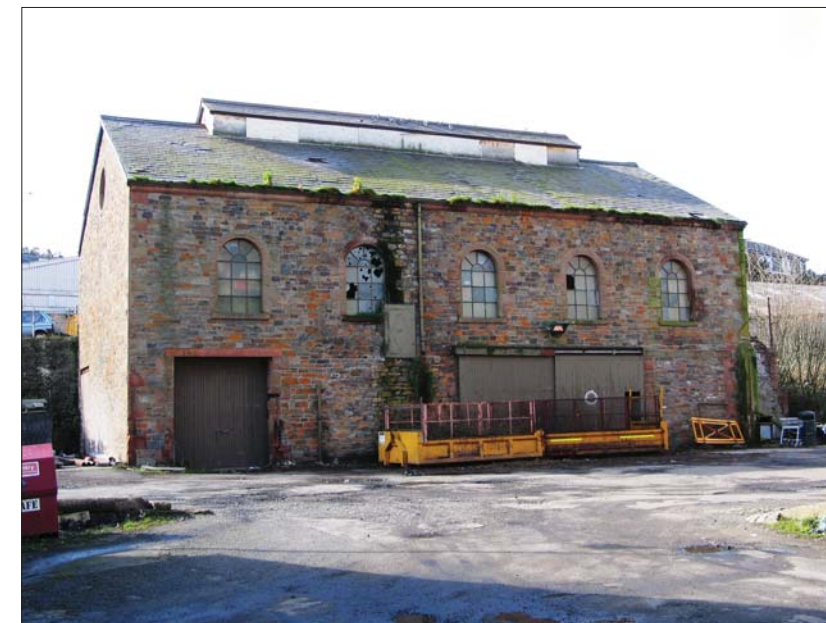
Building 6, view from NNE
