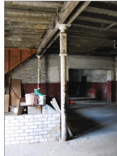
Plate 16 - Building 3, ceiling and columns
