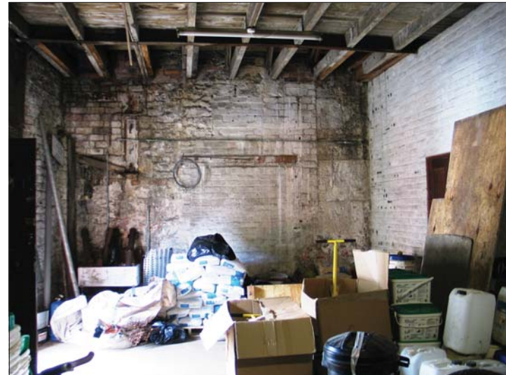
Plate 20 - Building 3, interior showing blocked bearing boxes
