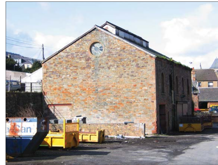
Building 6, view from E
