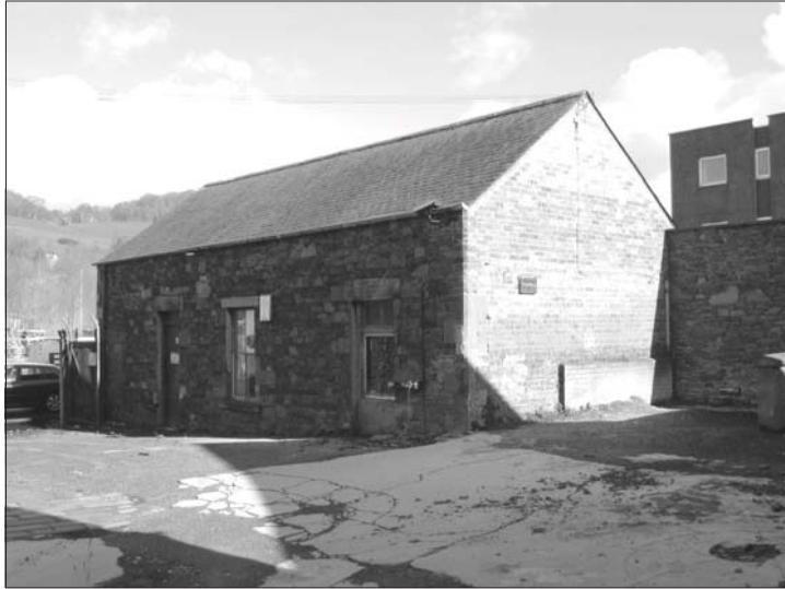
Plate 9 - Building 2, view from SW
