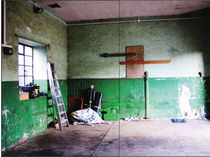
Plate 62 - Building 9, interior of stable
