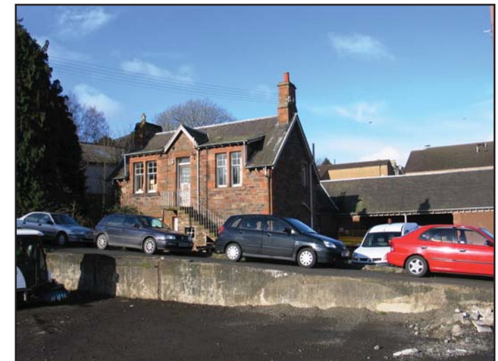
Building 8, view from NE
