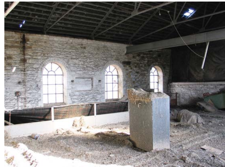
Plate 48 - Building 6, interior, first floor main room
