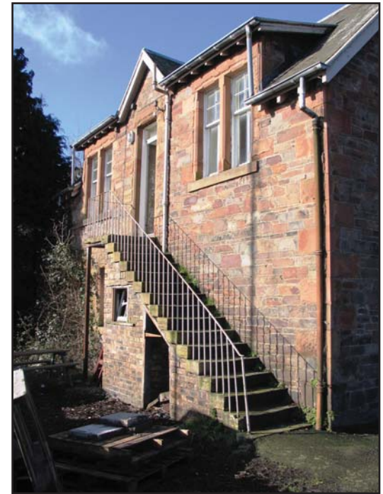
Building 8, view from NE
