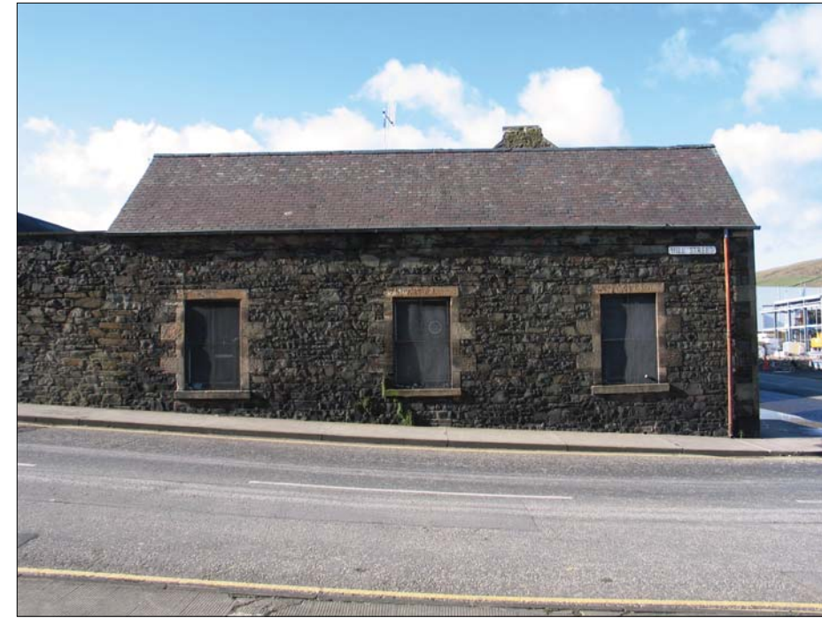
Building 2, view from E
