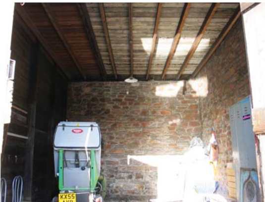
Plate 68 - Building 10, interior of cart shed
