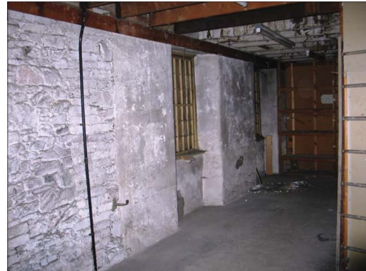
Plate 32 - Building 4, first floor interior (NW)
