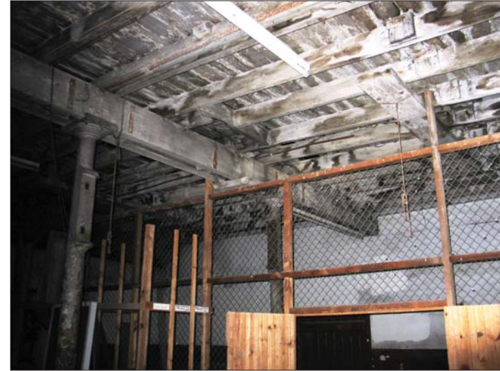
Plate 6 - Building 1, ceiling and column
