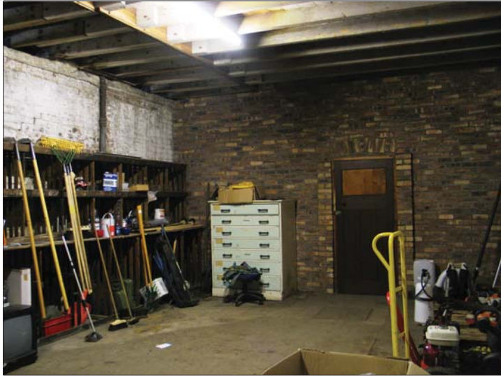
Plate 21 - Building 3, brick partition and earlier columns
