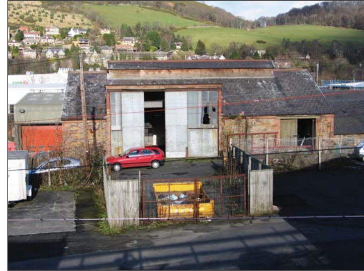
Plate 42 - Building 6, view from the S
