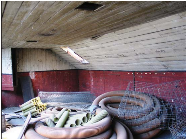
Plate 23 - Building 3, loft (south)
