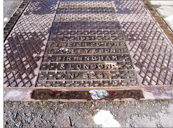
Plate 2 - Weigh Bridge detail
