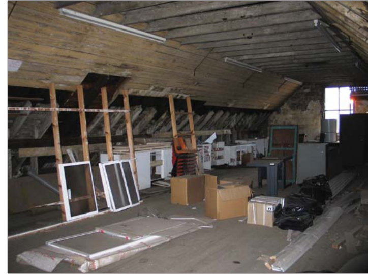
Plate 22 - Building 3, loft (north)
