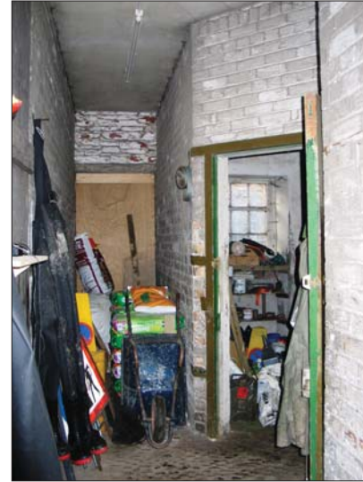
Plate 67 - Building 9, hall at W
