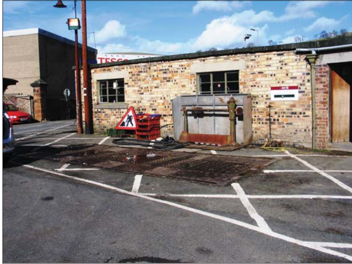
Plate 1 - Weigh Bridge, view from SE
