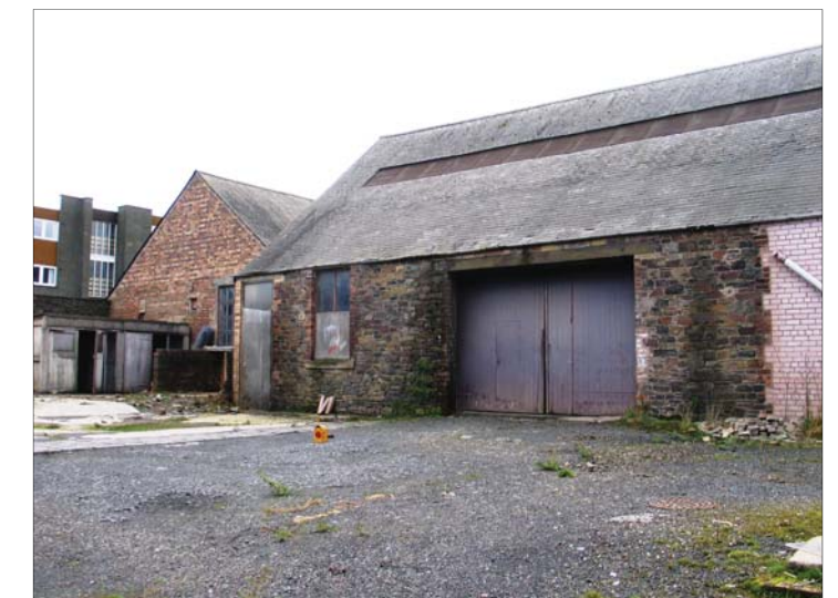
Buildings 1 and 3, view from NW
