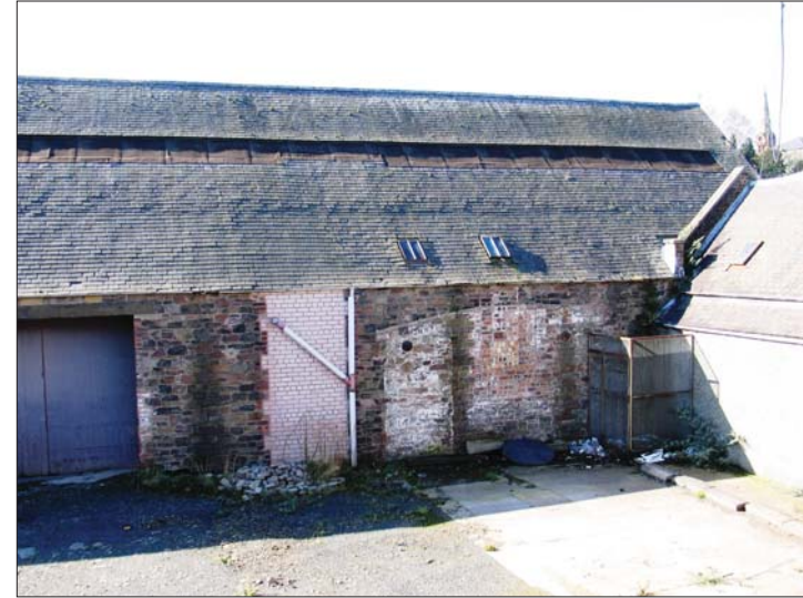
Plate 14 - Building 3, view from N
