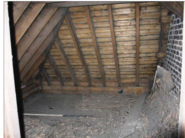
Plate 65 - Building 9, attic floor, room at SW
