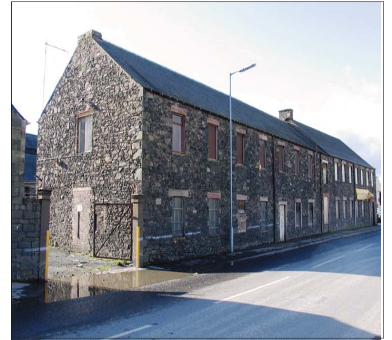
Building 4, view from NE
