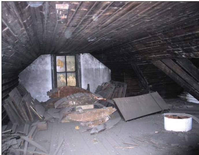
Plate 7 - Building 1, north loft
