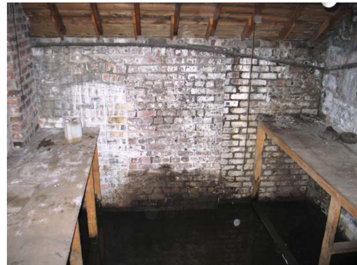
Plate 40 - Building 5, interior, S room
