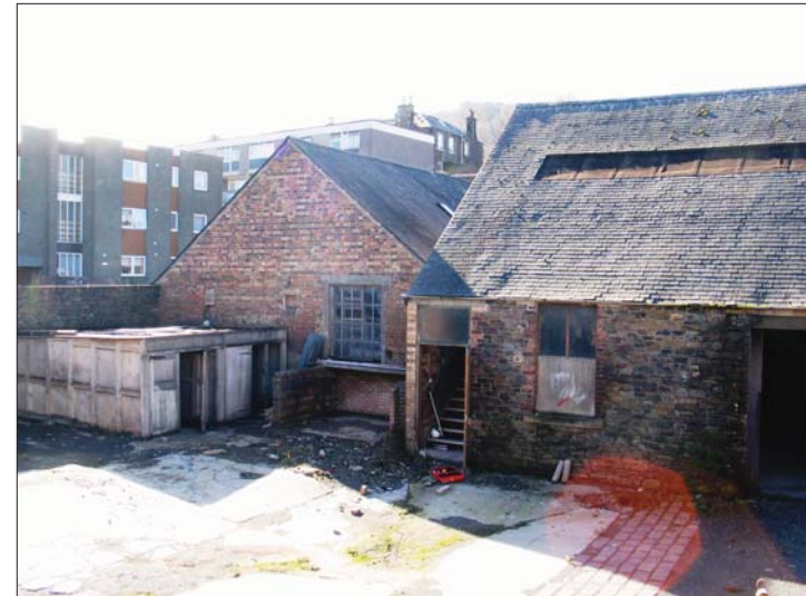
Plate 4 - Buildings 1 and 3, view from NW
