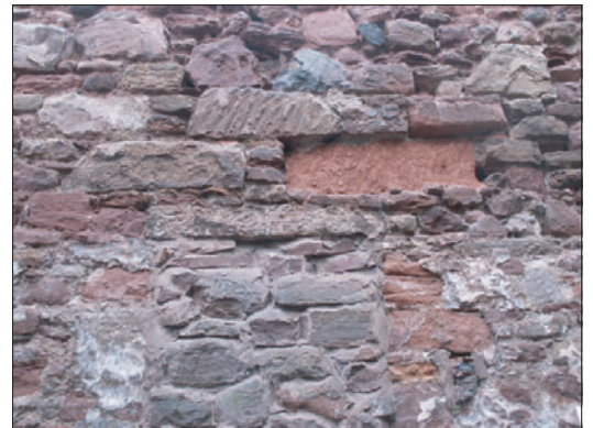
Plate 3. (below) The north wall - Detail of the blocked doorway head and lintel (15). Pantiles are visible just above the lintel on the left.
