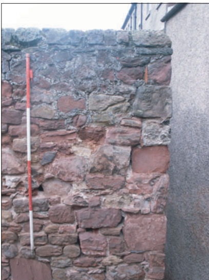
Plate 5. (left) The north wall - Detail of the upper coursing and quoins (19).
