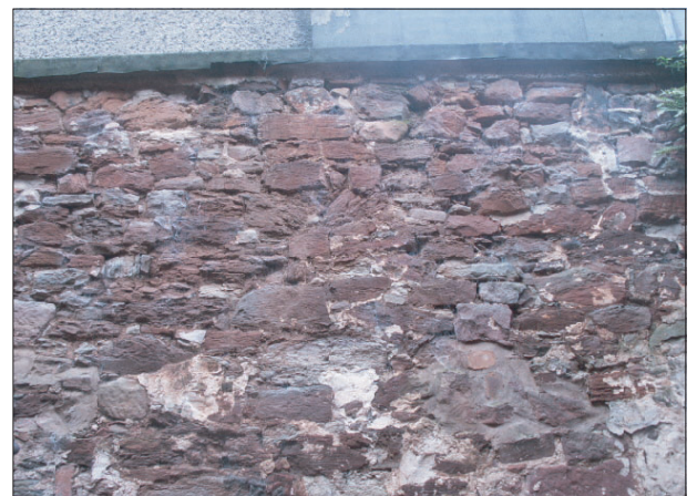
Plate 6. (below) The south wall - Line of possible gable (3) and blocked opening (2).
