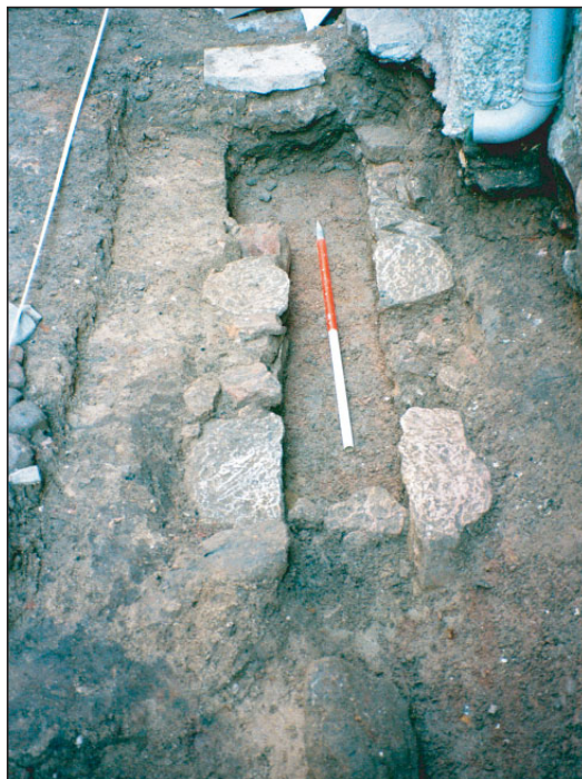
Plate 6 - Stone culvert 425: from the west
