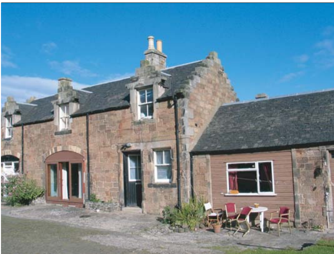
Plate 3: Building A, southeast corner
