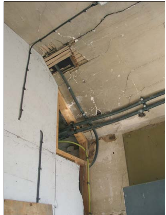
Plate 12: Hipped ceiling in Building B
