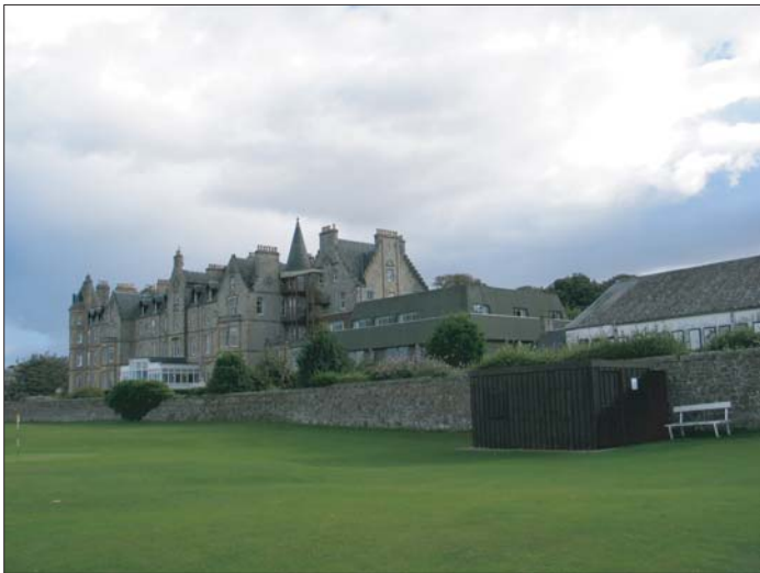
Plate 13: Buildings D, E and Marine Hotel from north-west
