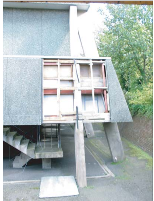
Plate 14: Building D, south-west corner looking east
