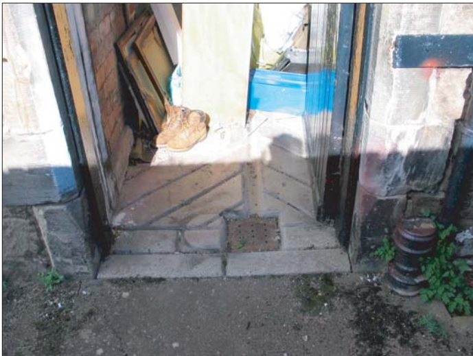
Plate 11: Drains in floor of Building B
