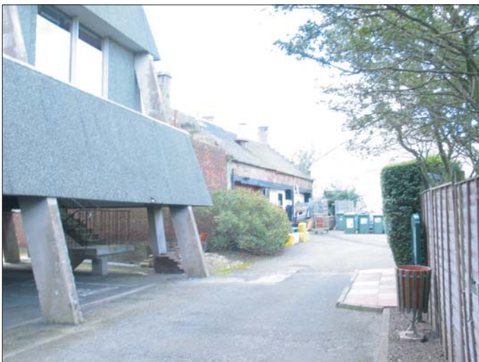
Plate 15: Building D, north-west corner looking west
