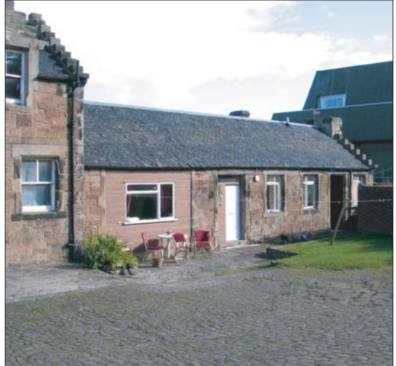
Plate 2: Building B, south elevation
