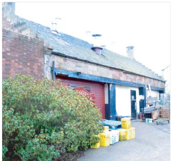
Plate 4: Building C, north elevation
