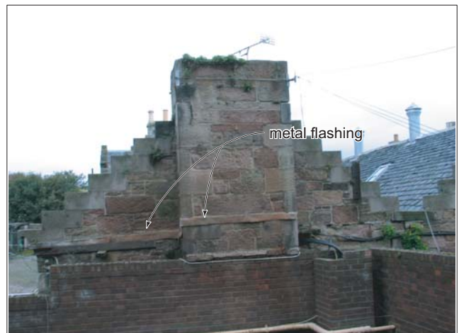
Plate 8: Building C, chimneystack and flashing
