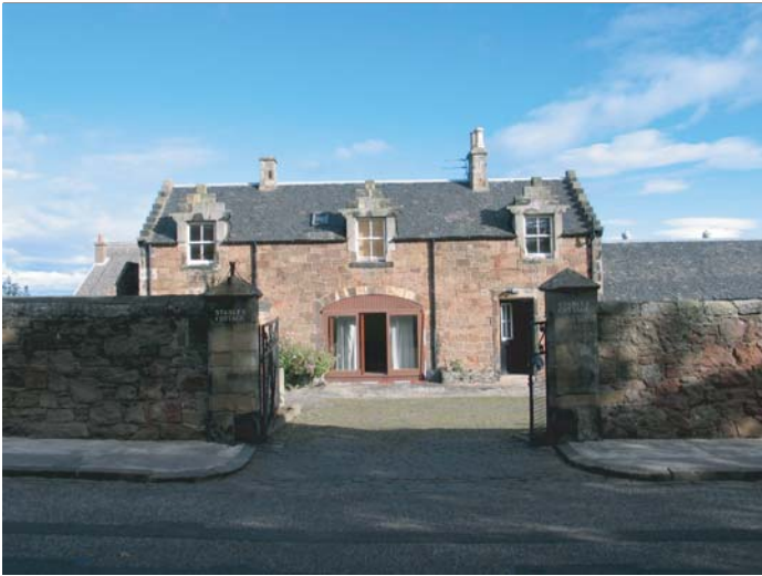
Plate 1: Building A, south elevation
