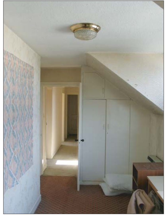
Plate 10: Building A, first floor hallway facing west
