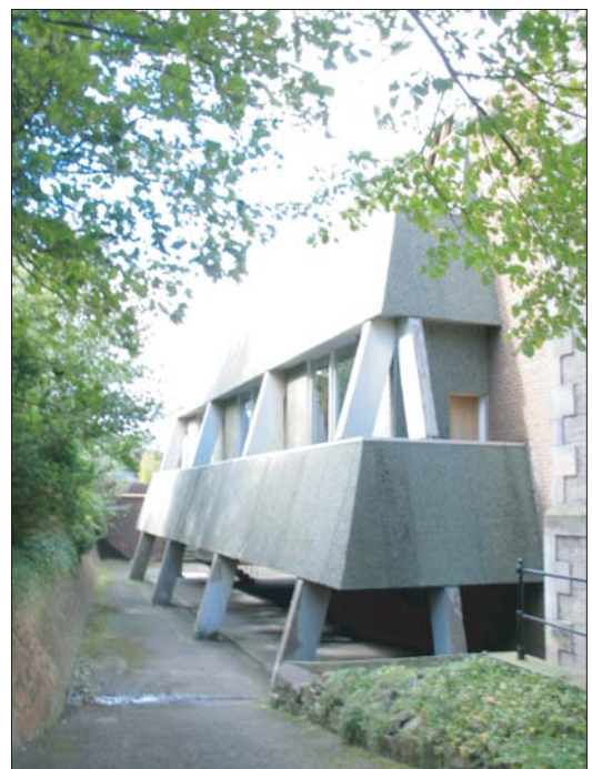
Plate 16: Building D, south-east corner looking west
