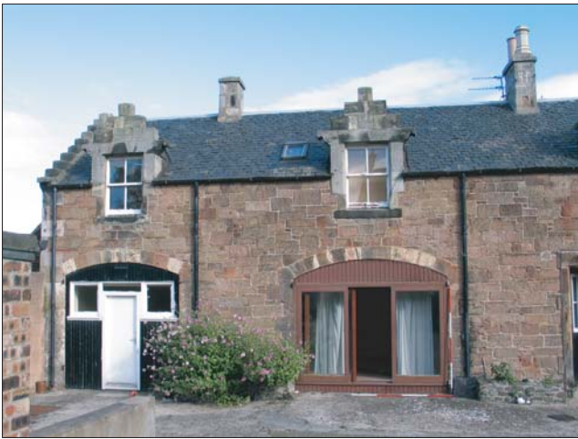
Plate 5: Blocked carriage arches in Building A
