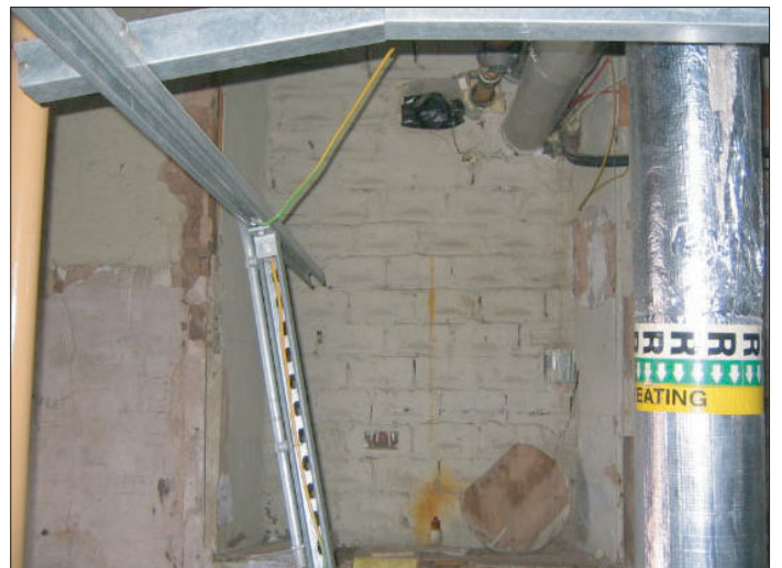
Plate 4: Blocked window in Building C, facing east
