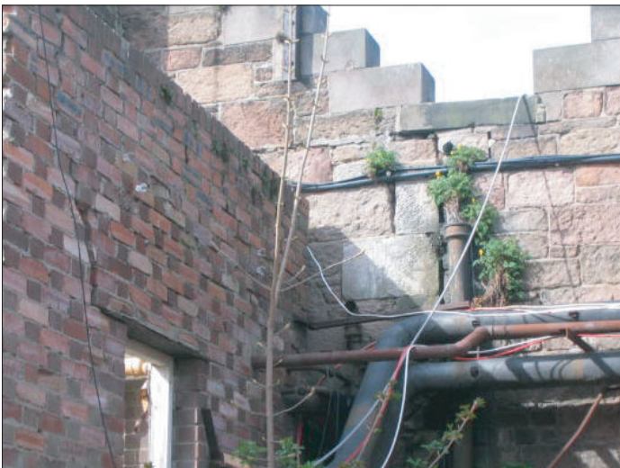
Plate 3: Eastern end of Buildings B & C facing west
