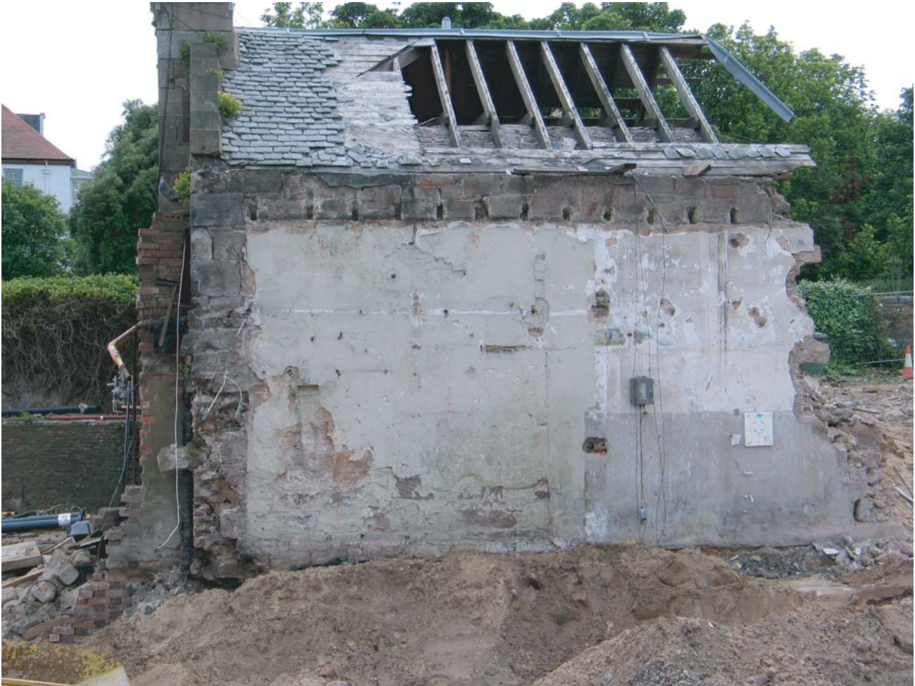
Plate 1: Exterior of Building B, with Building C removed, facing S.
