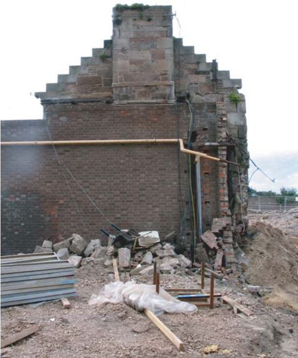
Plate 2: Exterior of Building B, facing W, showing brick skin below chimney stack.
