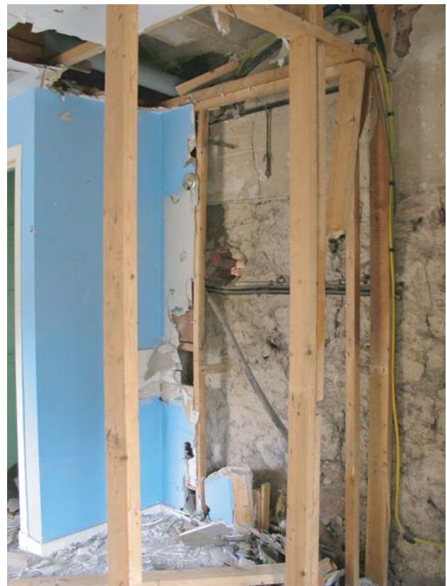
Plate 3: Building B, east interior wall-face with plasterboard removed.
