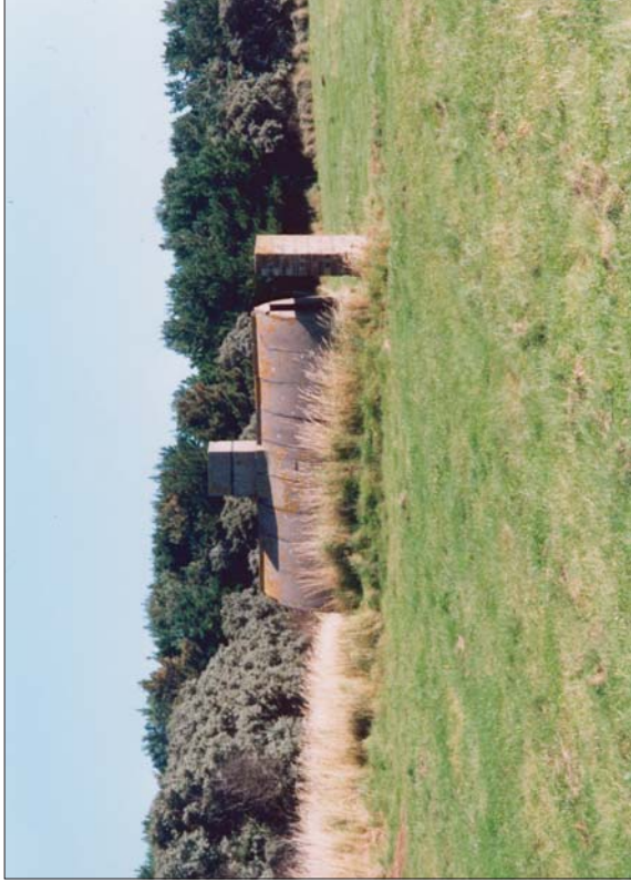
Plate 31 - Air raid shelter from the west
