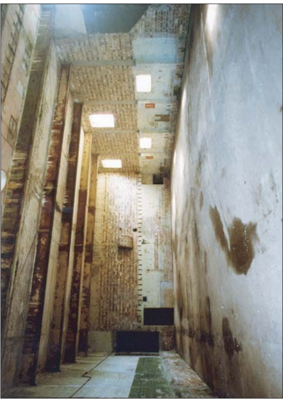
Plate 14 - Southern wall of the operations room
