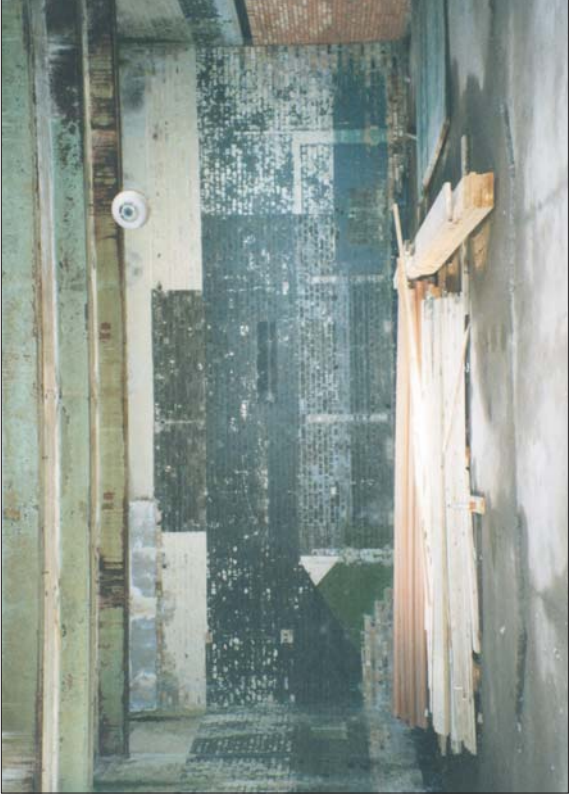
Plate 13 - Northern wall of the operations room (TJ)
