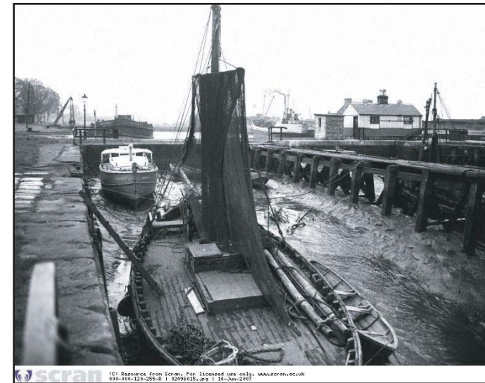
Plate 4: The harbour and dock beyond - looking east.
