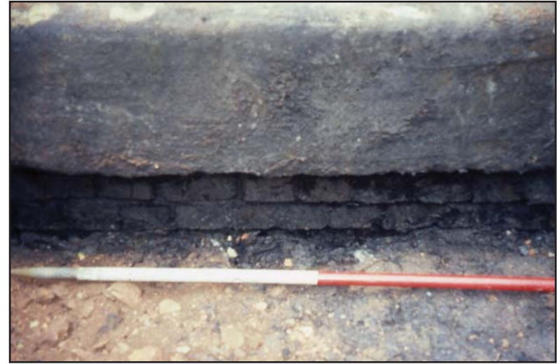
Plate 8: Trench 1 - Detail of brickwork on quay wall.
