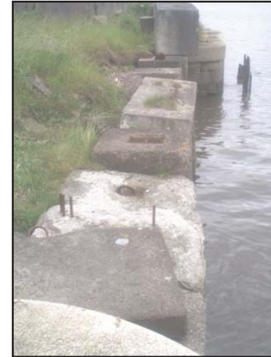
Plate 5a: Blocked 1880's gate - looking south.
