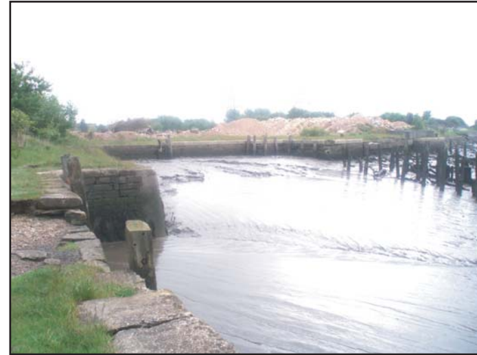
Plate 2: Entrance to wet dock - looking east.
