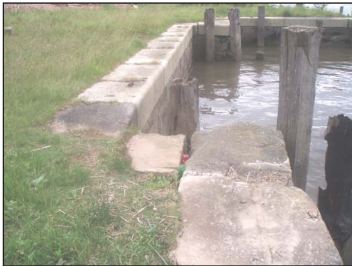
Plate 5b: Blocked 1860's gate. Note the difference in the cope stones - looking south (1860's in the foreground & 1880's beyond).
