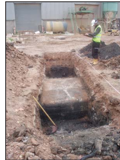
Plate 6: Working shot of excavation of Trench 2 - looking north.
