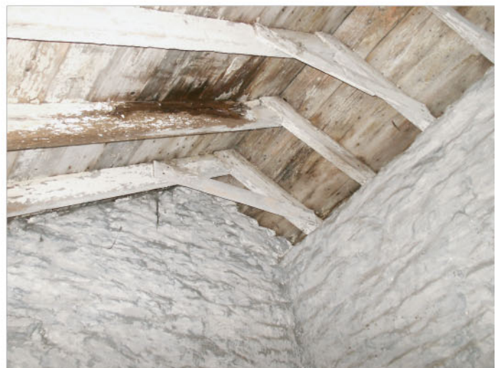
Plate 18 : Building D, Kennel 4. Interior. Detail of twin-pitch roof construction.
