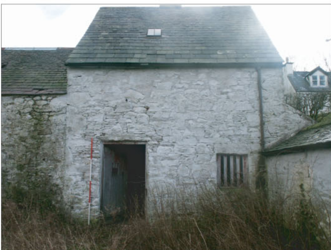
Plate 5 : Building A. North exterior elevation showing doorway, original door and window. Building D is shown part butted on the right.
