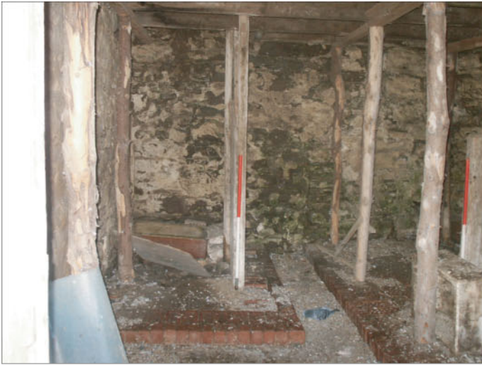
Plate 7 : Building A, Room 1. South interior elevation showing cobble and brick floor and blocked opening. Note the rough timbers, which are recent additions, supporting the joists of the upper floor.
