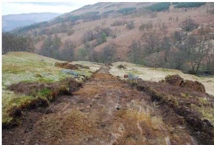
View to NNE along pipe route for Intake 5 as excavated.
