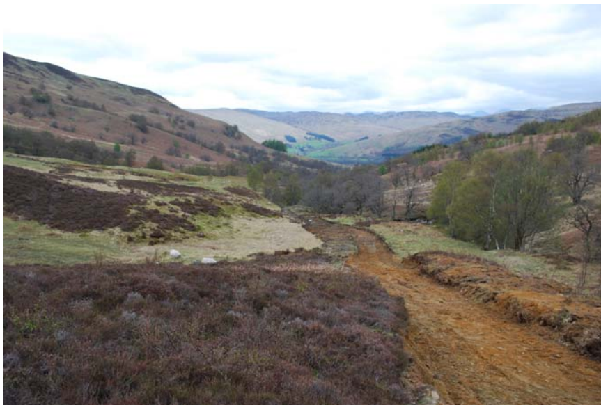
General view to the N of upgraded track Site 4 as excavated.
