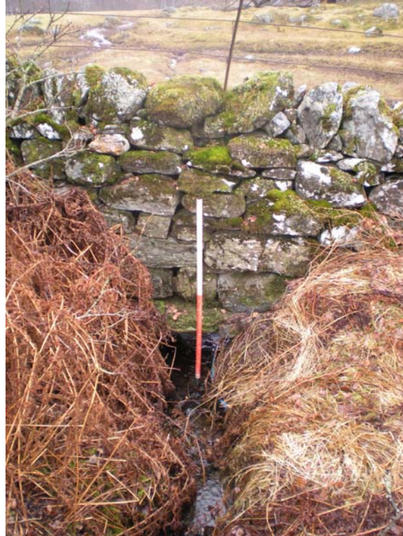
Culvert 18A in wall Site 18, view to the NNW.
