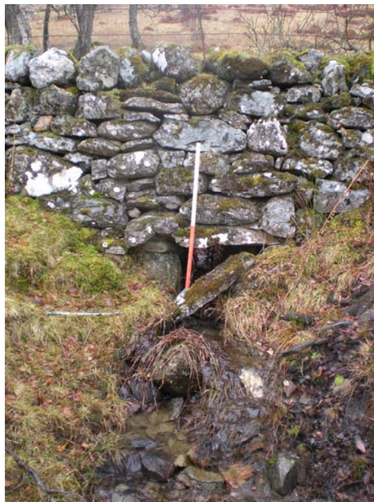
Culvert 18A in wall Site 18, view to the SSE.
