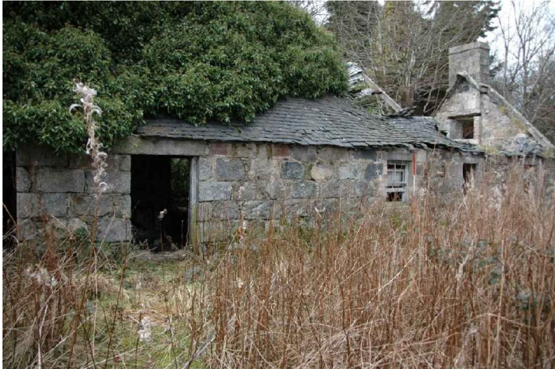
Illus 103 Gardener's Cottage from E, workshop door on LHS
