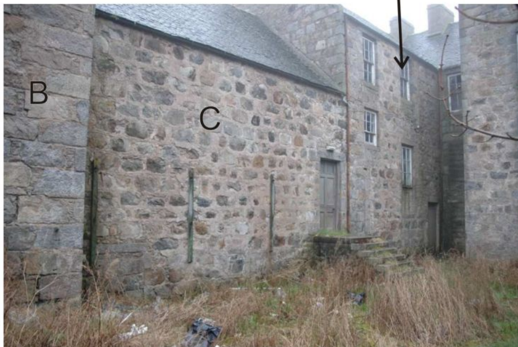
Illus 29 E wall of Old Chapel and Menzies Apartments.
