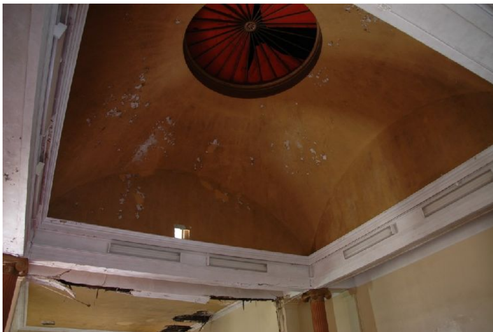
Illus 34 Oculus ceiling from below, capitals of pillars to LHS and centre base
