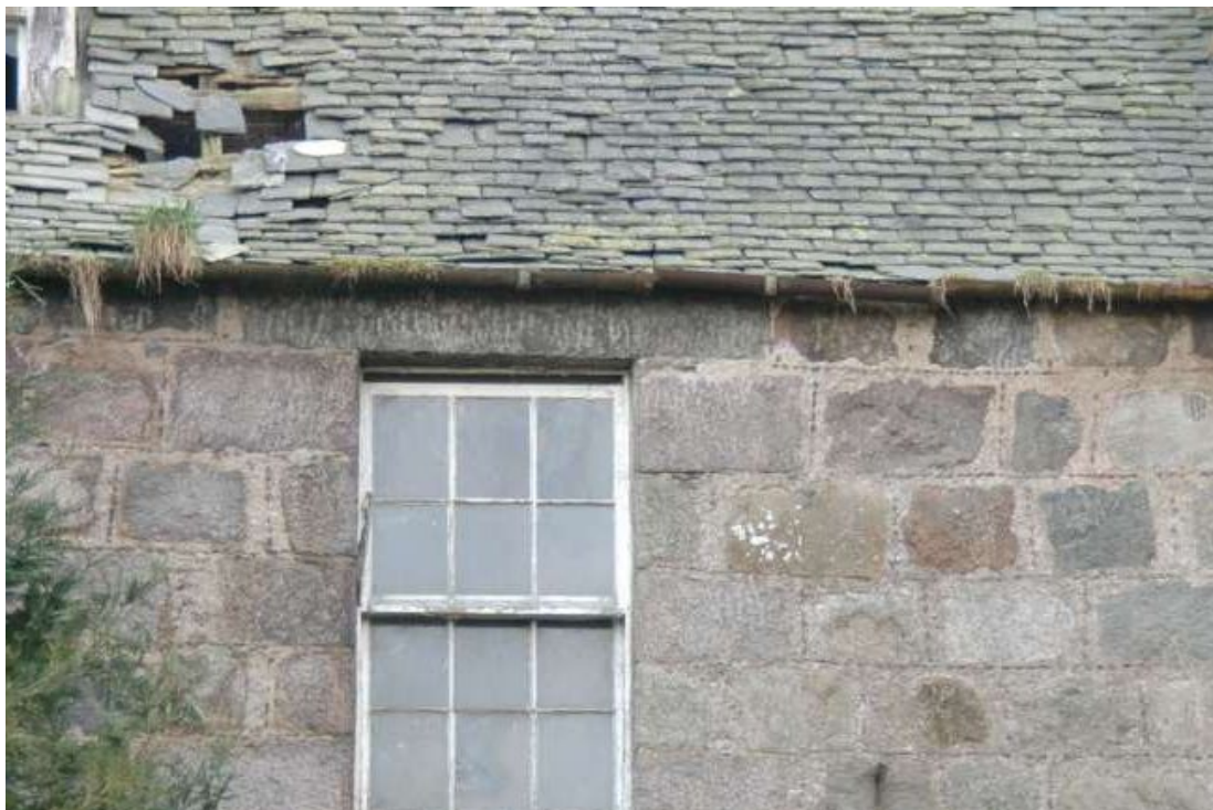
Illus 49 Detail of stone work of N front of Menzies House showing pinnings
