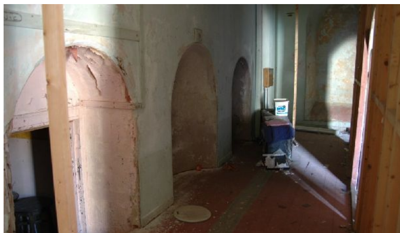
Illus 36 Interior of S end wall with central blind alcove flanked by doors to vestries partially blocked by stage
