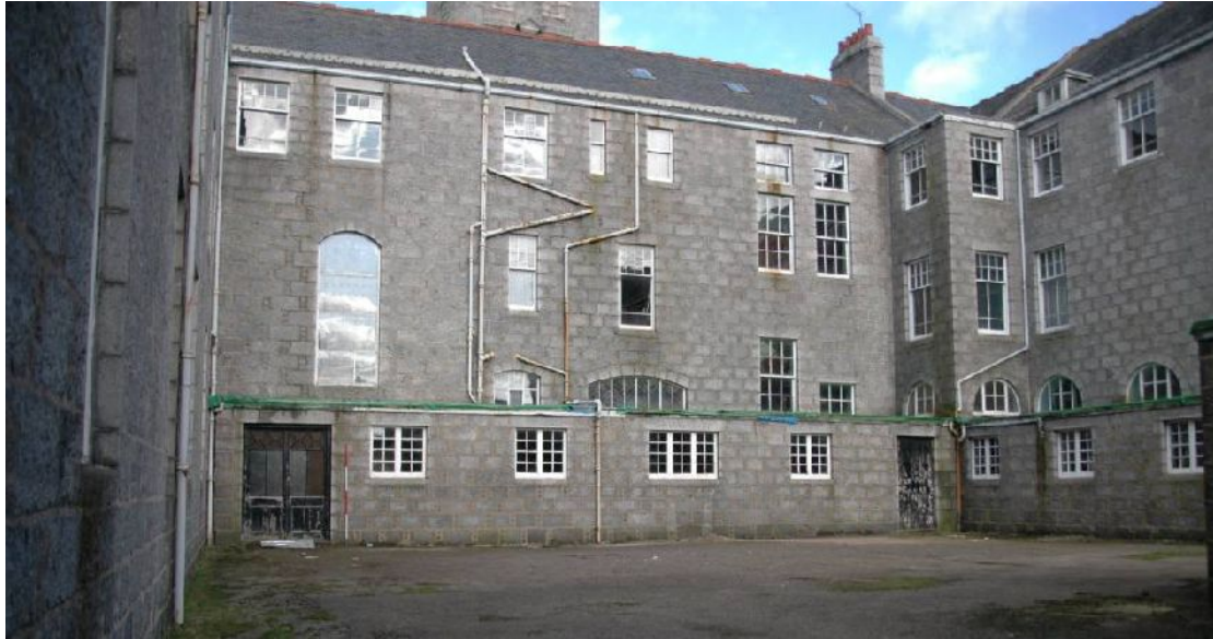
Illus 67 Internal courtyard looking N to the back of the front block. The window above main stair visible on LHS. Covered single storey passage around perimeter
