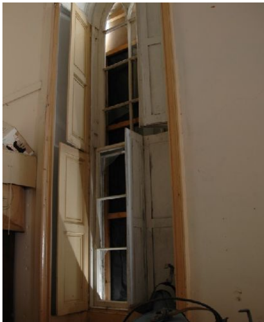
Illus 33 Internal shutters window W4 of W wall
