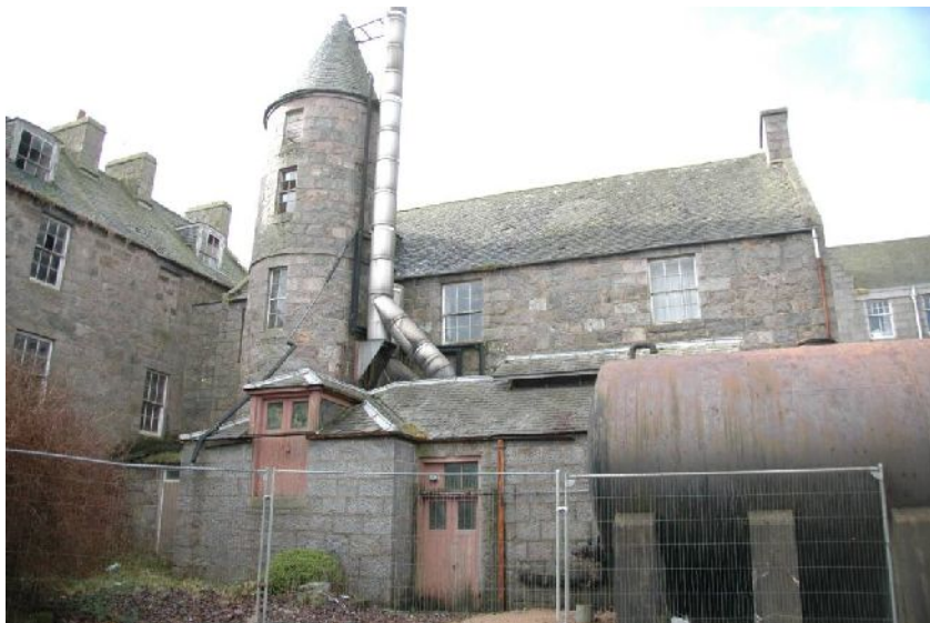
Illus 60 1854 extension with 1925 additions from E
