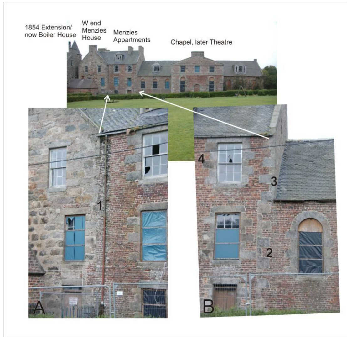
Illus 26 Building sequence on the W façade of Old College
