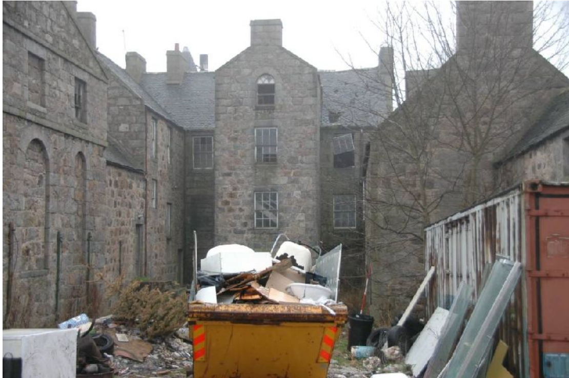
Illus 48 The back (S) side of the surviving W part of the Menzies House, flanked by the Old Chapel and Menzies Apartment (LHS) and the Laundry (RHS)
