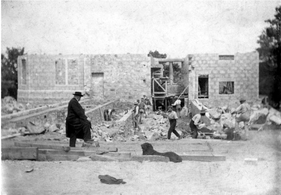
Illus 62 Building work in progress c. 1898 (Blairs Museum 122) Note at this stage the then W end of N wing had a bay window, later replaced at the W end of 1906 block
