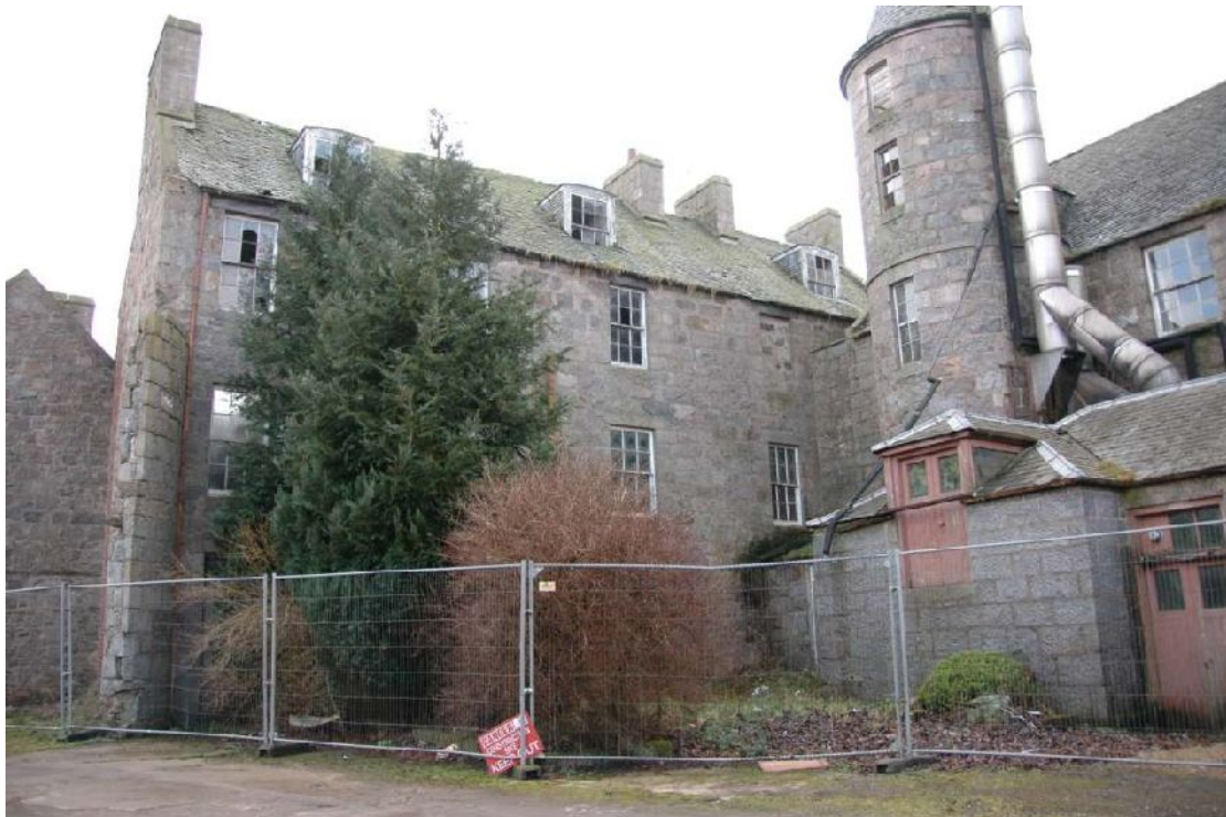
Illus 47 The surviving W wing of the Menzies House. The truncated round tower is visible to the LHS. The 1854 extension (now the Boiler House) with 1925 lower extension to RHS.
