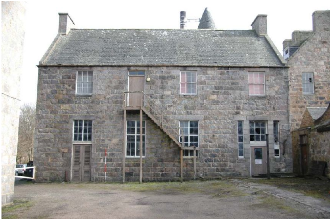
Illus 58 Boiler House/ 1854 extension from W
